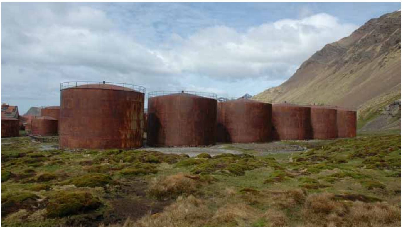
34.3 Tanks 52-57, west side of Tanks looking southeast
