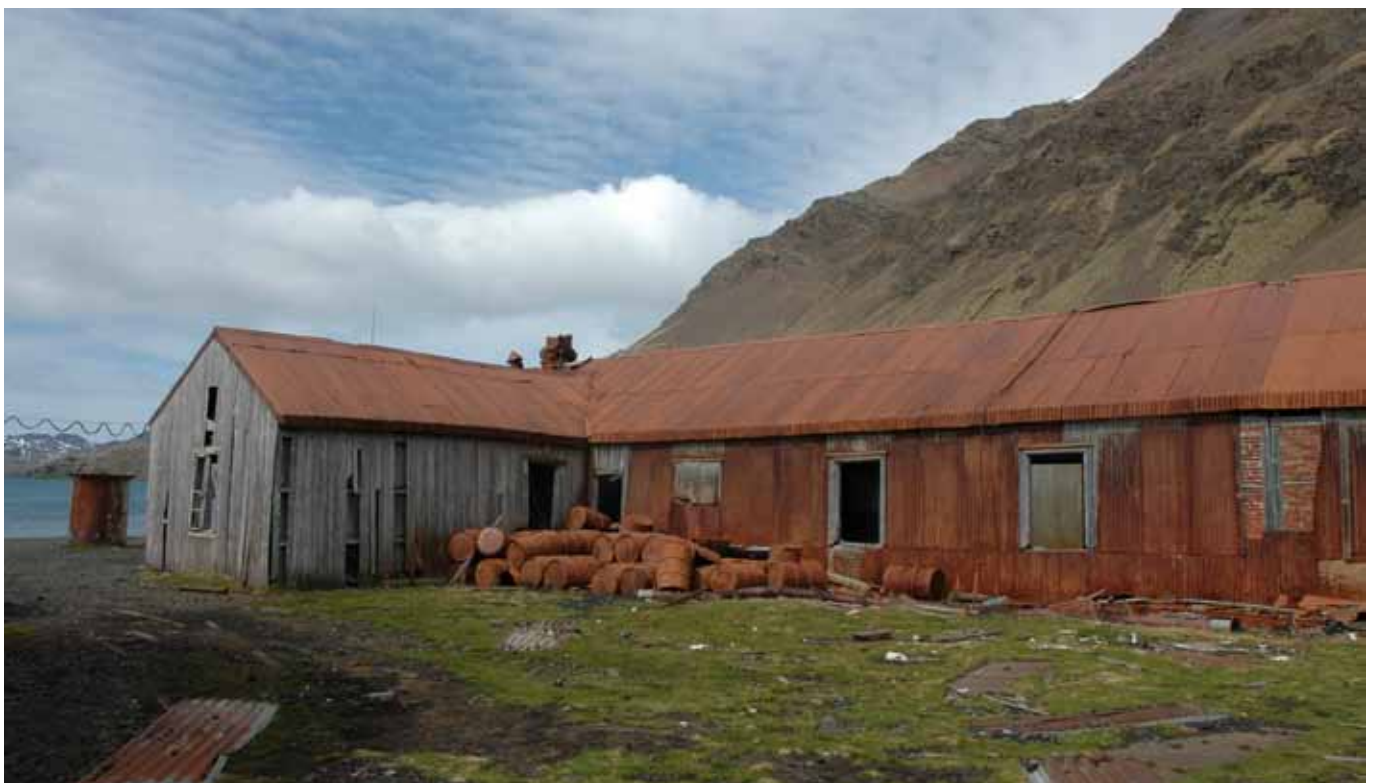
14.3 The north elevation of the main building and the north and west faces of the extension
