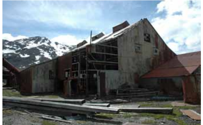
6.1 The southeast corner of the main building
