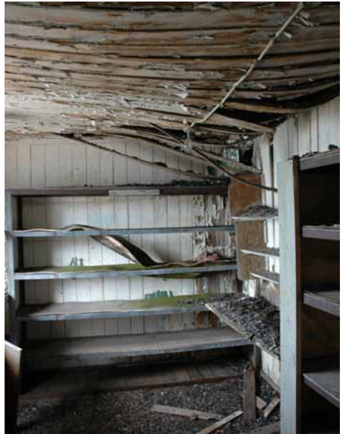
15.7 Ground floor Store Room
