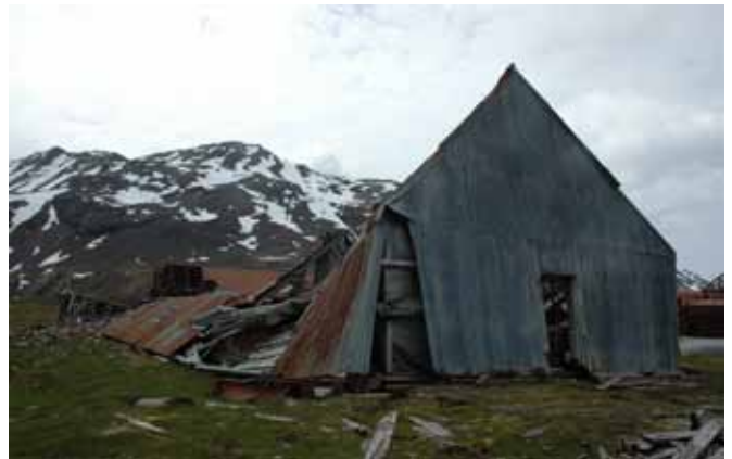
26.2 The south gable end
