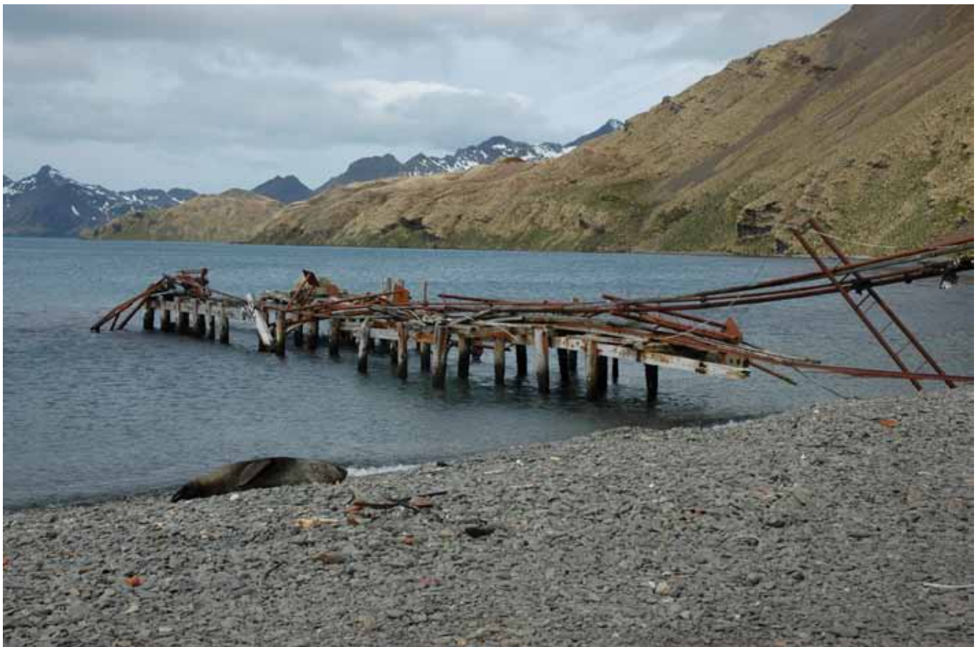
28.2 North side of Jetty No.28
