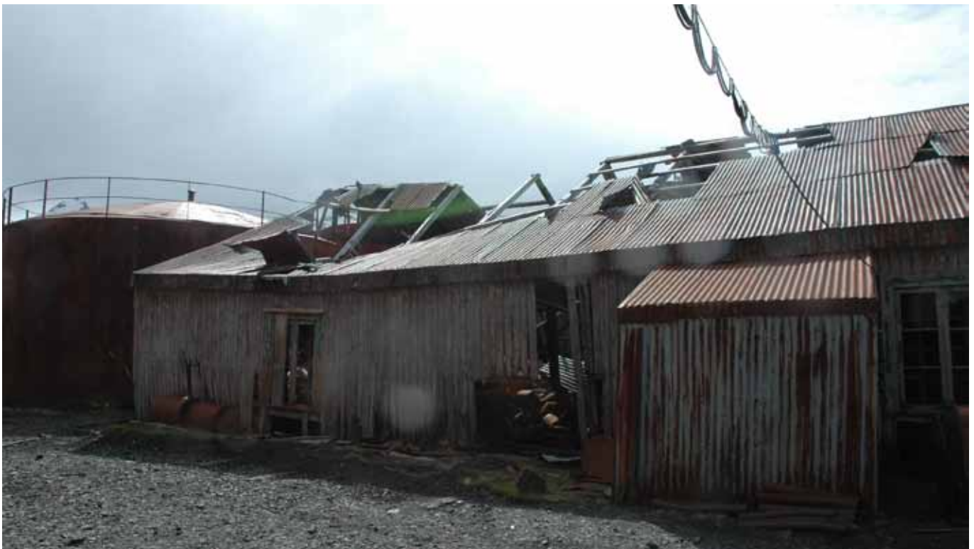
10.4 South elevation, west end with Tank 34 behind
