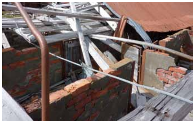
26.4 The rendered brick pens seen through the south door.
