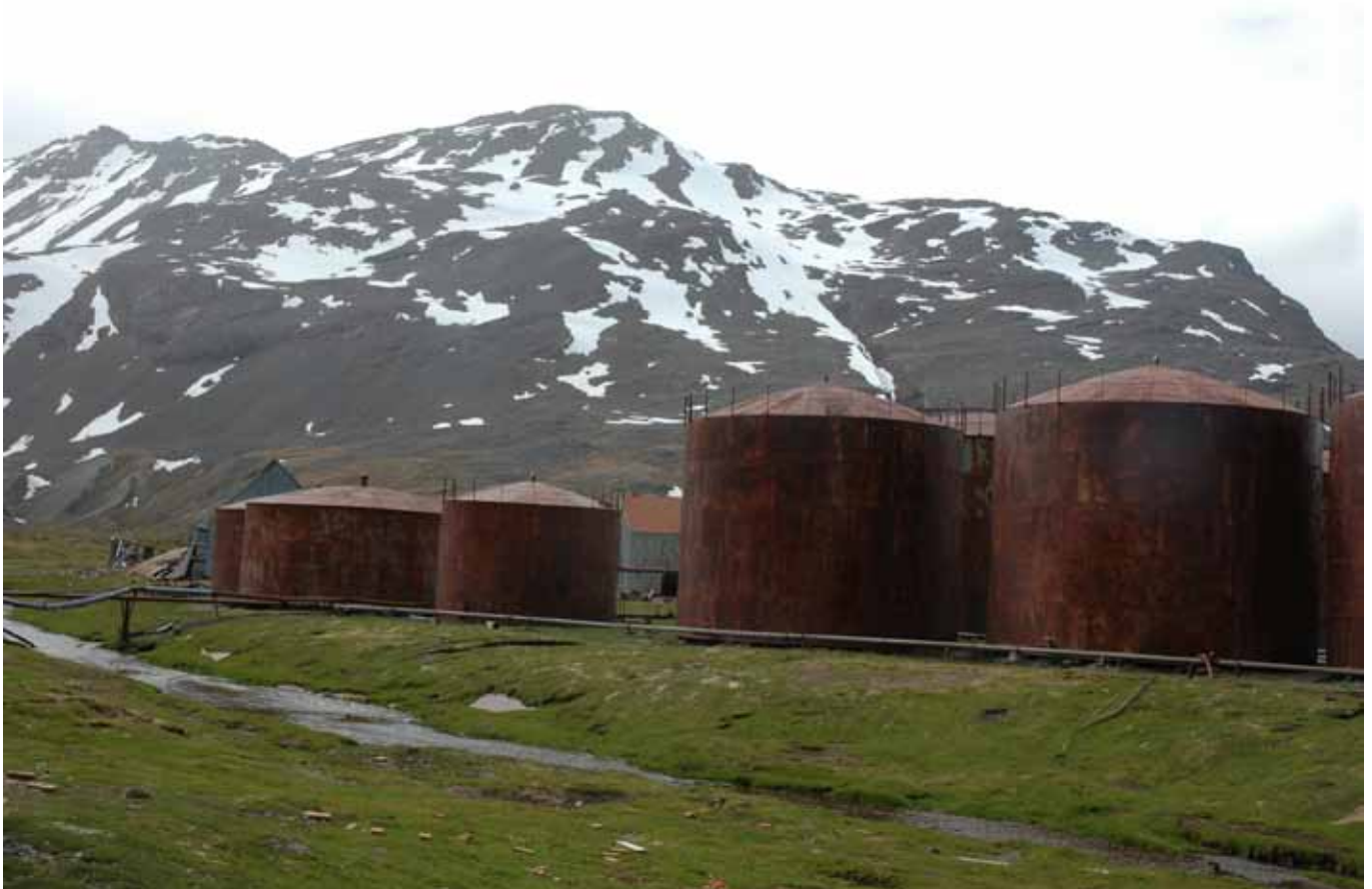
34.6 Tanks 43-47 looking northwards
