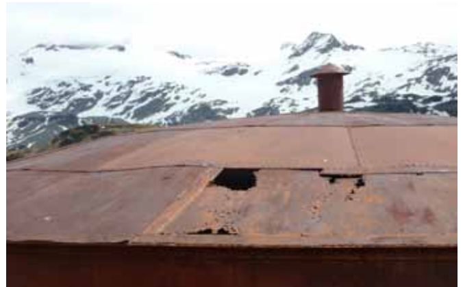
34.5 Roof of Tank No.47
