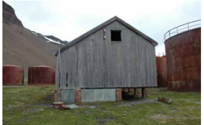
25.6 The east elevation. The passage extension to the south is easy to make out.
