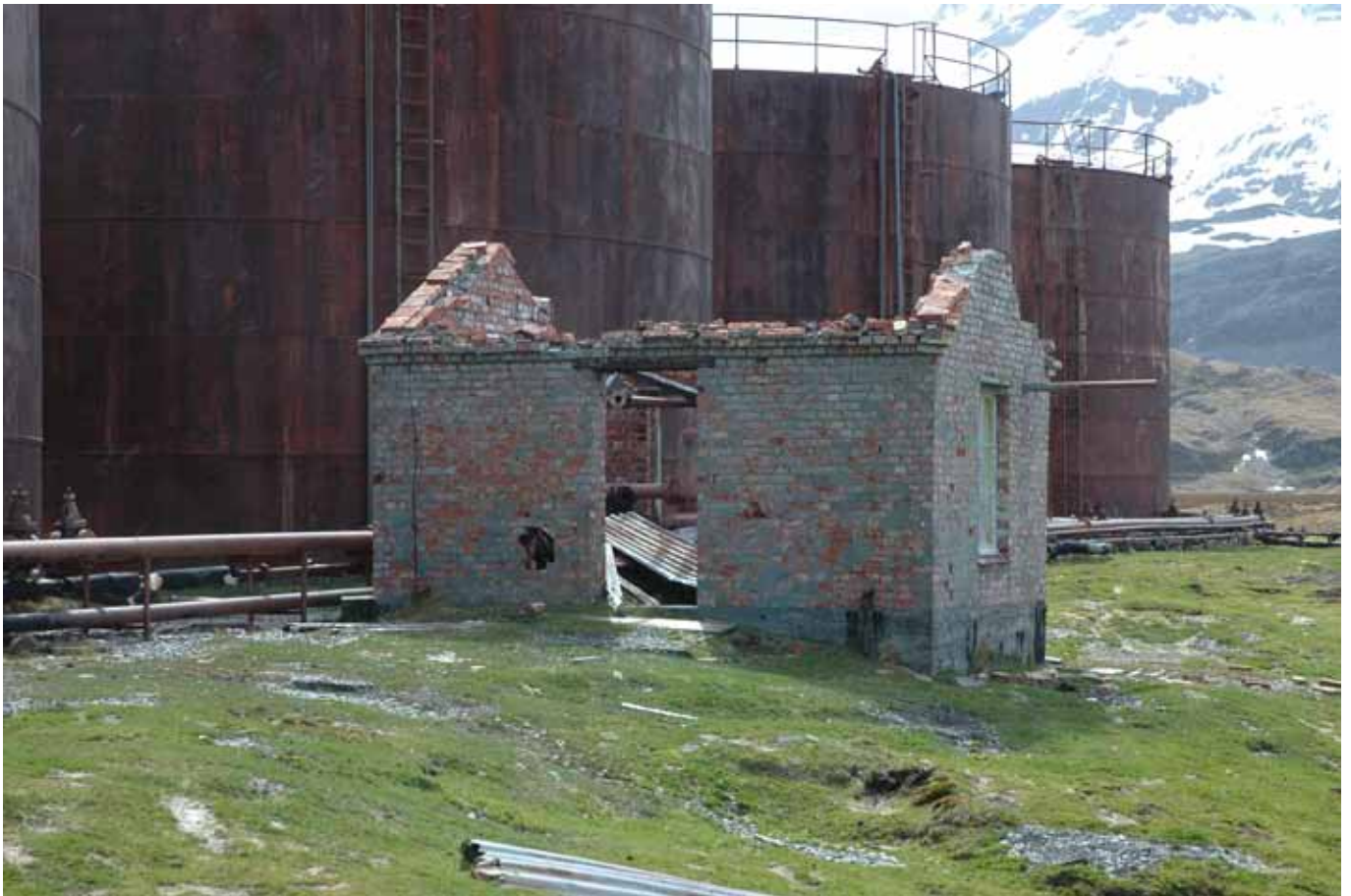
58.1 The south side of the building
