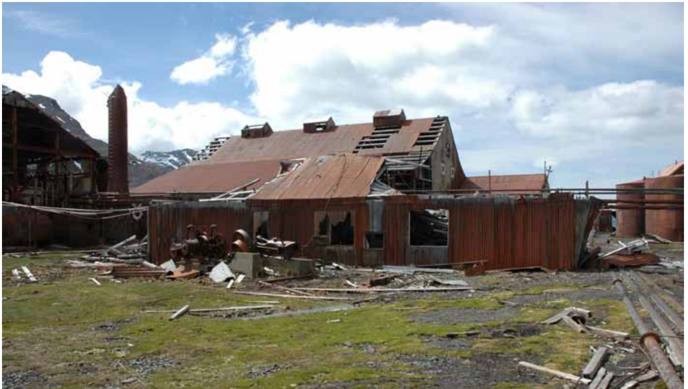
11.2 The west elevation with the Workshop (No. 6) in the background
