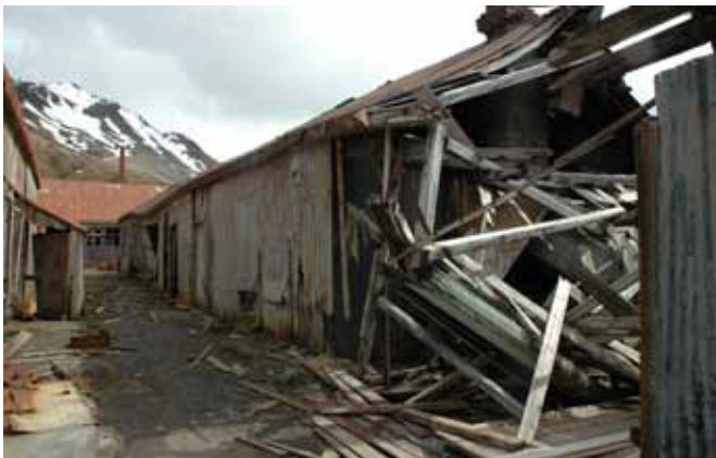
14.5 The collapse at the east end of the building
