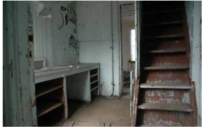
16.9 Kitchen and stair
