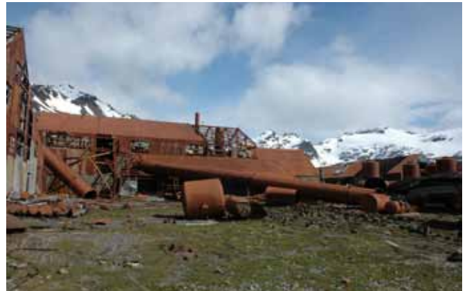
1.1 General view of the Plan looking west to the Boiler House
