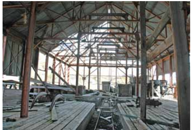
4.3.5 The interior looking west
