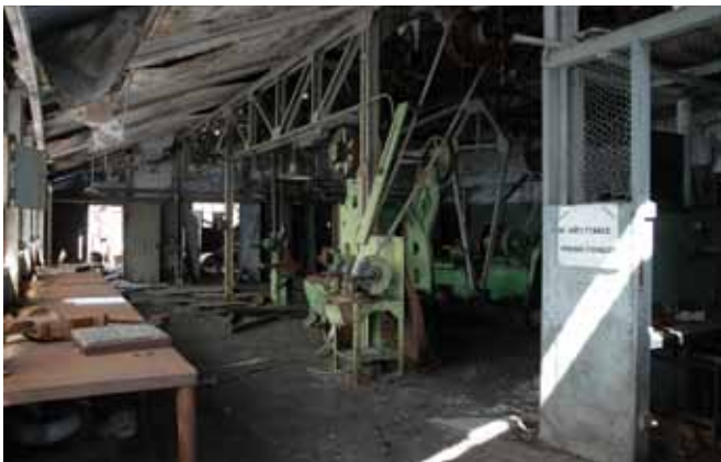
6.3 The Workshop on the east side of the building
