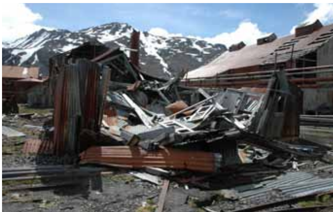
11.3 The south end of the building
