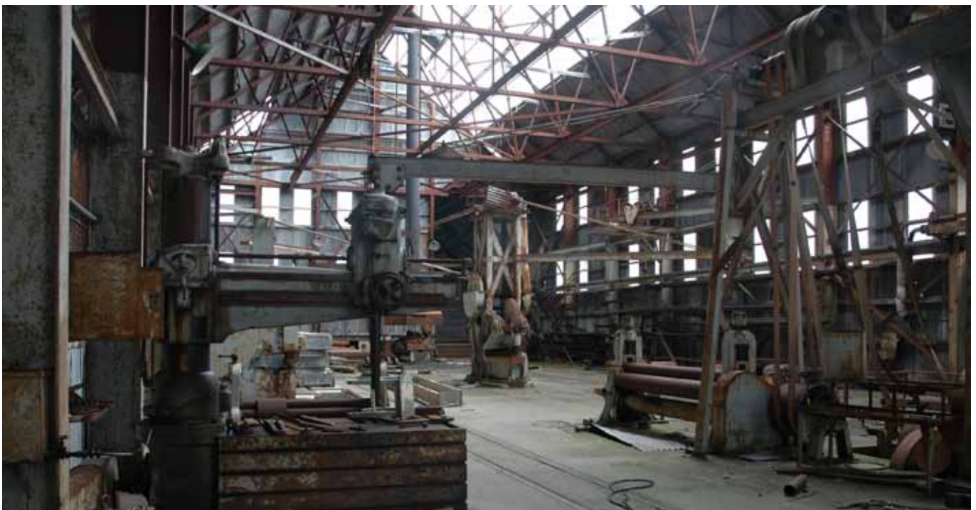
19.4 Interior of the main space looking west
