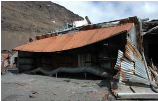
8.2 The lean-to on the south end of the east side
