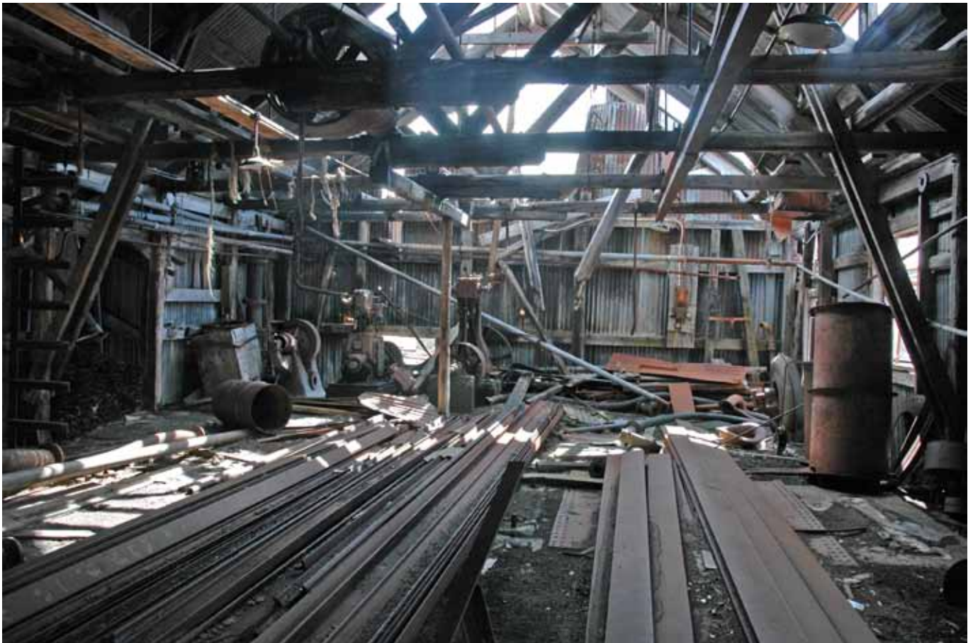
12.6 The interior of the main wing looking northwards
