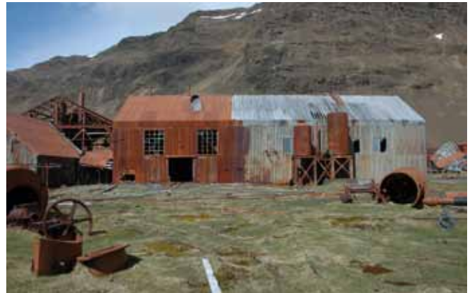
5.1.1 North elevation of the West Wing
