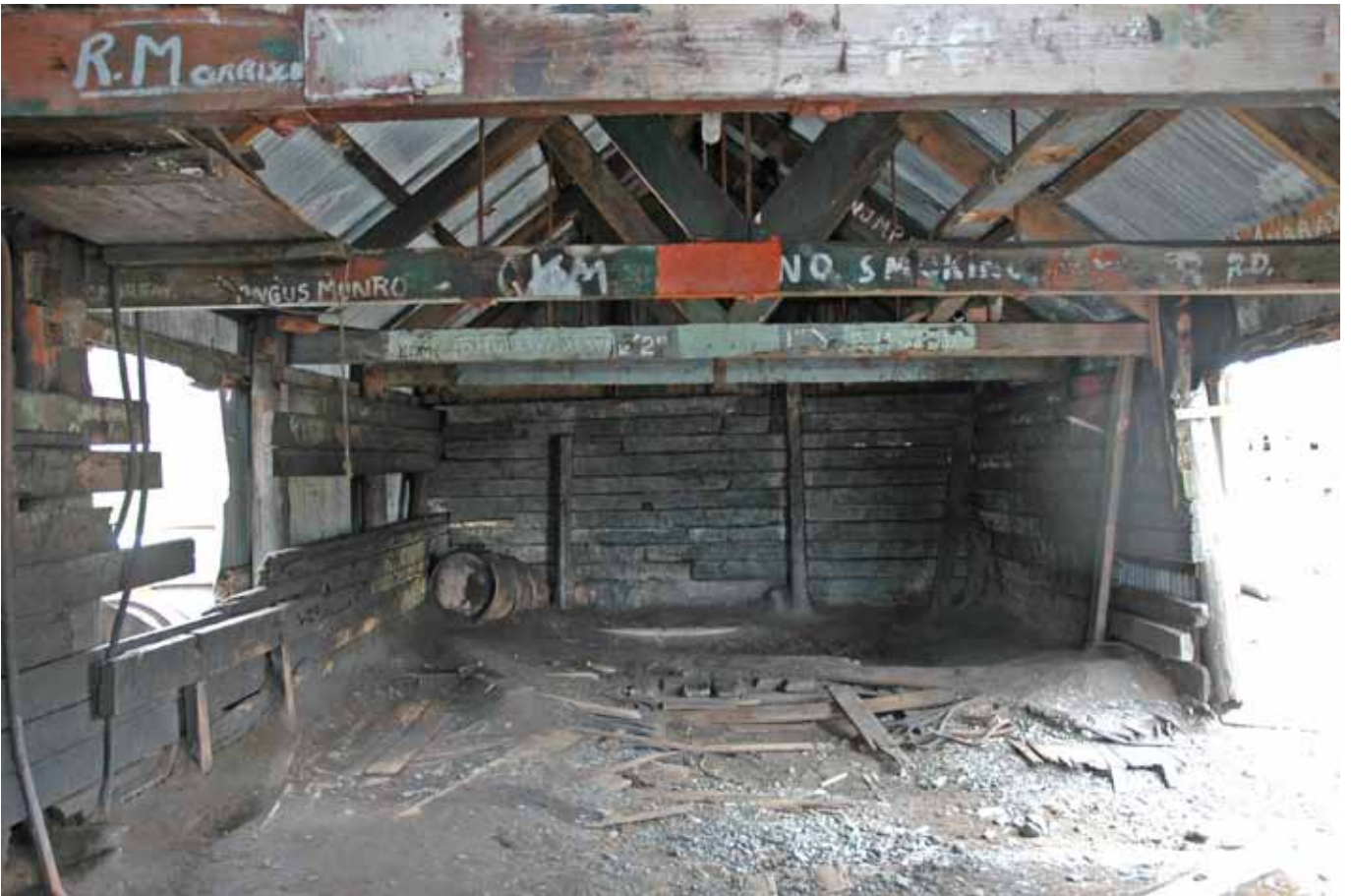
21.4 The interior looking west
