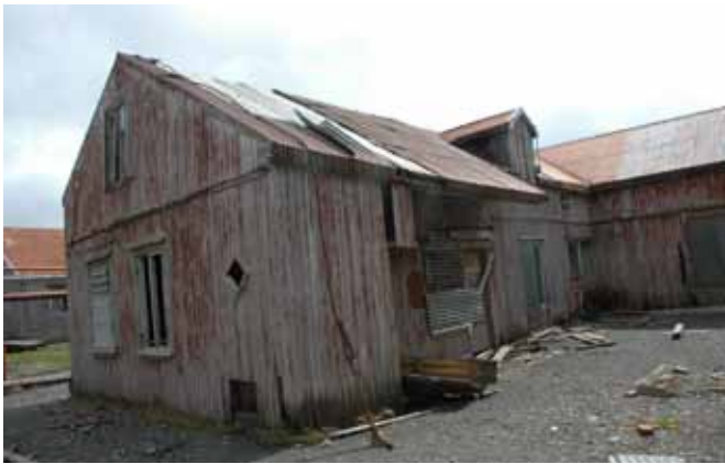
15.4 The south and east elevations of the west wing
