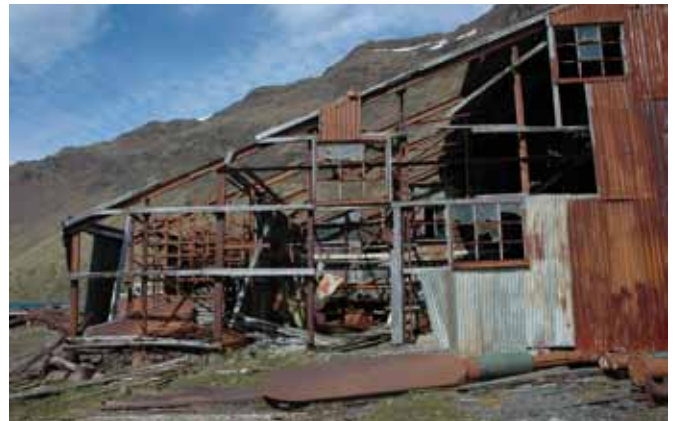
6.6 The northeast corner of the building
