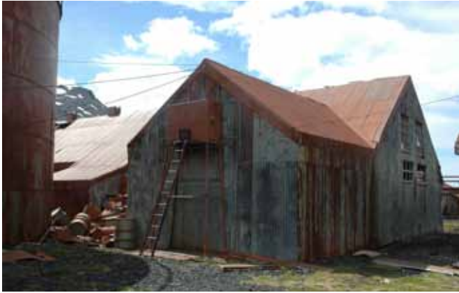
12.4 The south elevation of the main wing and the extension
