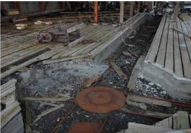
4.3.4 The lowered railway track and turntable
