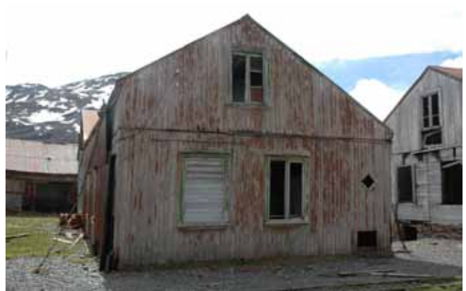
15.1 South elevation of the west wing
