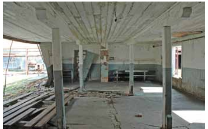
14.6 Interior of the Mess Room space
