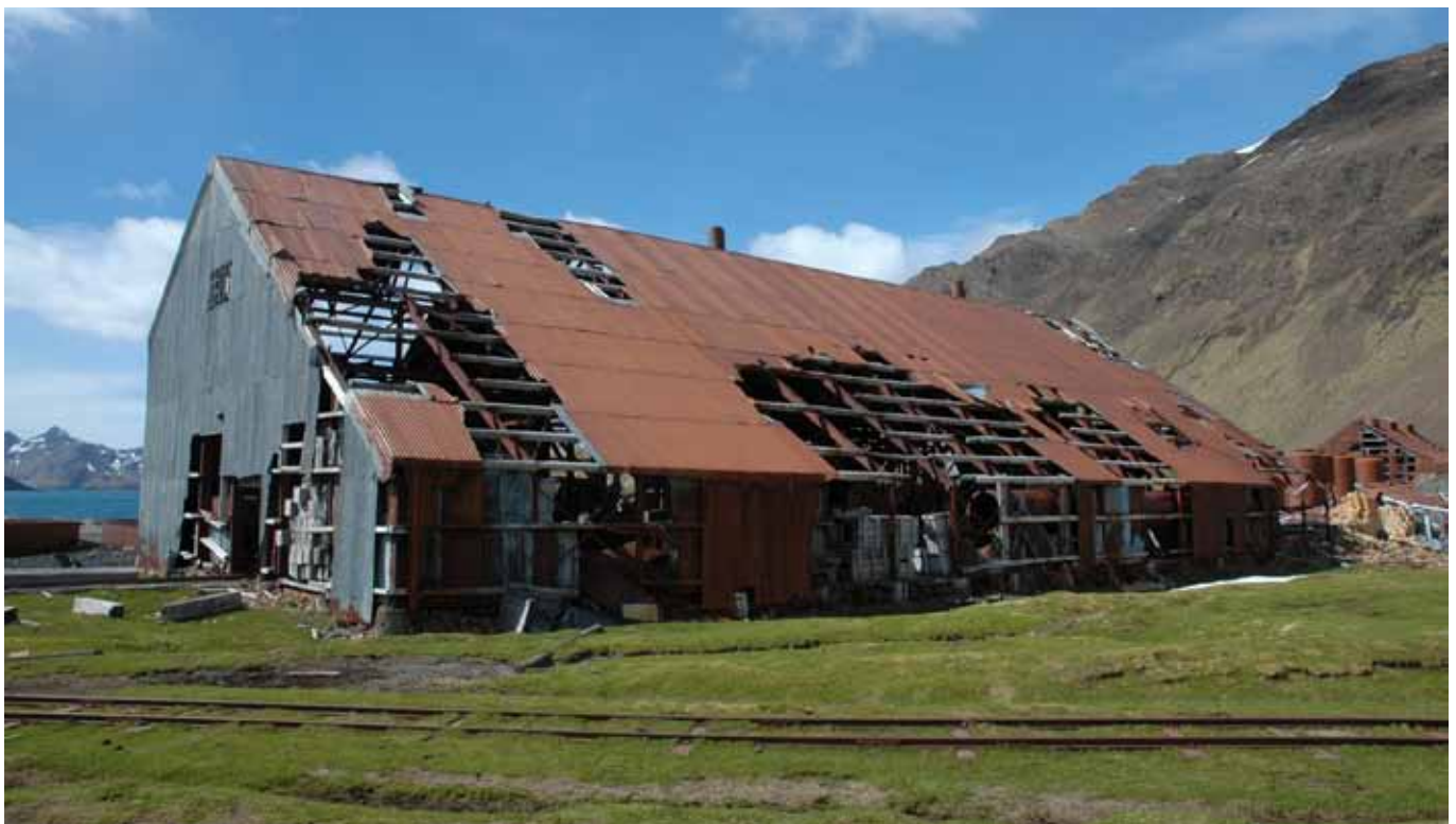
4.1.3 The west elevation of the North Wing
