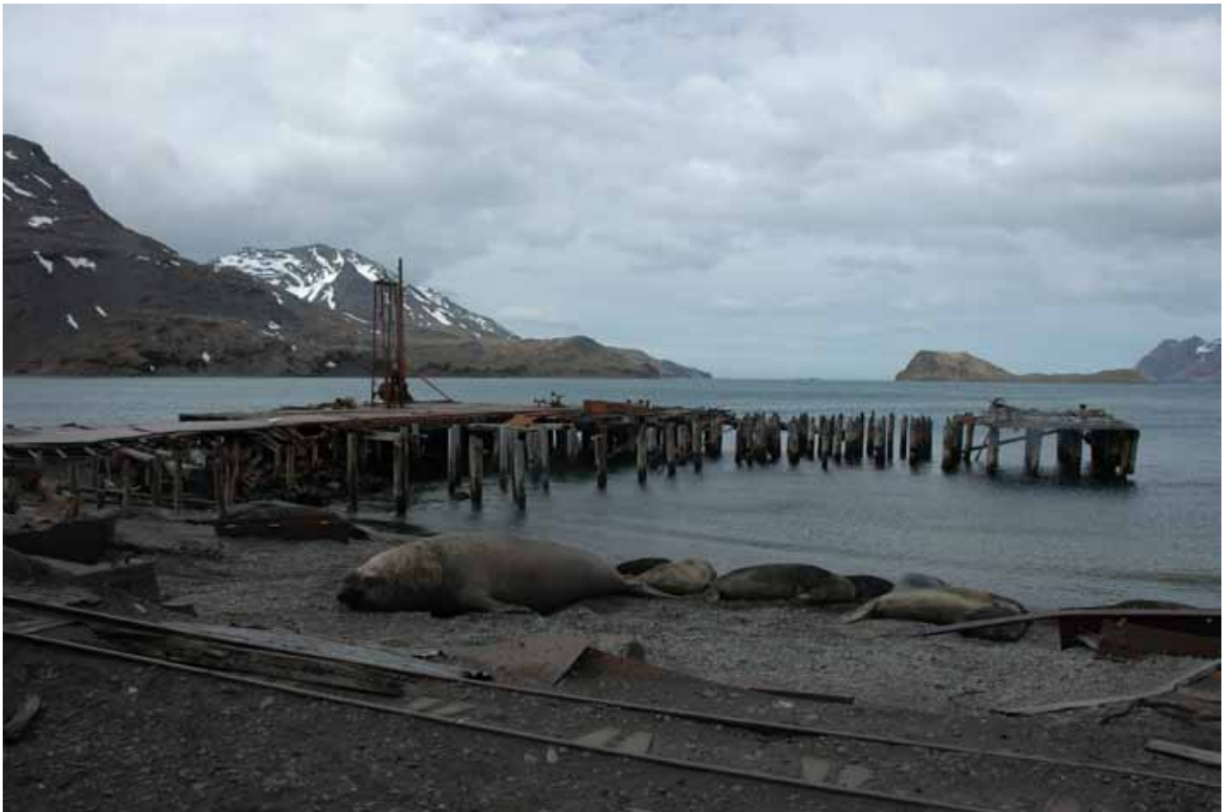
30.2 General view of the south side of the Jetty
