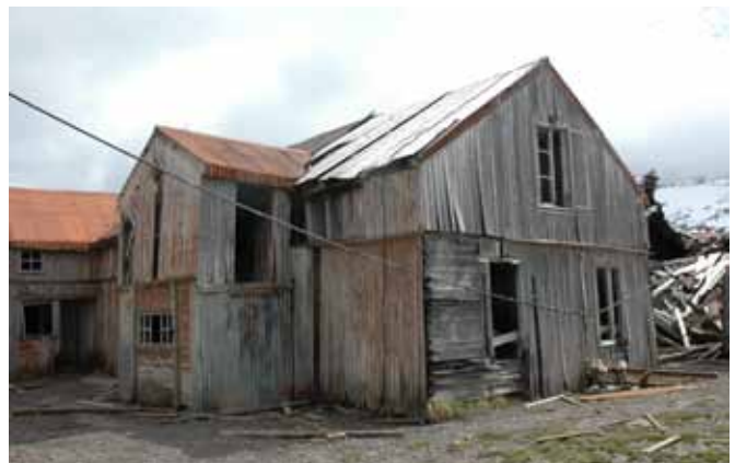
15.2 East elevation of the north wing
