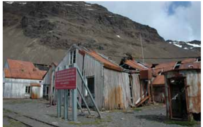
14.2 The east elevation and part of the north
