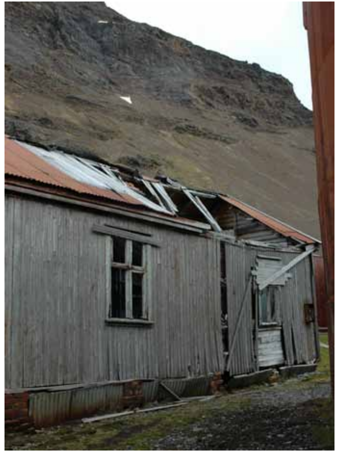
25.1 The northwest corner
