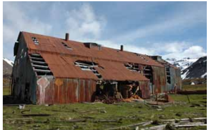
4.1.2 The east elevation of the North Wing
