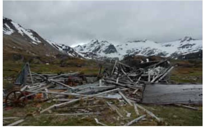
27.2 The centre of the building looking west
