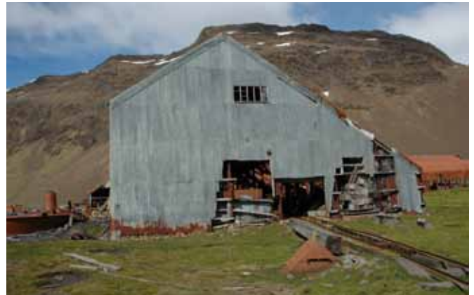
4.1.1 The north elevation of the North Wing
