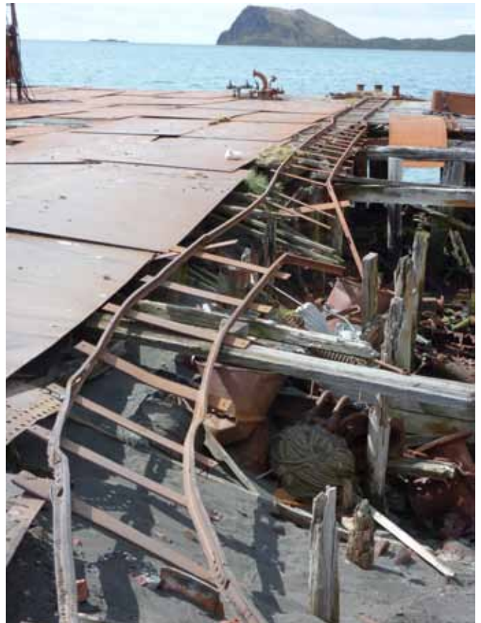
62.3 Tracks running out onto Jetty 30
