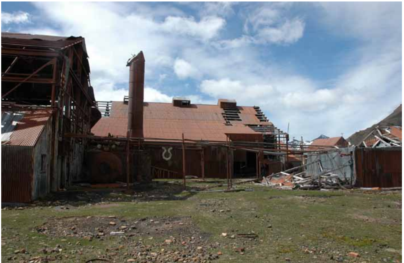
6.2 The west elevation of the South Wing which contains the Forge
