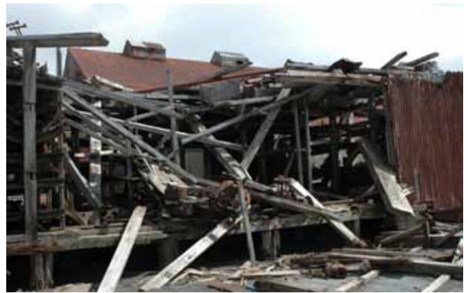
8.3 The central section of the building
