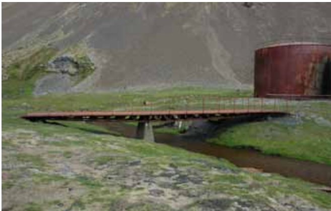
33.1 North side of bridge
