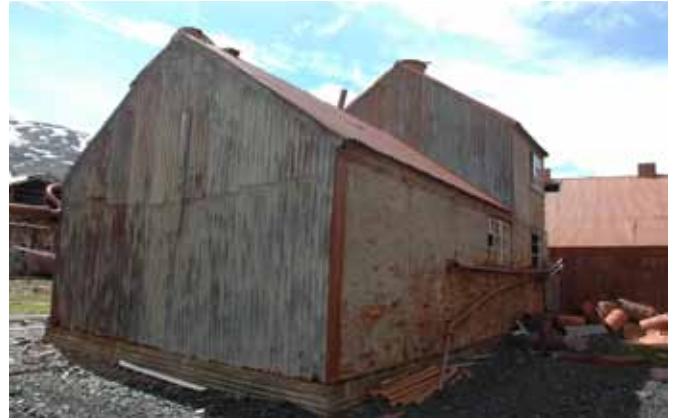
12.5 The west and south elevations of the northwest wing
