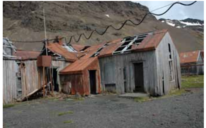
14.1 The extension to the north side of the building
