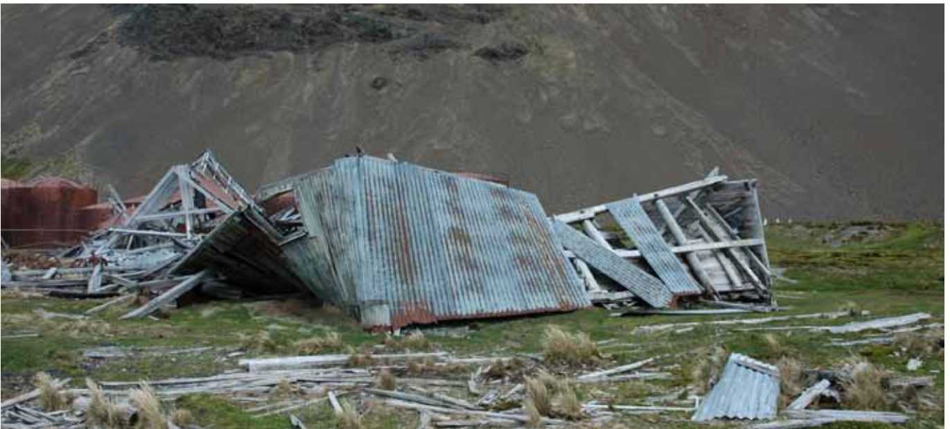
27.3 The northeast corner of the building
