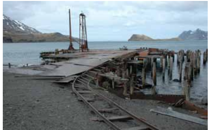
30.1 Railway running onto the Jetty
