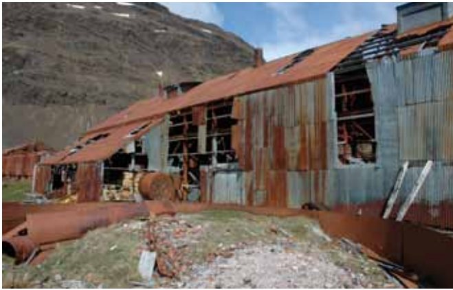
4.1.4 The east elevation of the North Wing
