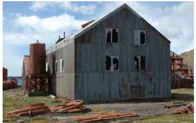
5.1.2 West elevation of the West Wing
