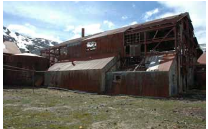
5.2.1 The west elevation of the Boiler House
