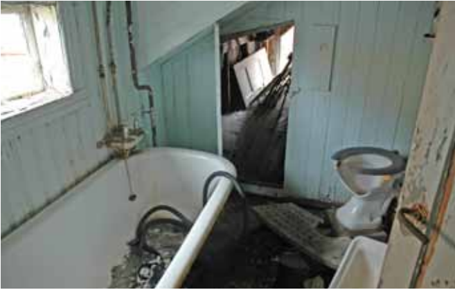
16.6 First floor bathroom
