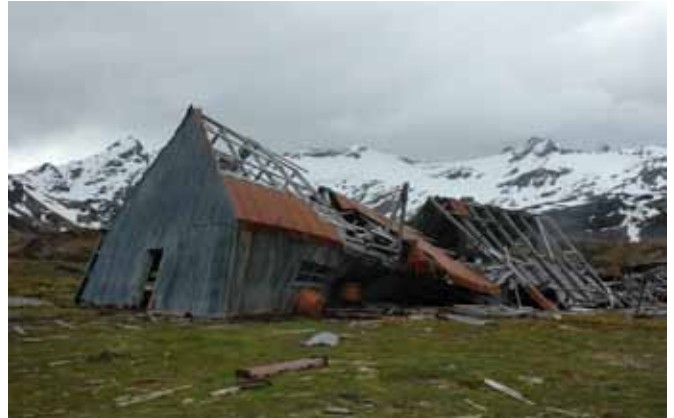
26.1 South and east elevations
