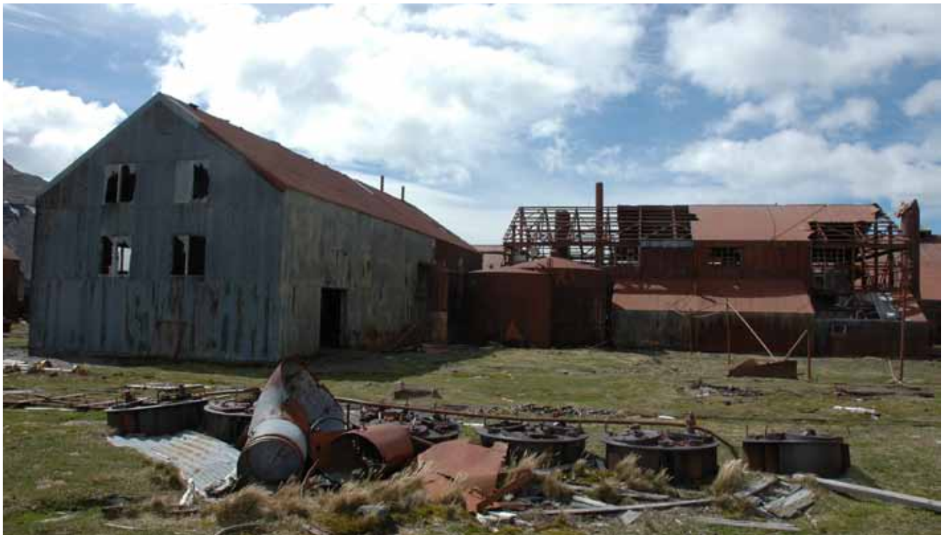
5.1.3 West and south elevations of the West Wing (the Power Station) with the Boiler House to the right
