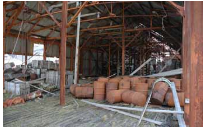
4.3.1 Interior of the West Wing looking east from the west end
