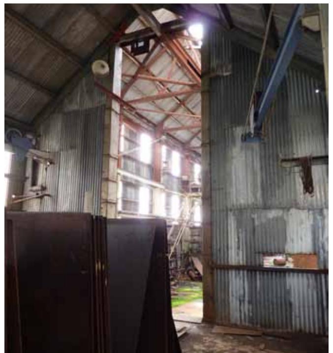
19.7 The opening between the steel store and main building
