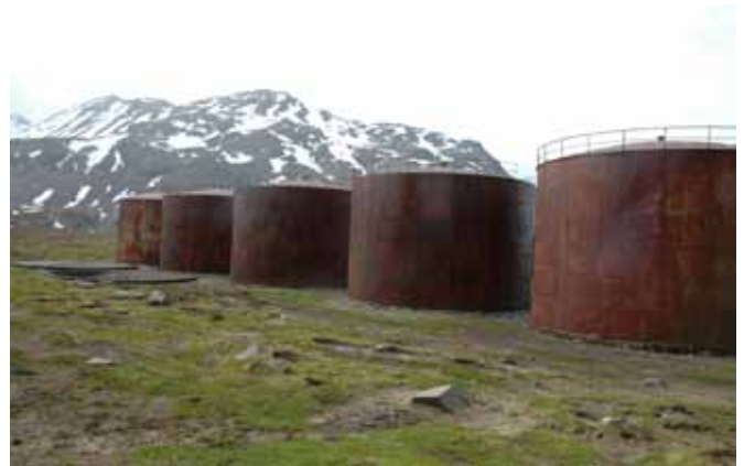
34.2 Tanks 52-57 east side
