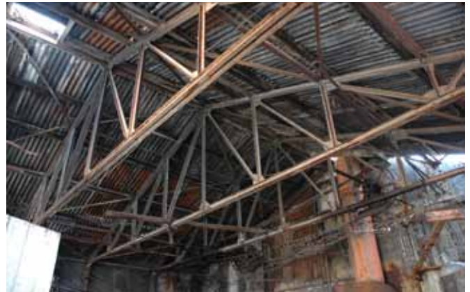
6.5 The roof of the Forge
