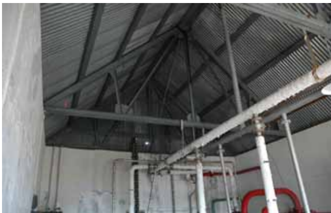
9.3 Interior of roof looking west
