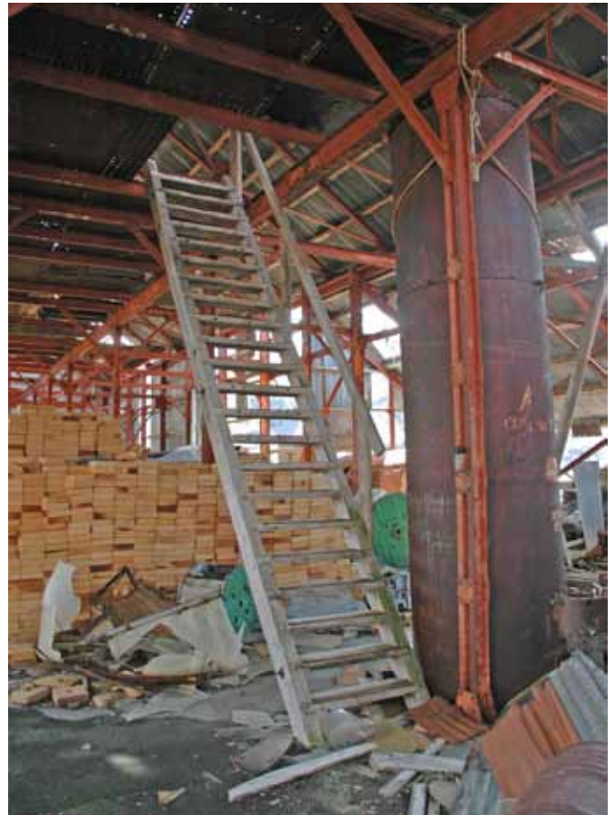
4.1.6 The stair to the upper deck
