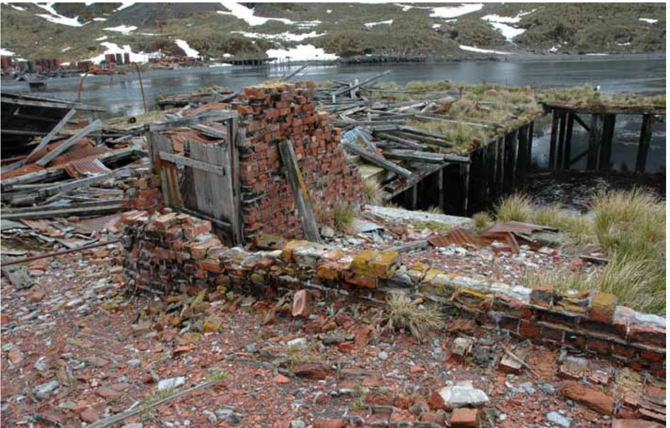
29.3 The Jetty can be seen beyond the Jetty Store. The brick remnant in the foreground may be part of the Boiler House (No. 30).
