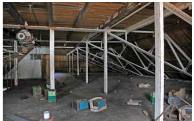
40.4 The upper floor storage space
