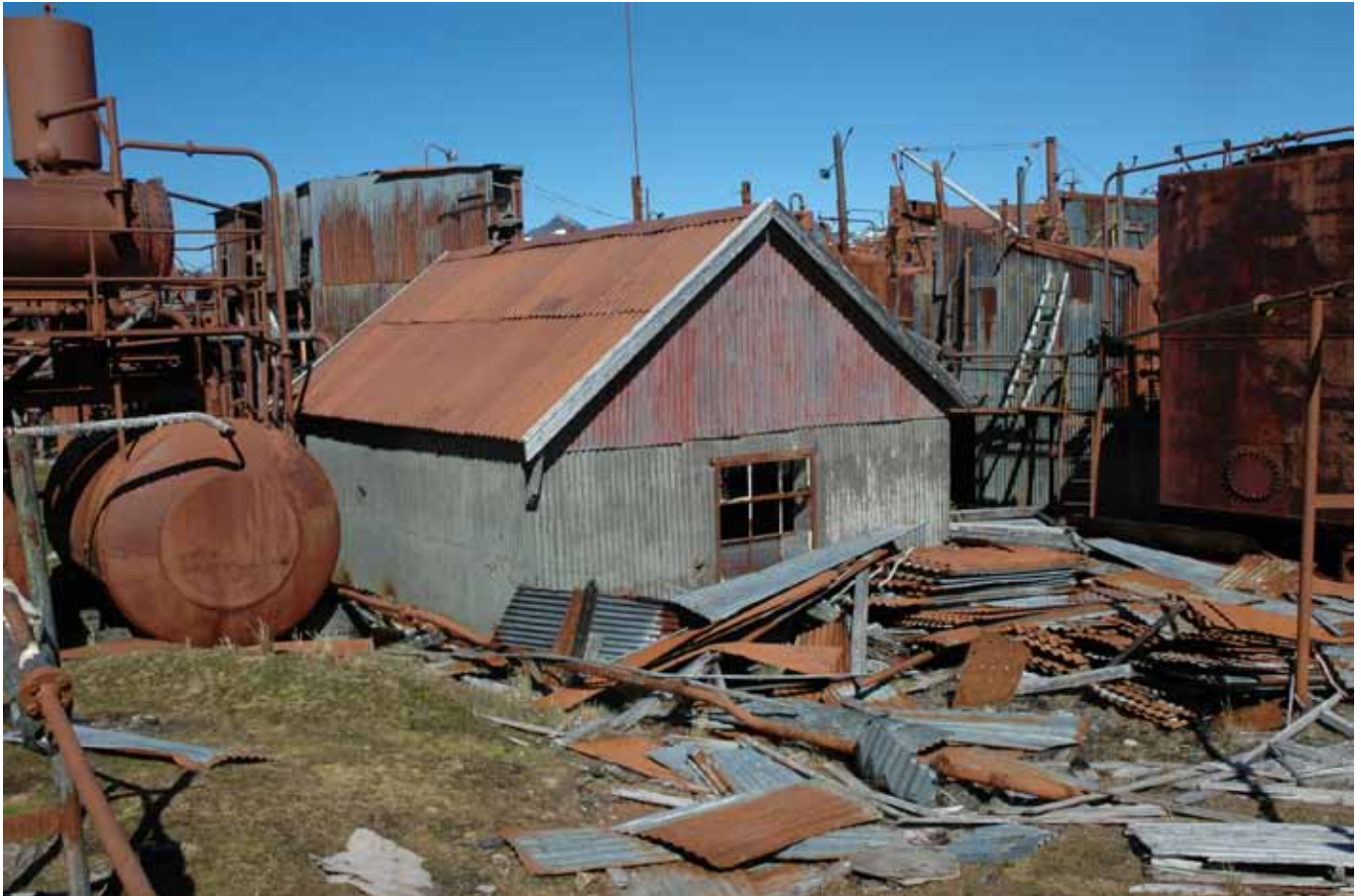
23.2 North and west sides of the building
