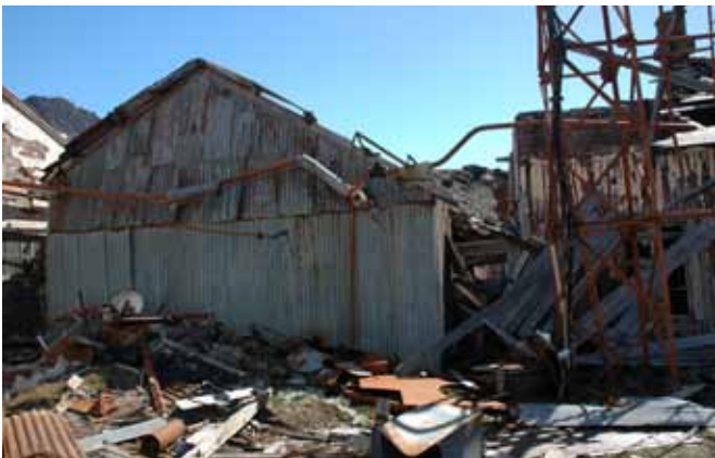
53.6 The southeast elevation of the main wing
