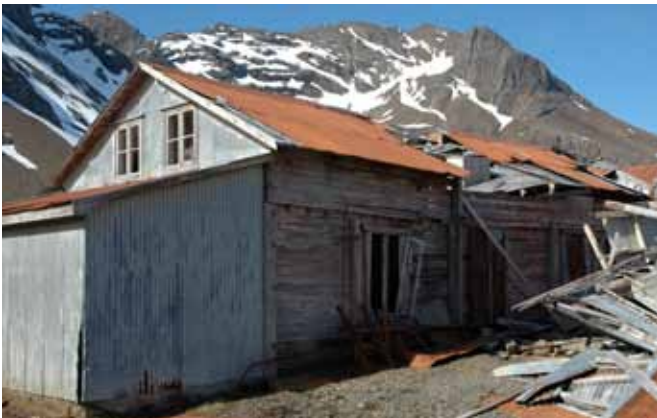
64.1 The south side of the building looking east
