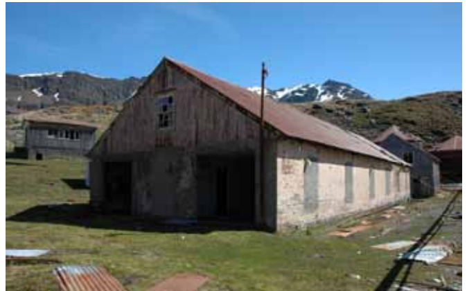
52.1 Southeast end and northeast elevation
