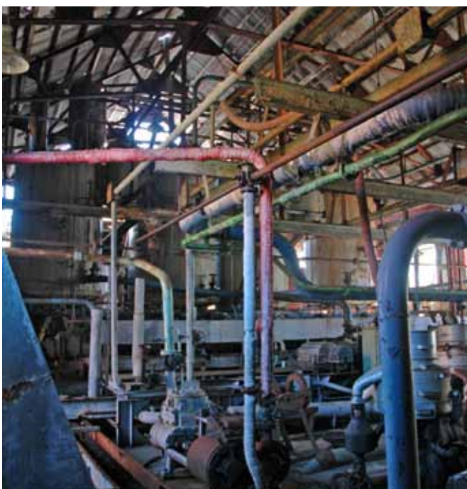
2.3 The interior of the east end of the building
