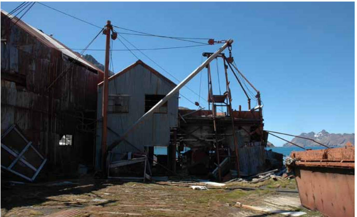
3.3 The west elevation. The large building to the right is No. 4 the Hartmann Plant.
