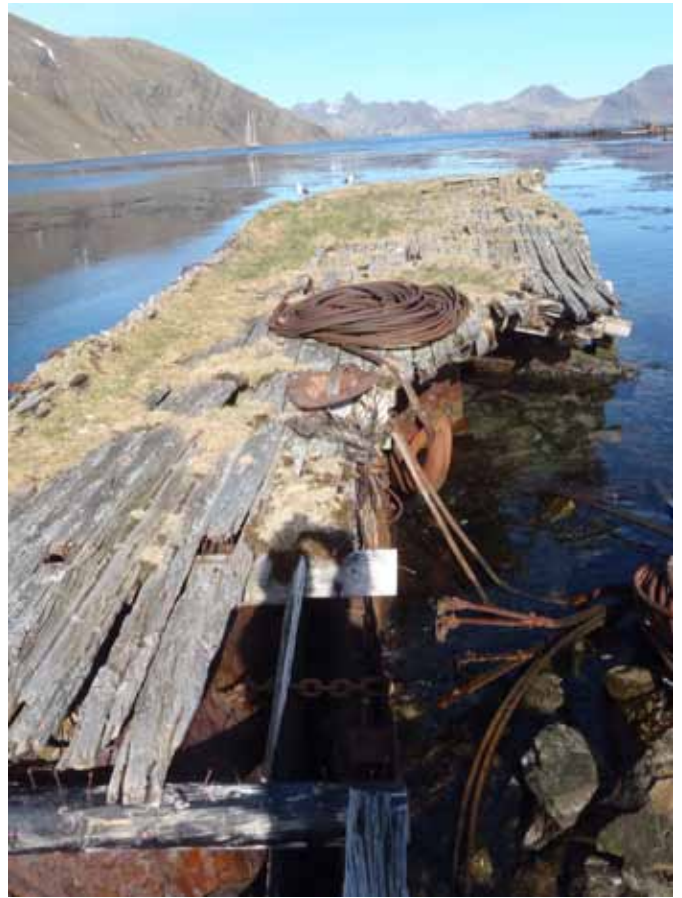
88.3 Detail looking along the deck
