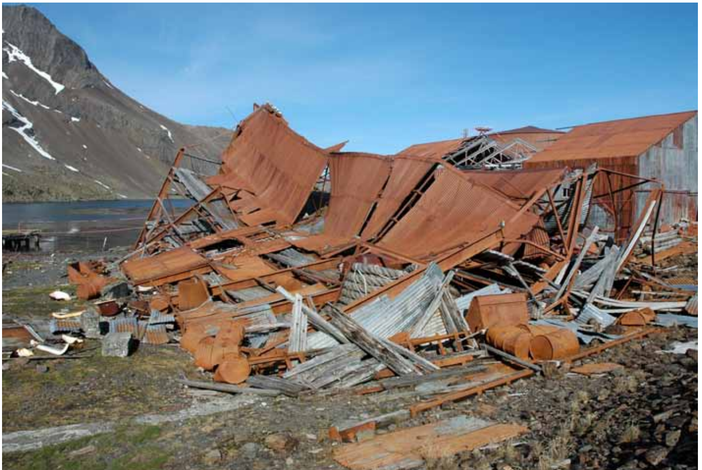
74.3 The west end of the building
