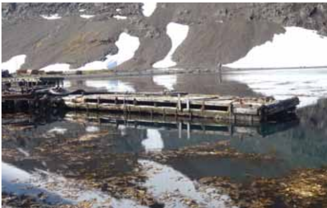
87.1 General view of the Pier looking northwards
