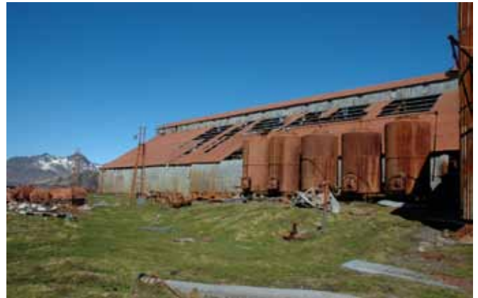
10.1 The east end of the north elevation
