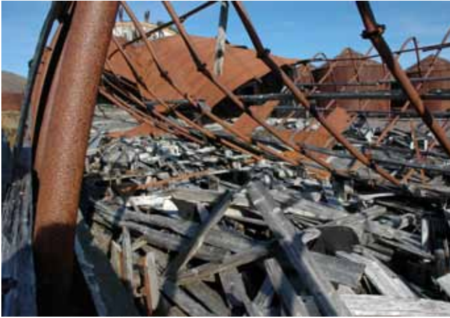
80.3 Looking eastwards along the north side of the building
