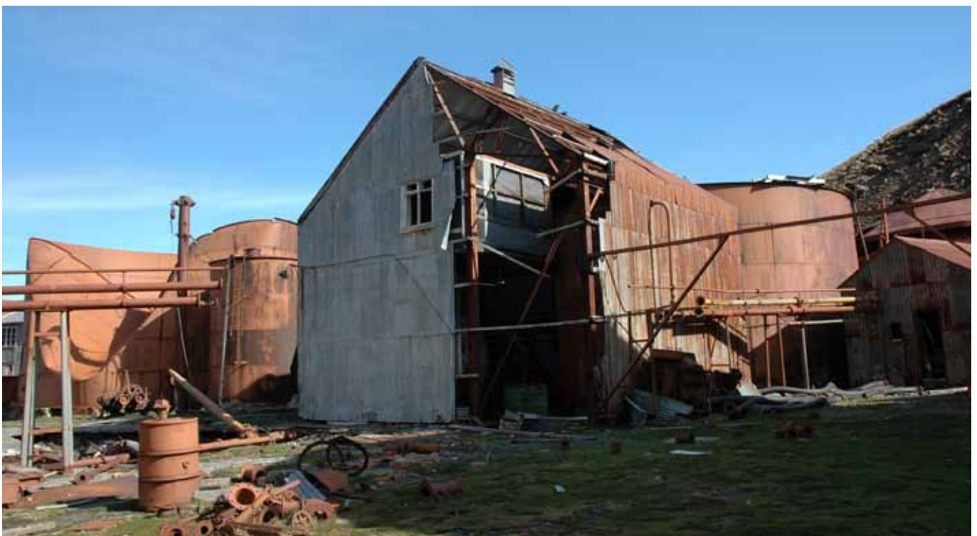
68.3 The northeast corner of the building
