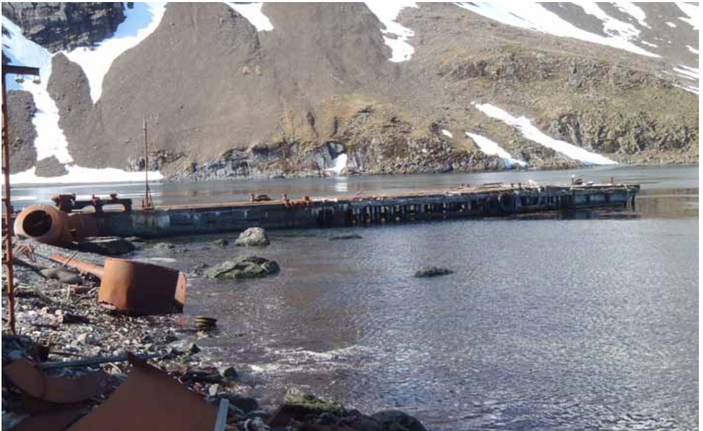
84.3 General view of the south side of the Pier
