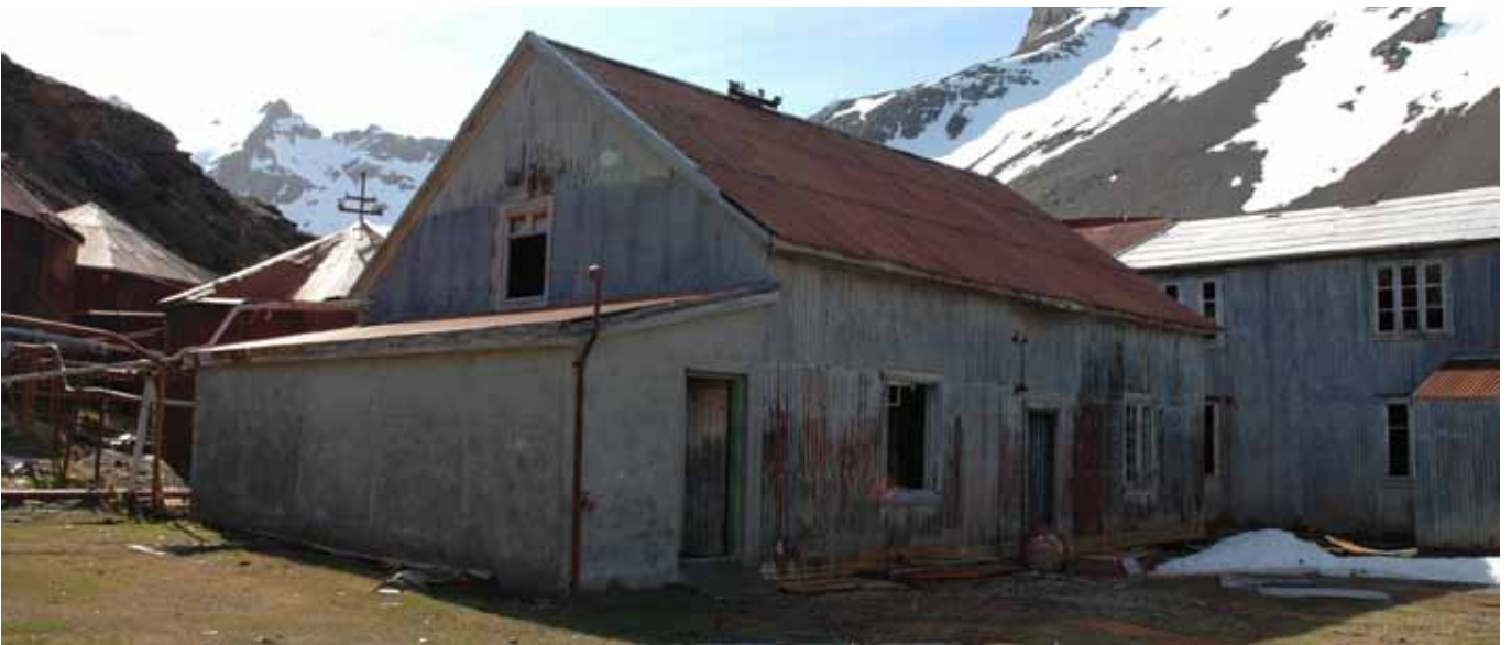
67.4 South and east elevations
