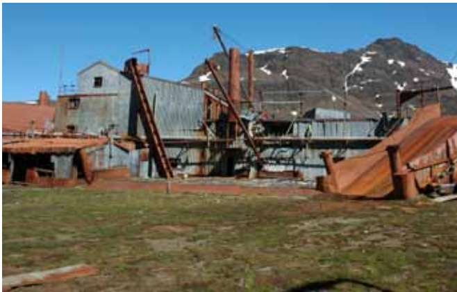
1.1 Looking southwest with the ramp to the bone loft on the right and the Rose Down Plant centre
