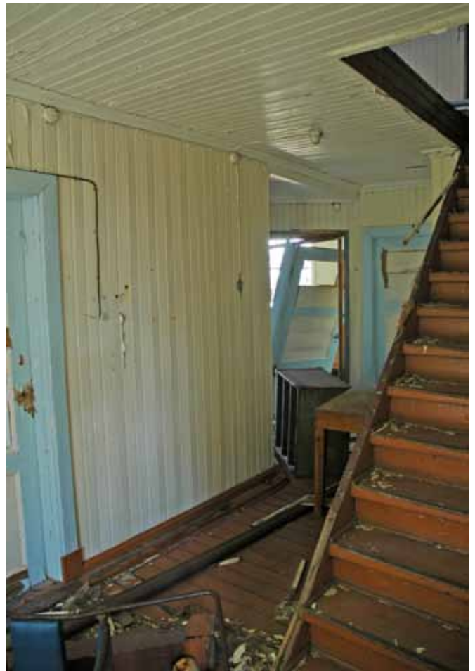
43.6 Central passage on ground floor
