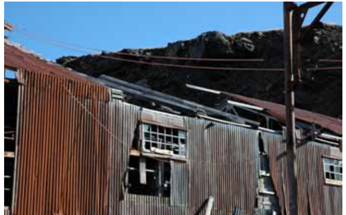
72.3 Detail of the north elevation
