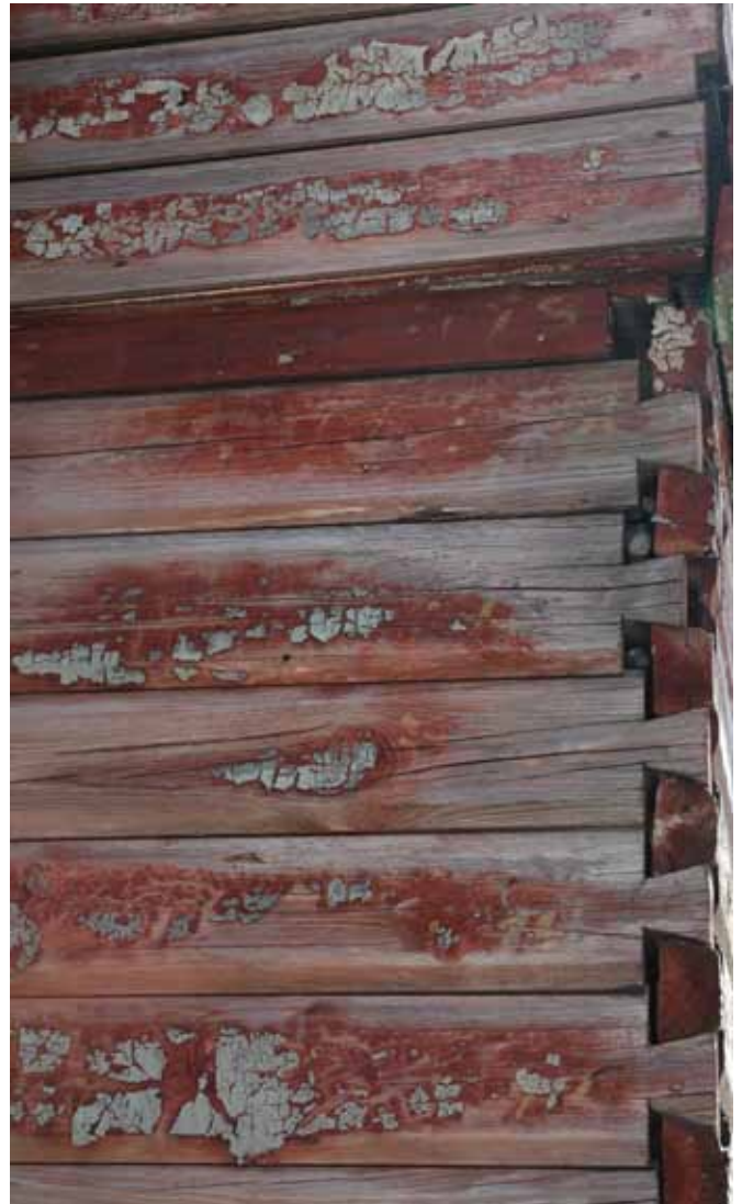
64.2 Typical corner detail of the original building
