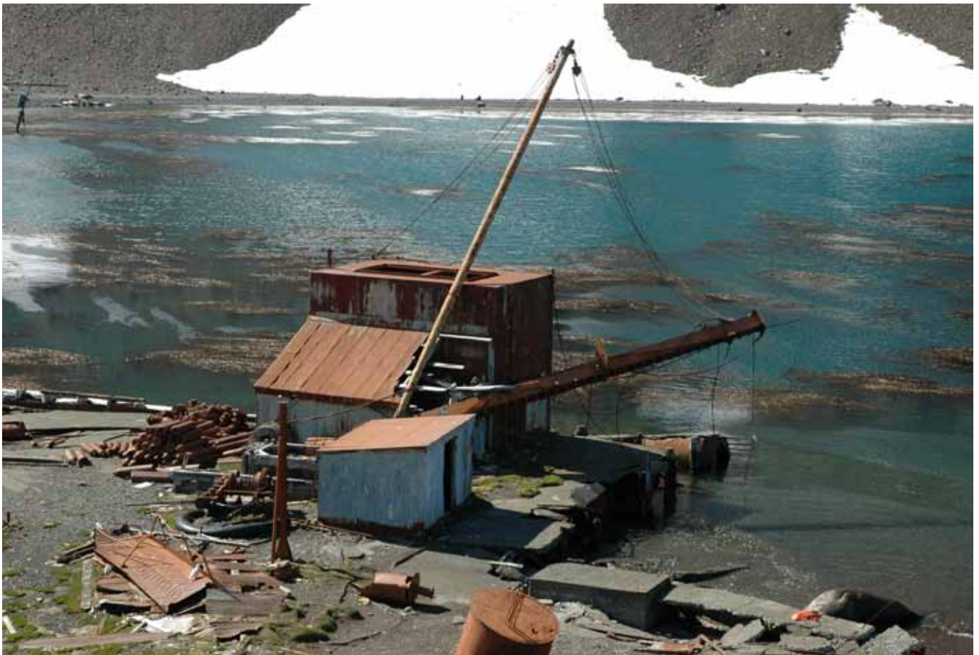
62.2 General view from the south (from Building No. 40)
