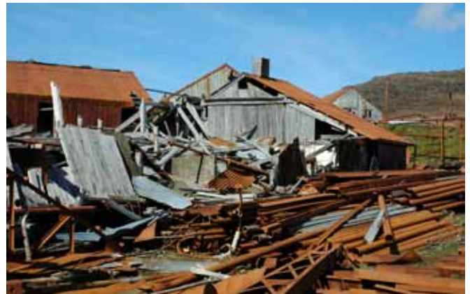
33.3 The northwest side of the building looking south
