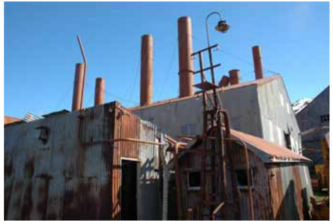
25.3 The north and east elevations seen behind Building Nos. 26 and 27
