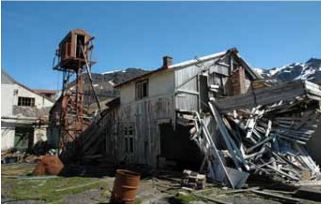
53.3 The northeast wing showing the southeast and northeast elevations
