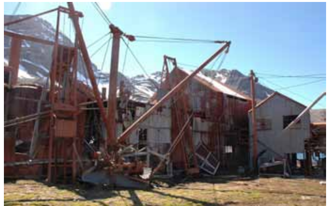
4.2 The south elevation of the building
