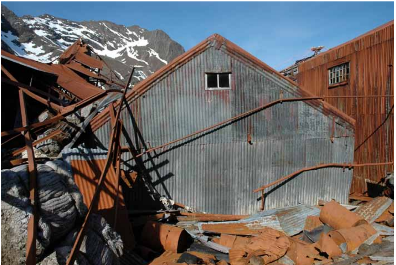
75.1 The remaining west wall of the Paint Store
