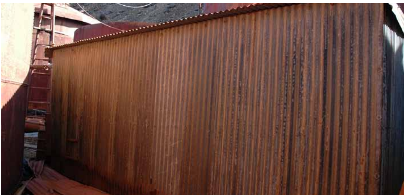
71.1 The south wall of the Butterworth Store
