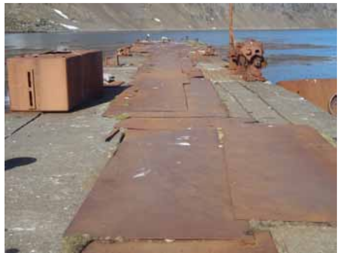
84.2 View along the Pier looking east
