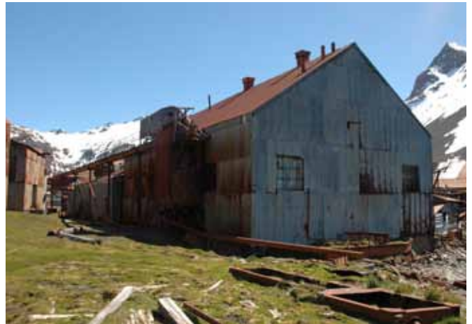
2.2 The south and east elevations
