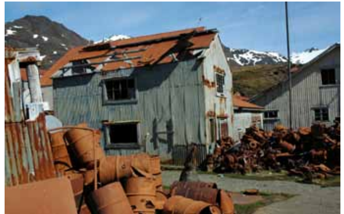
38.1 The two storey block on the southeast end of the building
