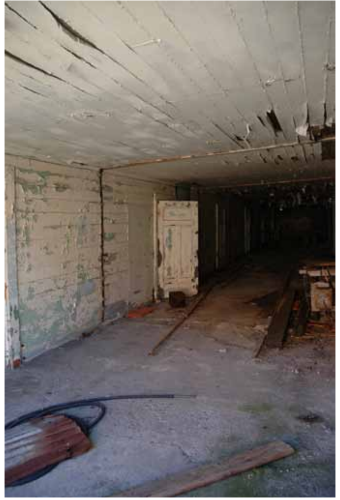
52.5 Ground floor storage area looking northwest
