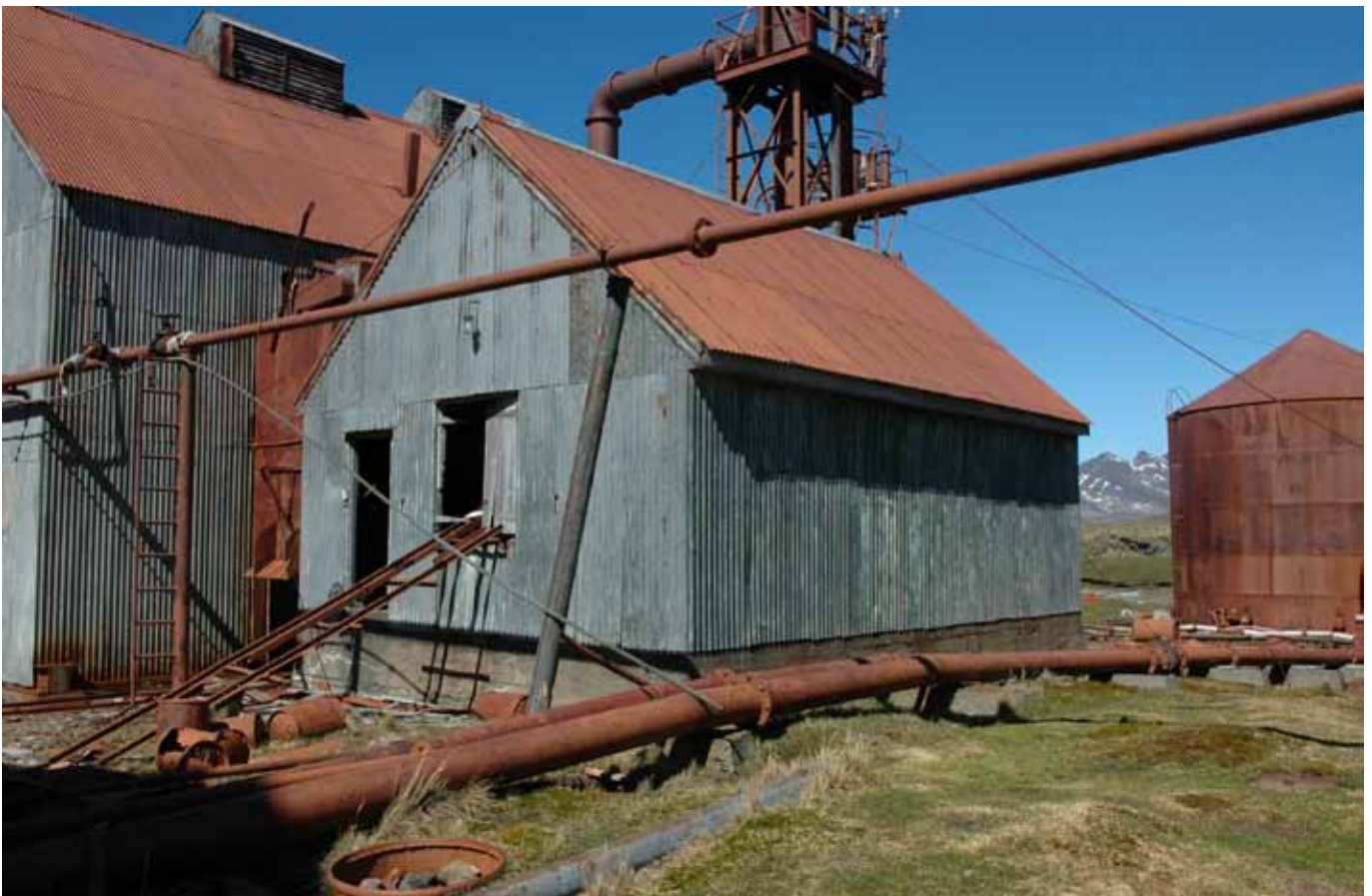
13.2 The north and west elevations
