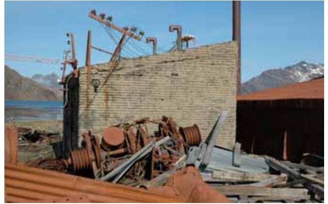
77.1 The west side of the Substation
