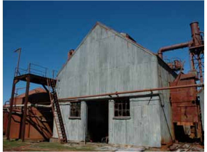
12.1 The north side of the building
