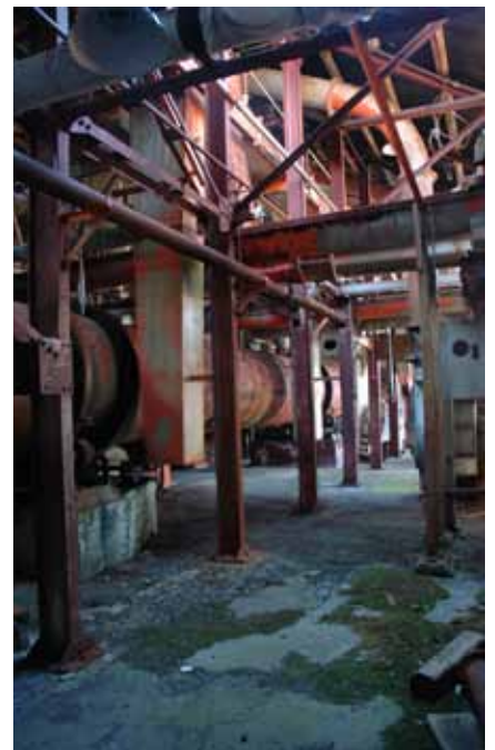
10.7 The west end of the main shed looking east and showing one of the rotary cookers
