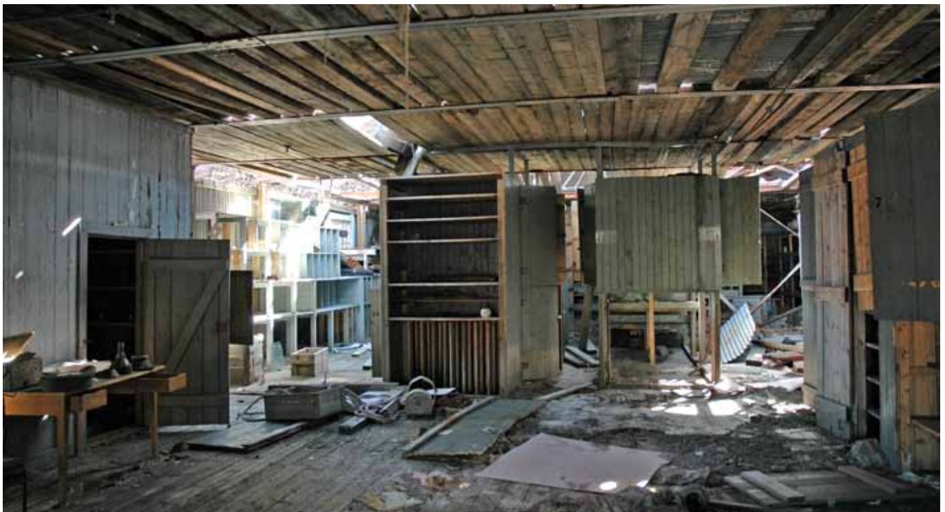
72.4 Ground floor storage area
