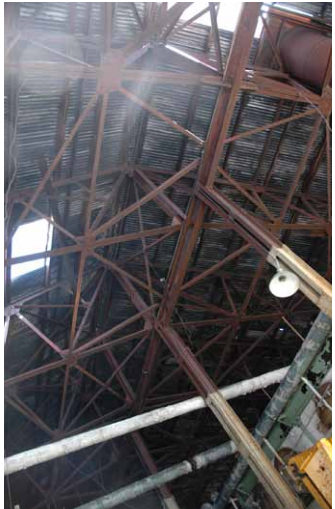
25.6 The roof structure
