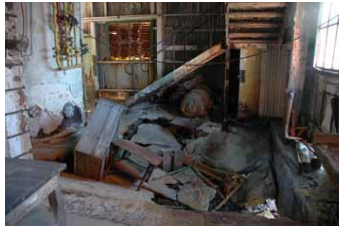
4.1 The interior of the east end of the building
