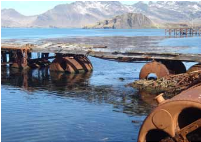
82.1 The connection to the shore at the west end of the Pier
