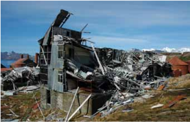
45.1 The north end and west side of Hillside Barracks
