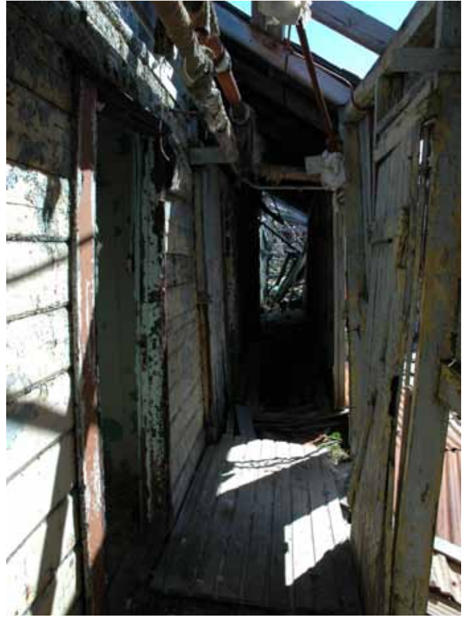
53.5 The added passage on the northeast side of the main wing
