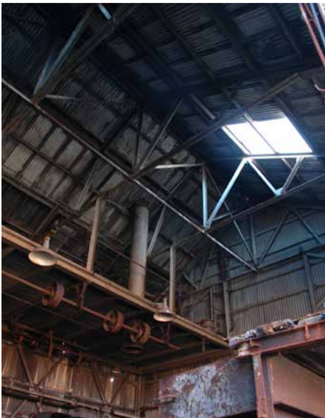
30.4 The roof structure
