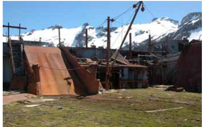
6.1 The ramp to the base lost at the north end of the east side
