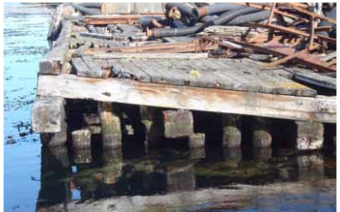
87.2 Detail of the Pier
