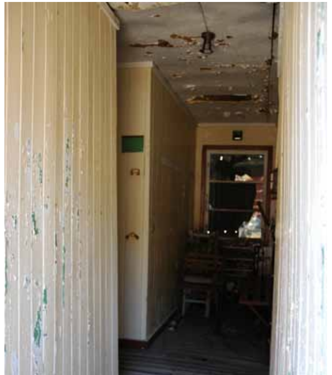
48.3 The entrance area looking east
