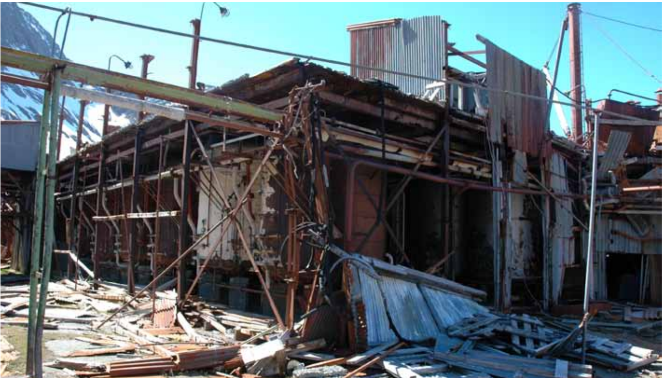
6.5 The southwest corner of the building
