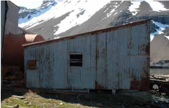
26.1 The south elevation of No. 26, the Battery Store
