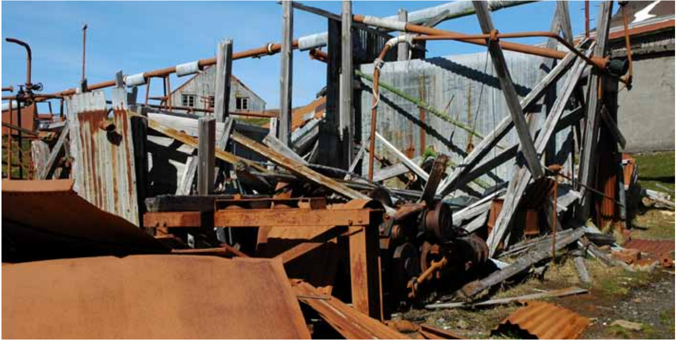
34.1 The east side of the building
