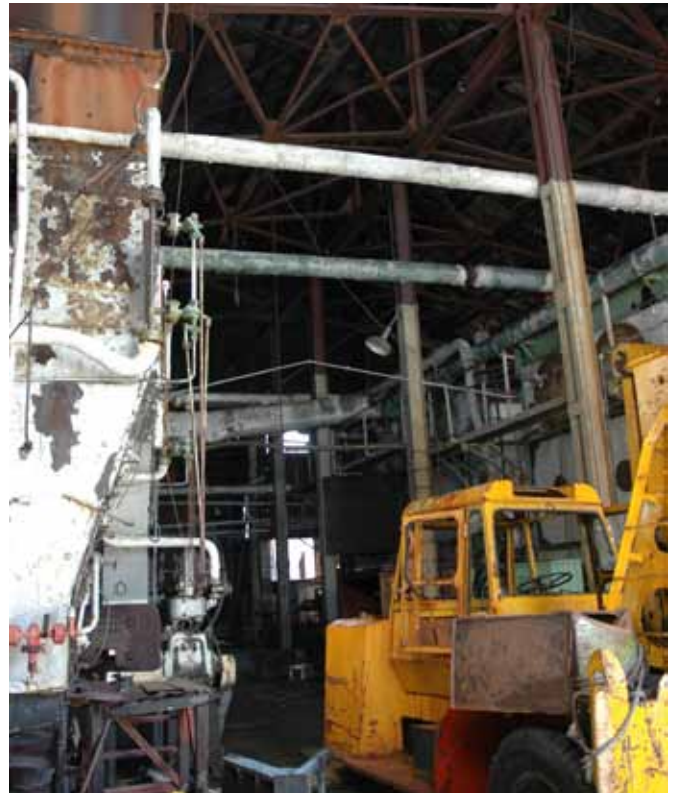
25.1 The interior looking southwards from the north doors
