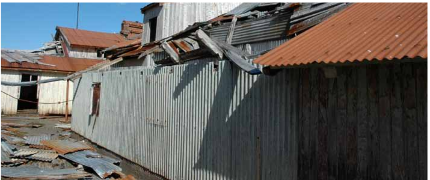
64.3 The north side of the building looking east
