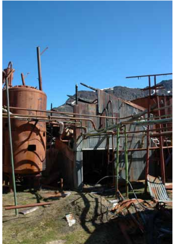
22.1 The north end of the building
