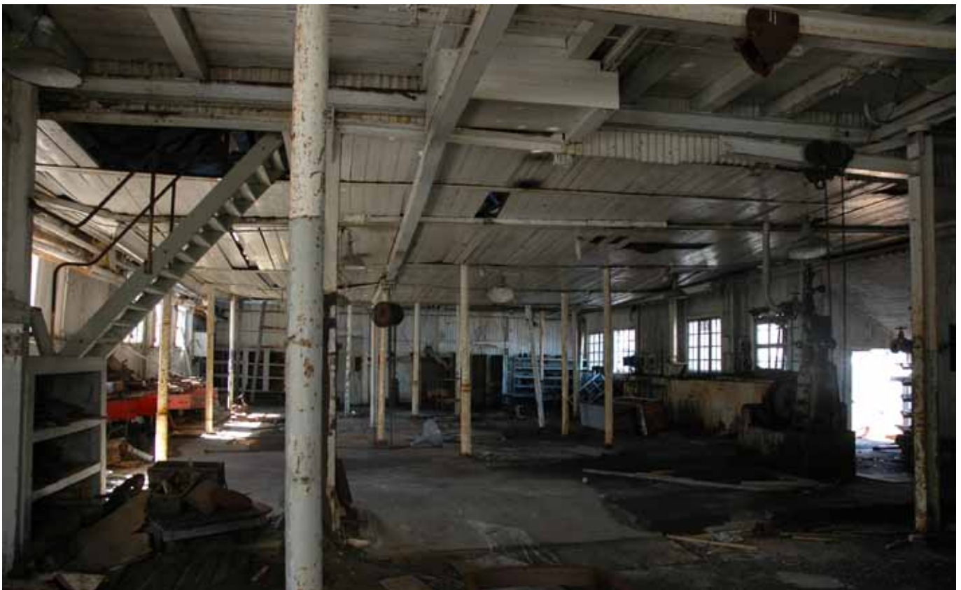
31.2 The interior of the south end of the building looking northwards
