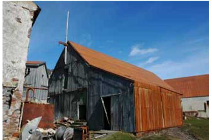
36.3 The east corner of the building
