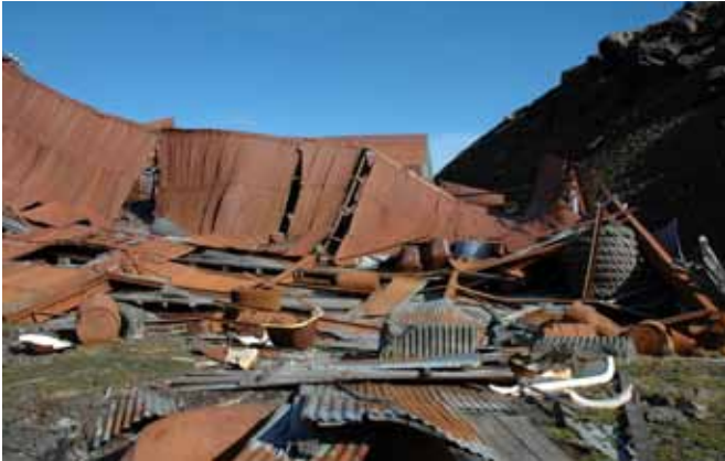
74.1 The north side of the building
