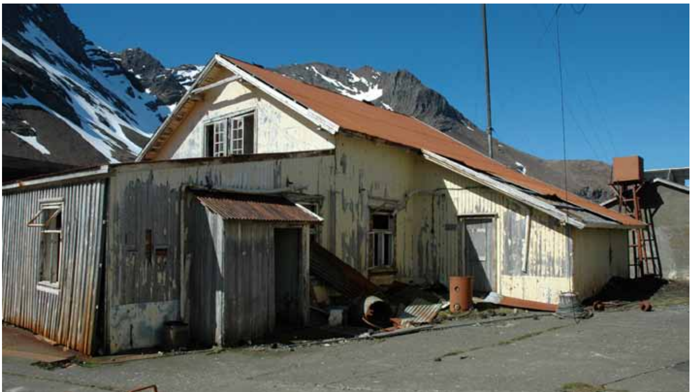
59.3 The southwest corner of the Manager's House
