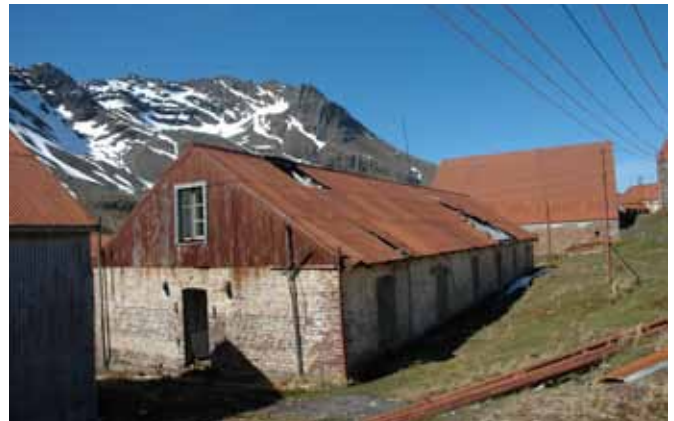
52.2 The northwest end of the D Barracks and southwest elevation
