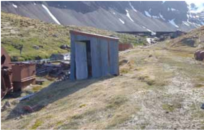
97.2 The north side of the building
