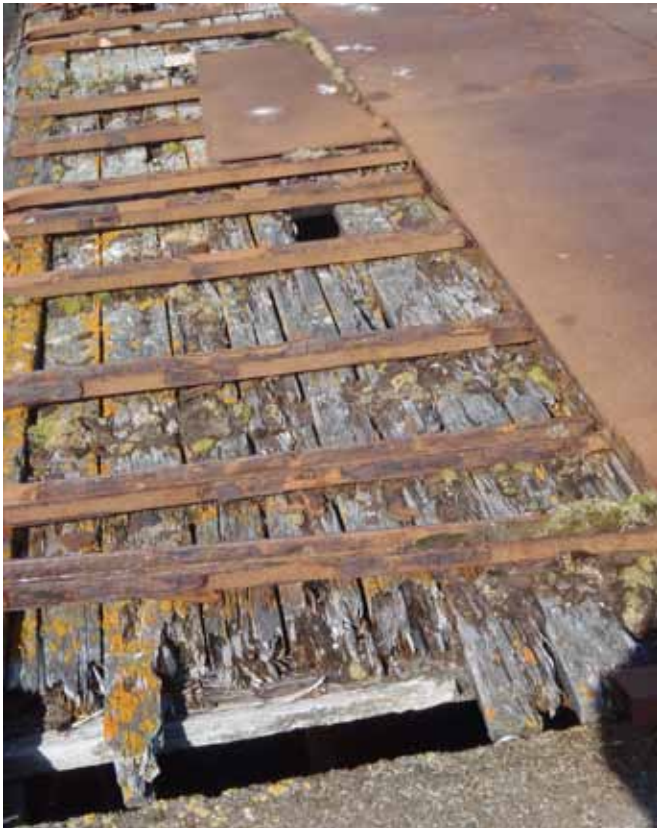
84.1 General condition of the deck
