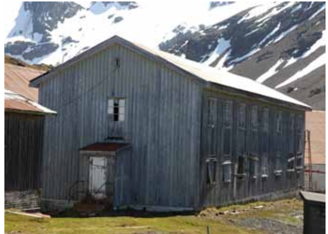
49.1 South and east elevations
