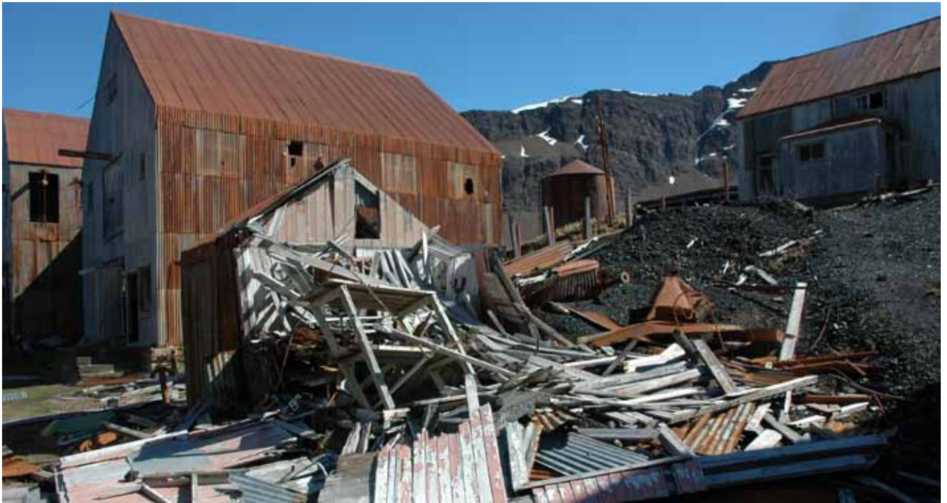
29.1 Looking southwards with the Catcher Store (No. 28) in the background
