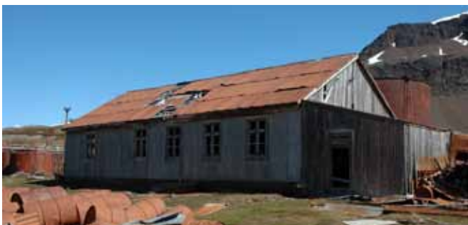
20.4 The east elevation with the northern lean-to from the switch room
