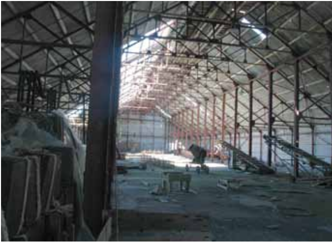
10.3 Interior of the main store shed looking eastwards
