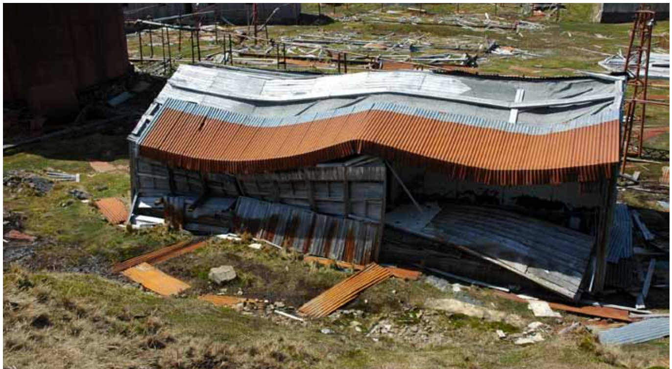
46.4 The west side of the Welfare Hut
