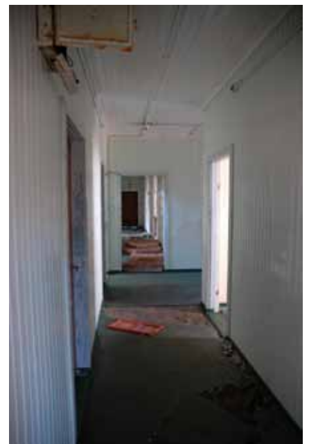
51.5 Ground floor central corridor looking northeast
