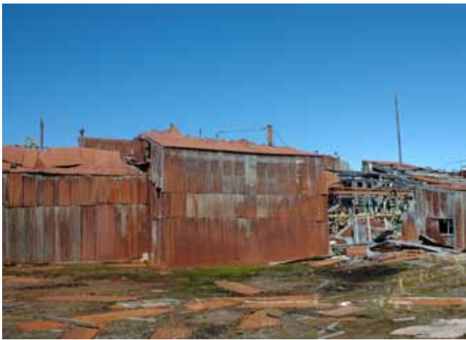
22.2 The west side of the Separator House looking southwest
