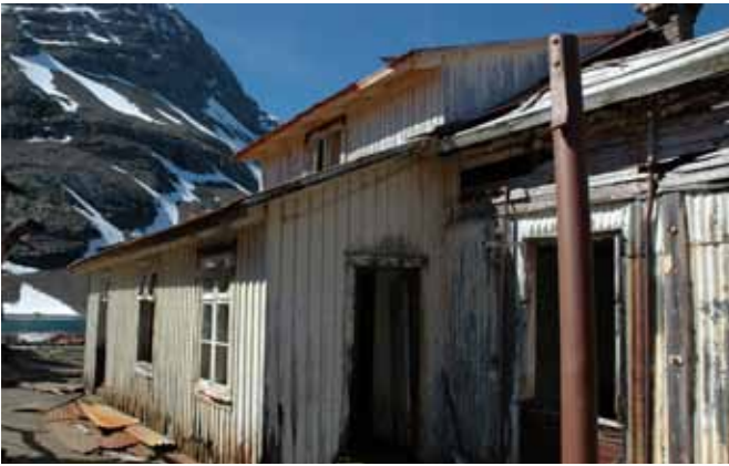
53.4 The northwest elevation of the northeast wing
