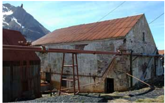
35.2 The north and west elevations
