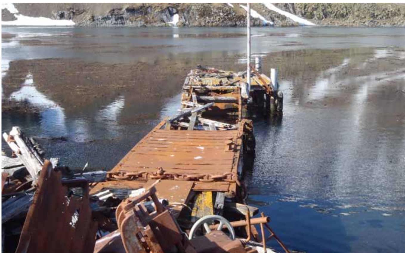
85.2 View along the Pier looking eastwards
