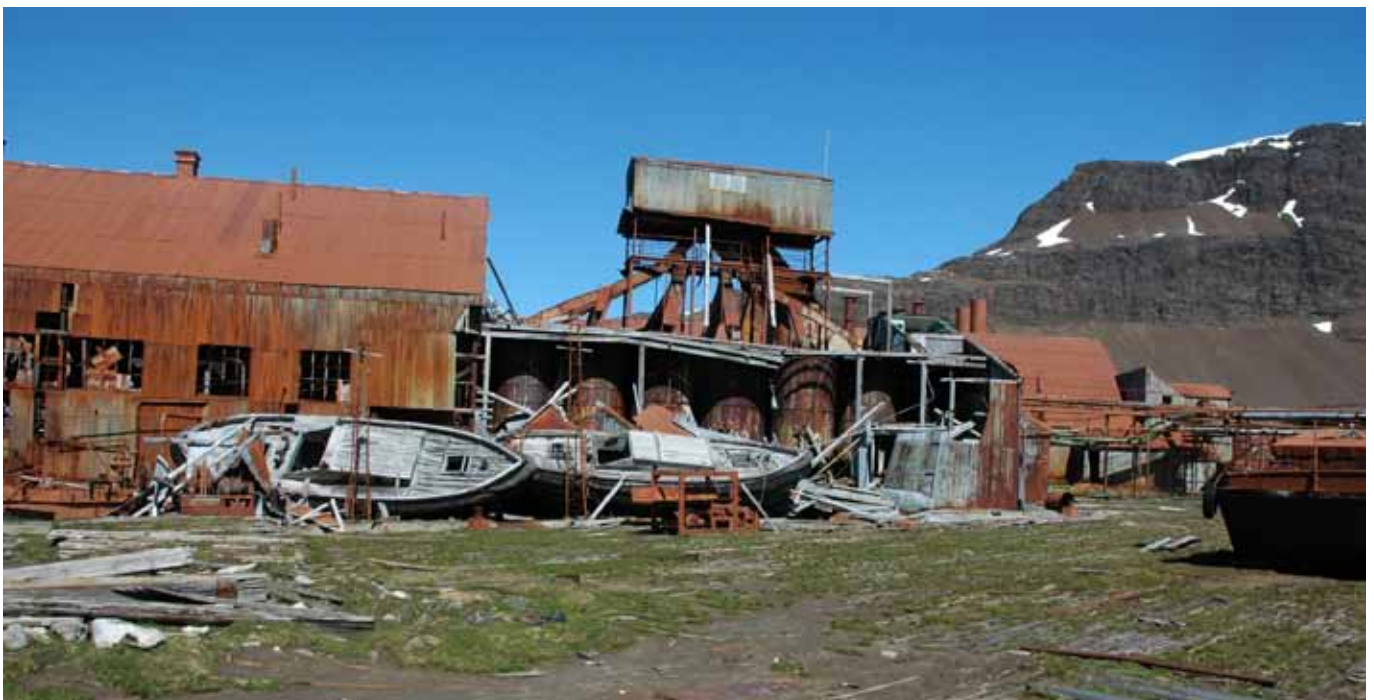
1.3 General view looking south towards the Blubber Cookery
