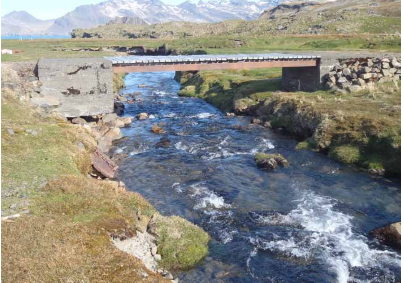
93.1 The Bridge seen from the west
