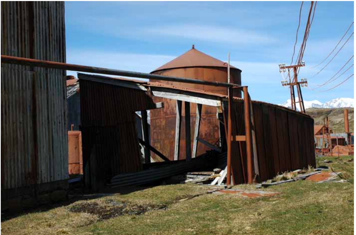
42.2 The north and west elevations
