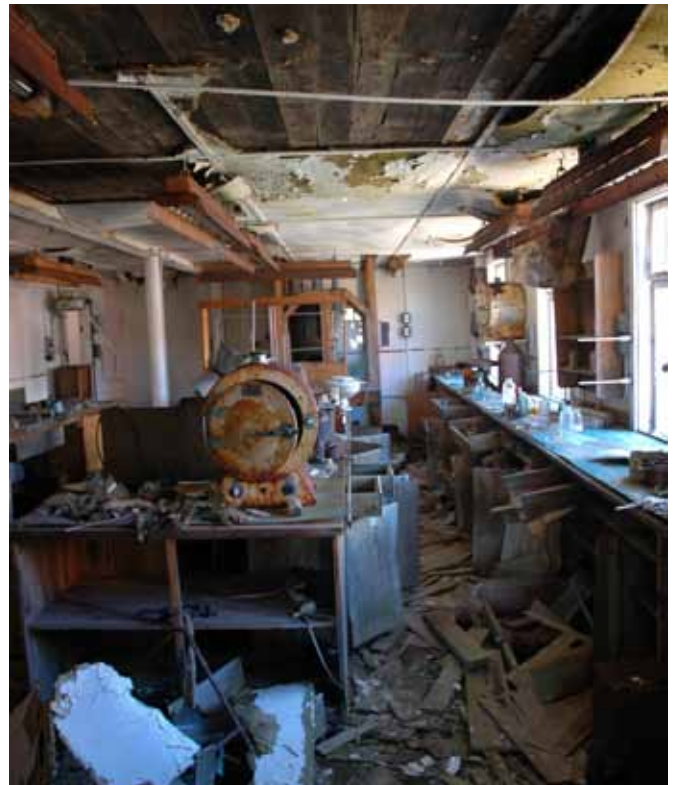
20.5 The interior of the Main Laboratory
