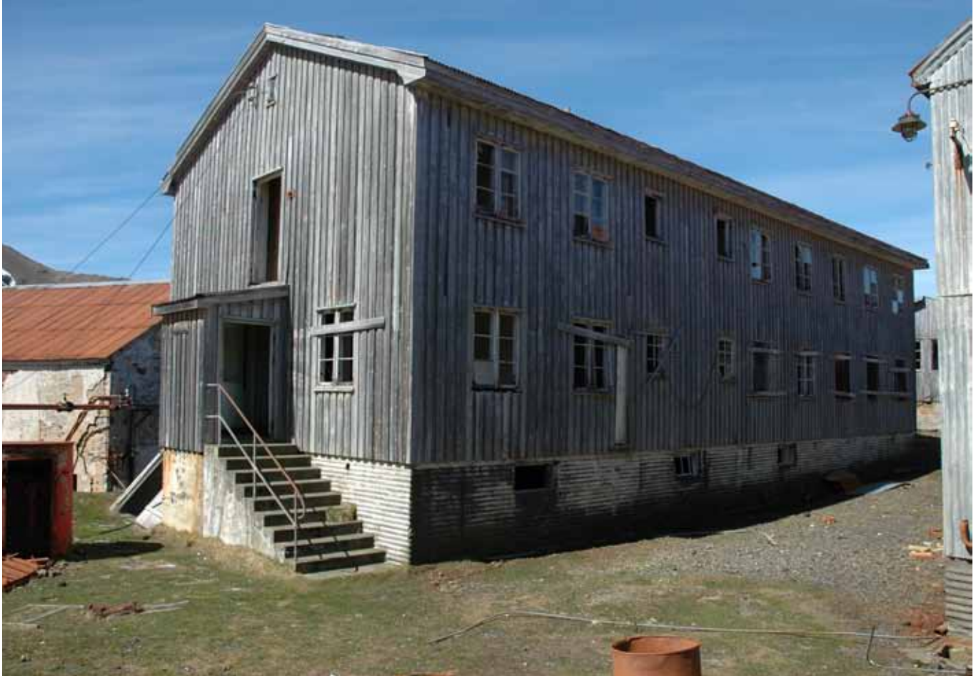
49.2 North and west elevations
