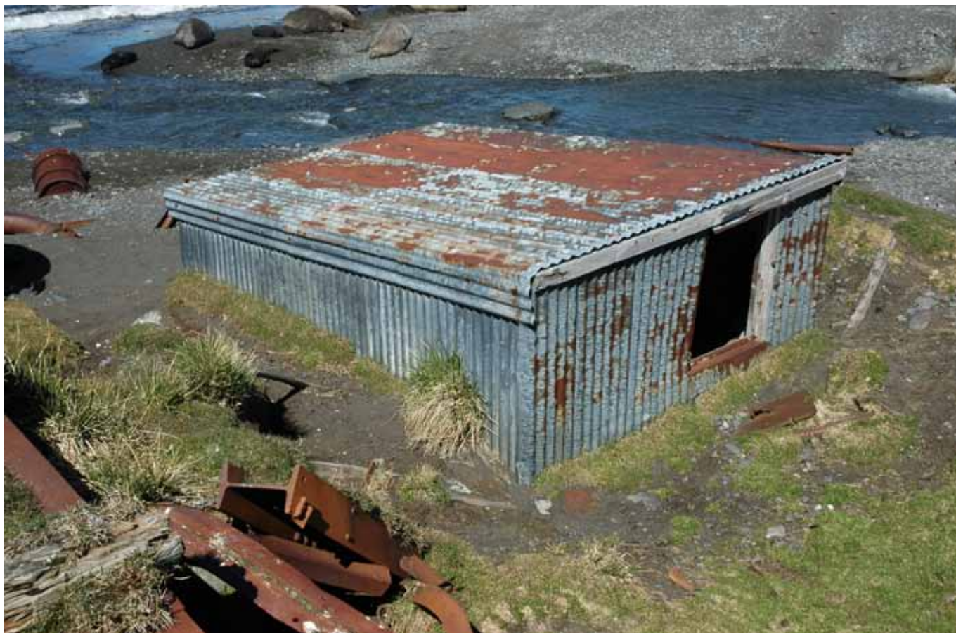
11.1 The Valve House looking southeast (ie., north and west elevations)
