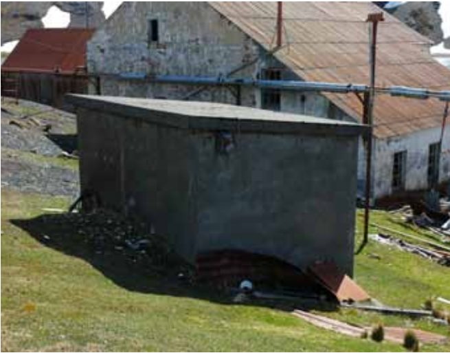
14.1 The northwest elevation
