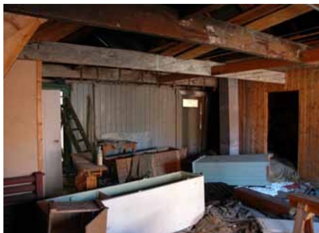
65.3 First floor drying room and bedrooms
