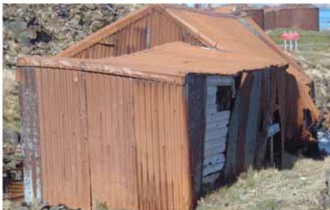
96.1 The west and south sides of the Valve House
