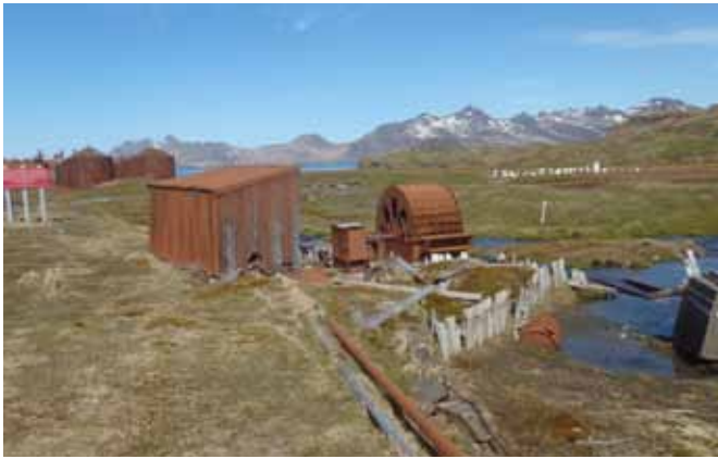
97.1 The west and south sides of the building
