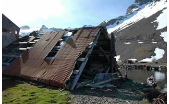
73.2 The east end of the roof
