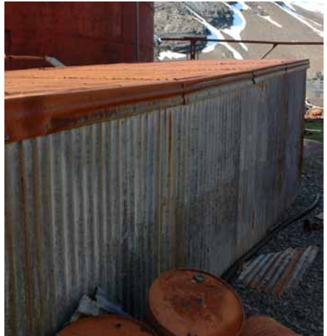
70.1 The south wall of the Hose Store looking eastwards
