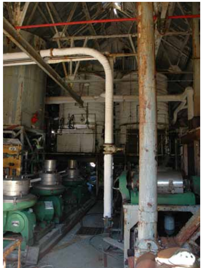
12.3 Interior of the building
