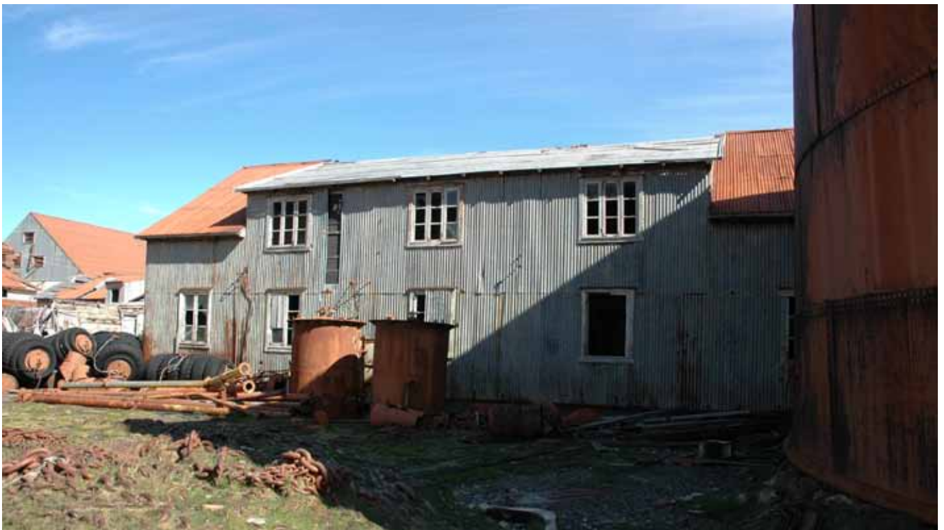
63.3 The east end of the north elevation
