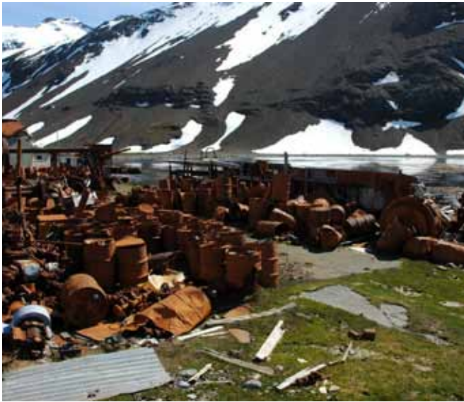
37.1 The whole building and adjacent area is covered in the scrap metal assembled in 1982
