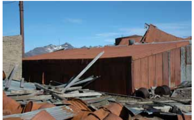
76.1 The north and west elevations
