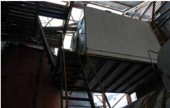
68.1 The steel stair and high level enclosed space
