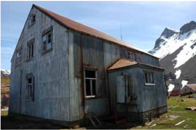
43.3 South and east elevations
