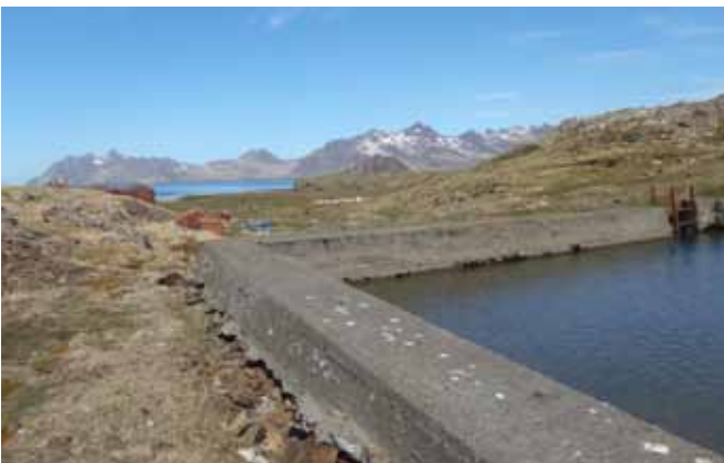
94.2 The Dam walls
