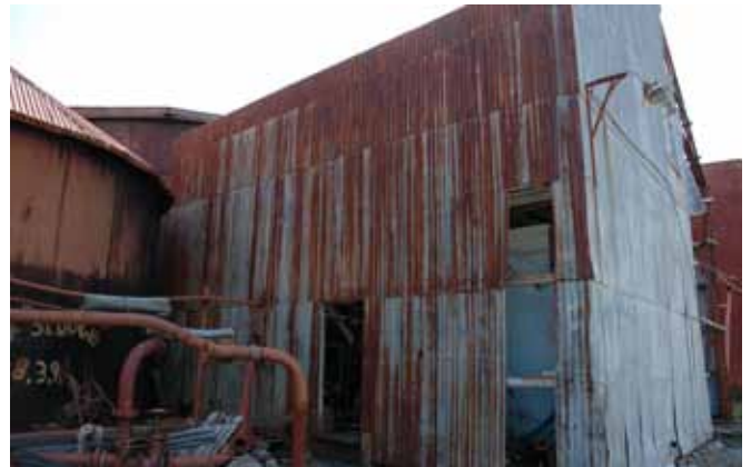
68.2 The southwest and southeast elevations
