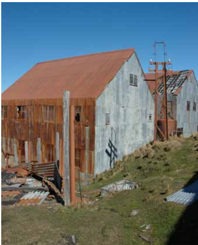
28.2 The north and west elevations
