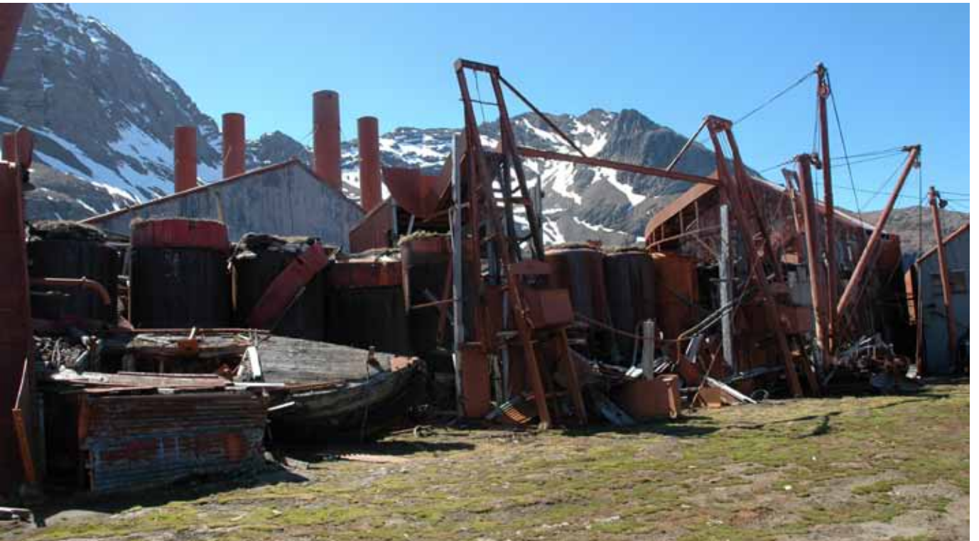
4.5 The west end of the south side of the building with the Boiler House in the background
