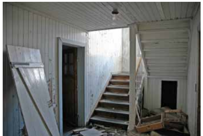
50.5 Staircase at the southern end of the Barracks
