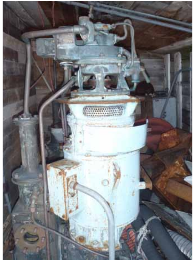
97.3 Interior and remaining pump
