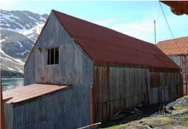
36.2 Southwest and northwest elevations
