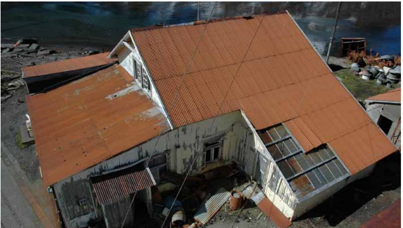
59.6 General view from the upper floor of Building No. 40
