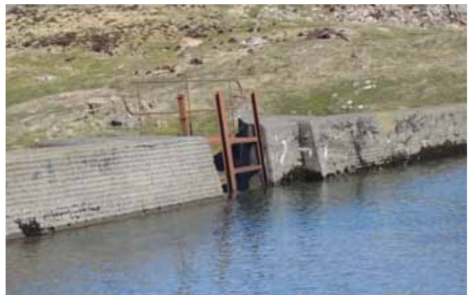
94.3 The overflow sluice
