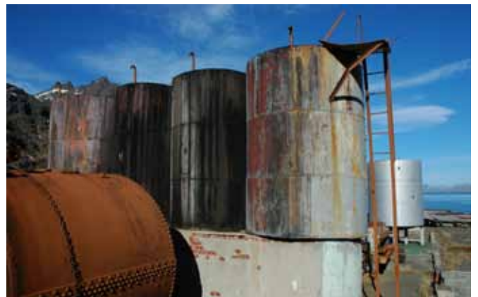
3.10 Tanks at the east end of the Boiler House area
