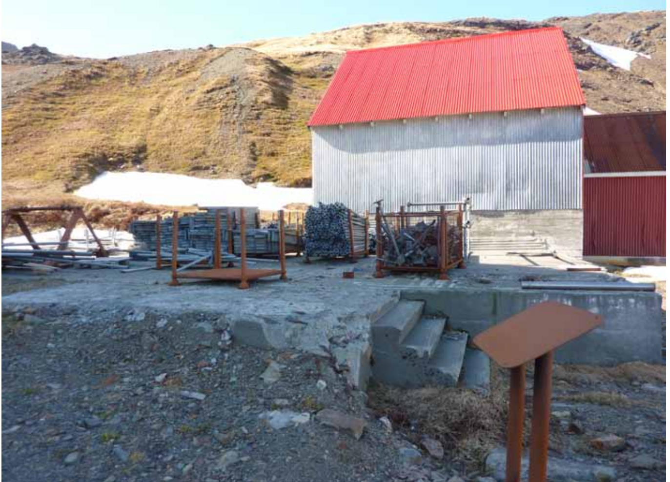
40.1 The base of the Provisions Store in the foreground with the Slop Chest (Building No. 46) in the background
