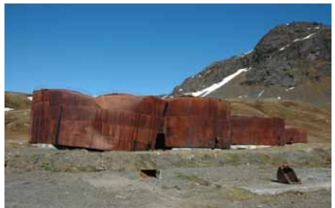
78.3 General view of the north side of the Tanks
