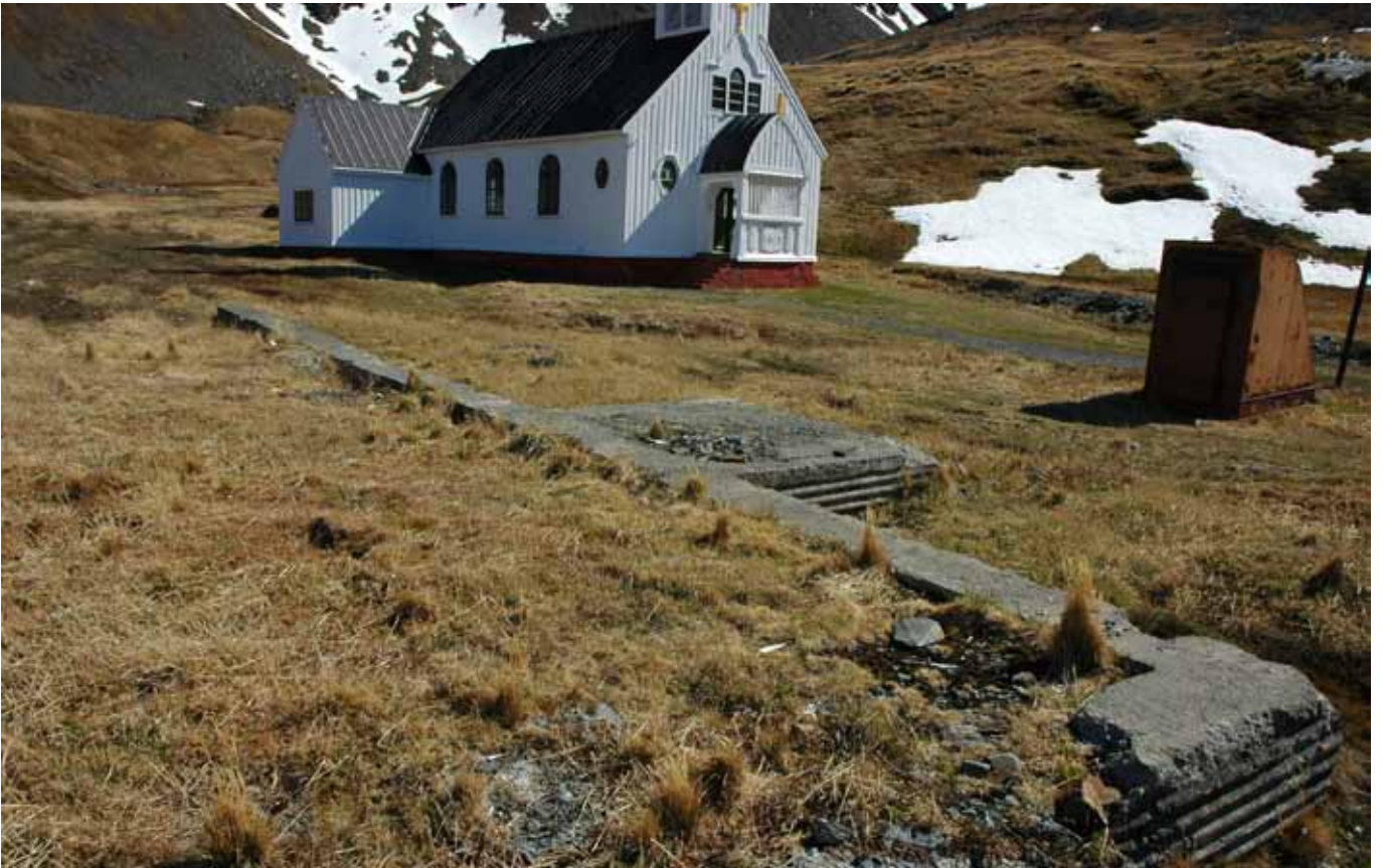
33.2 The remaining concrete base of the Cinema looking northwest
