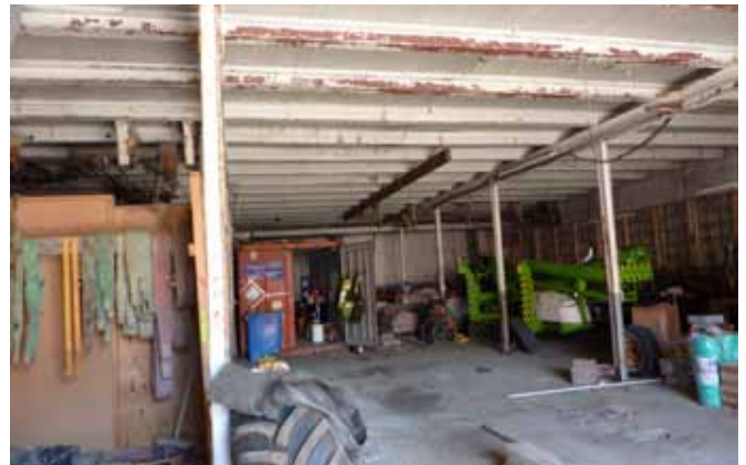
11.2 Interior ground floor of the main space now used for garaging
