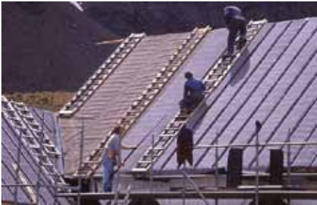
Roofing ladders made on site.
