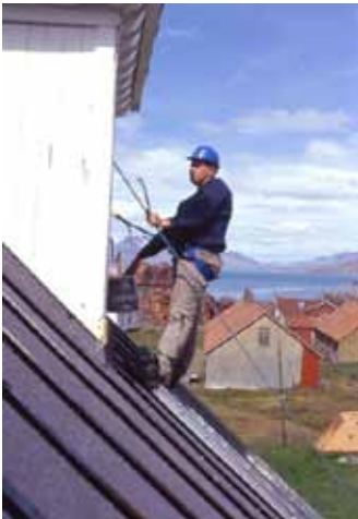
Dave paints the steeple.
