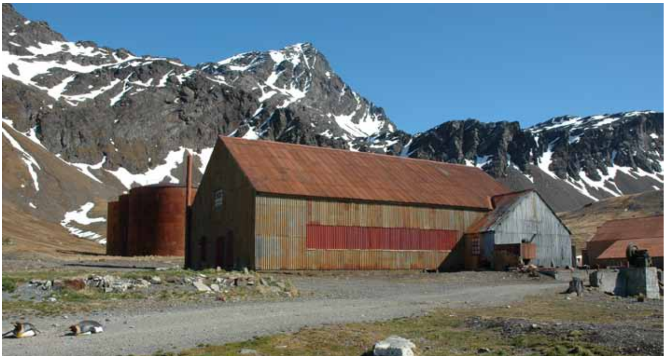
11.3 South and east elevations
