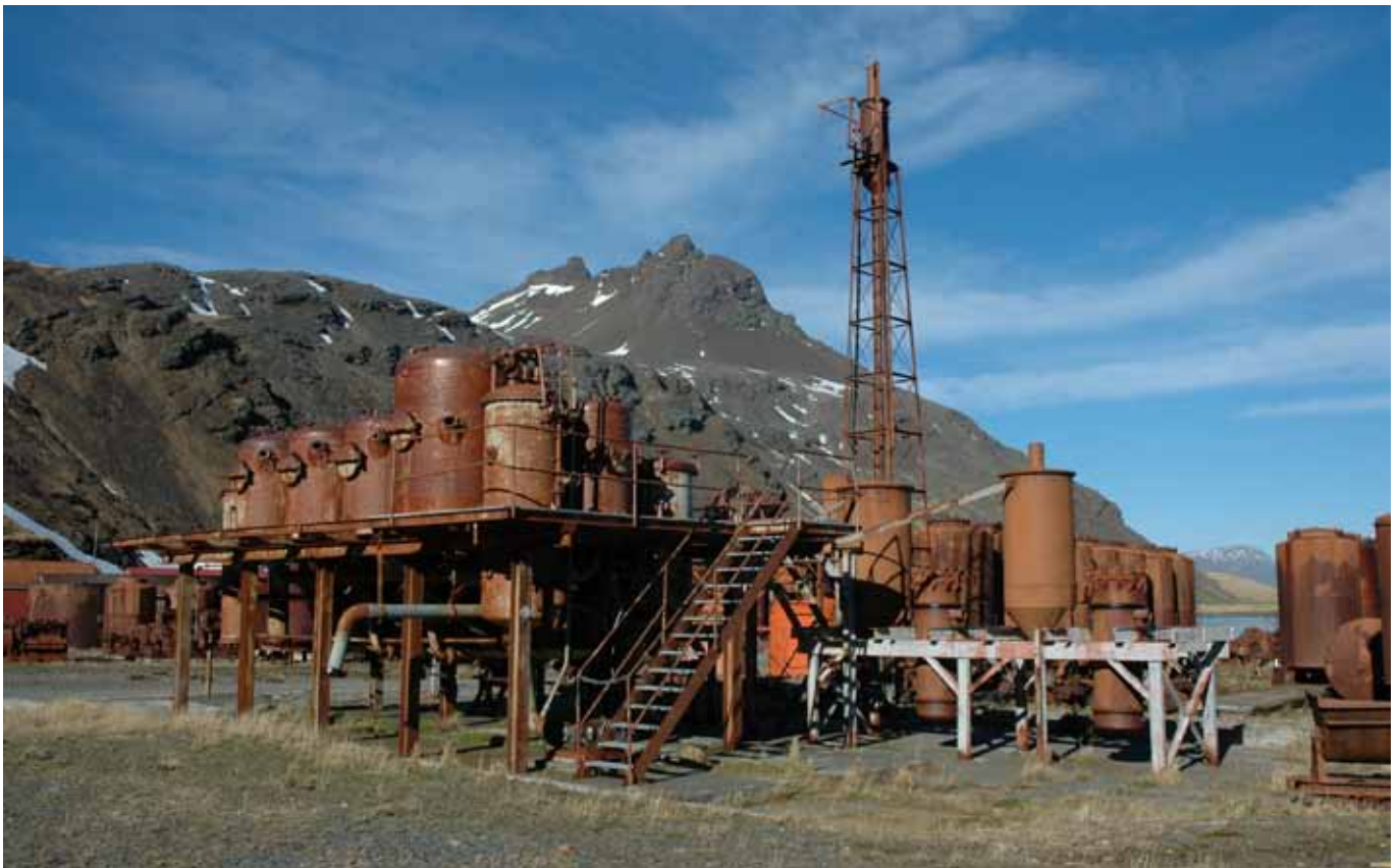
5.3 General view of the Glue Water Plant looking northeast
