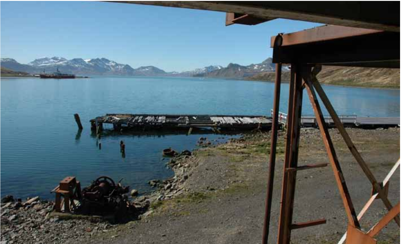
59.2 The north end of the Jetty
