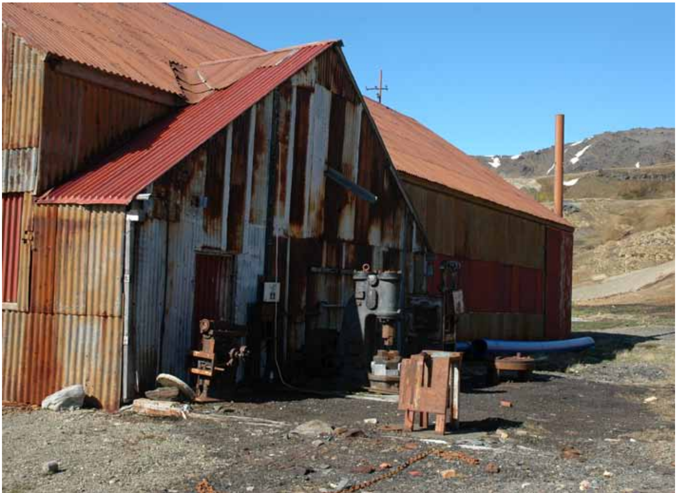
11.4 West elevation showing the location of the demolished Workshop
