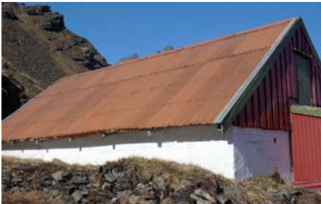
42.1 The west elevation partially below ground
