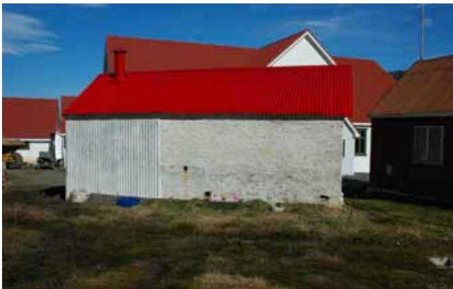
45.1 The northwest elevation
