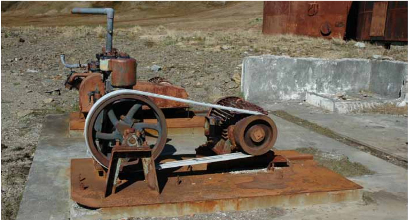
15.1 Remaining pump and motor
