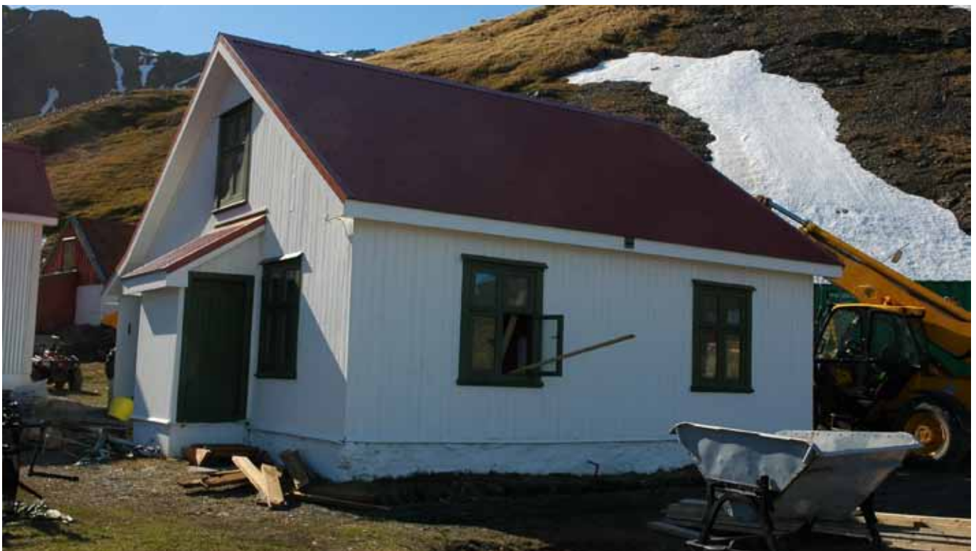
37.3 The south and east elevations
