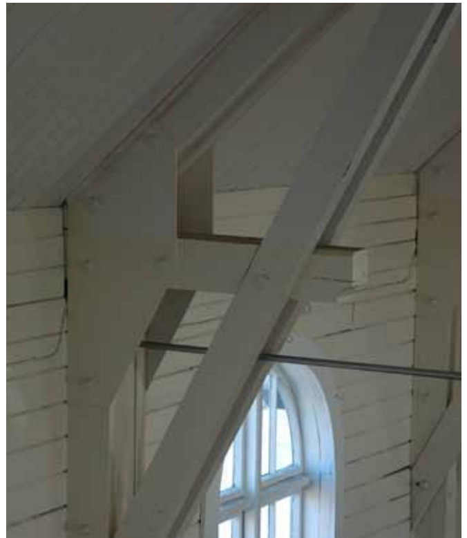
34.19 Steel plates installed to strengthen the roof trusses
