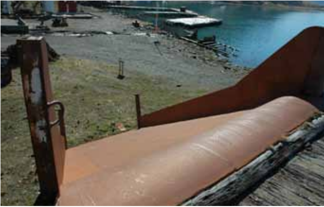
2.9 Steel ramp up to the meat cooker platform
