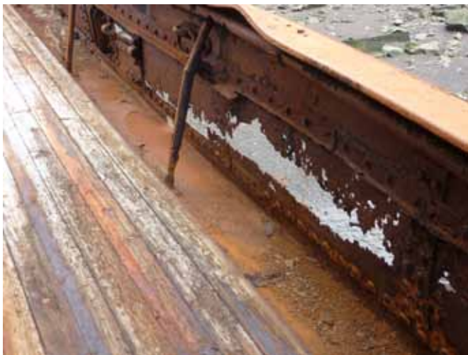
52.4 The corrosion of the bulwarks of the Dias
