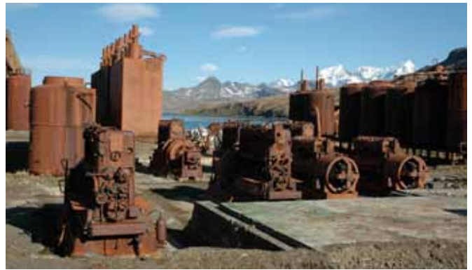
4.4 General view of the generator sets
