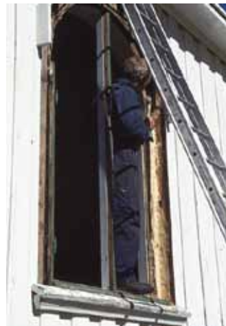
Tim cuts out rot from a window frame.
