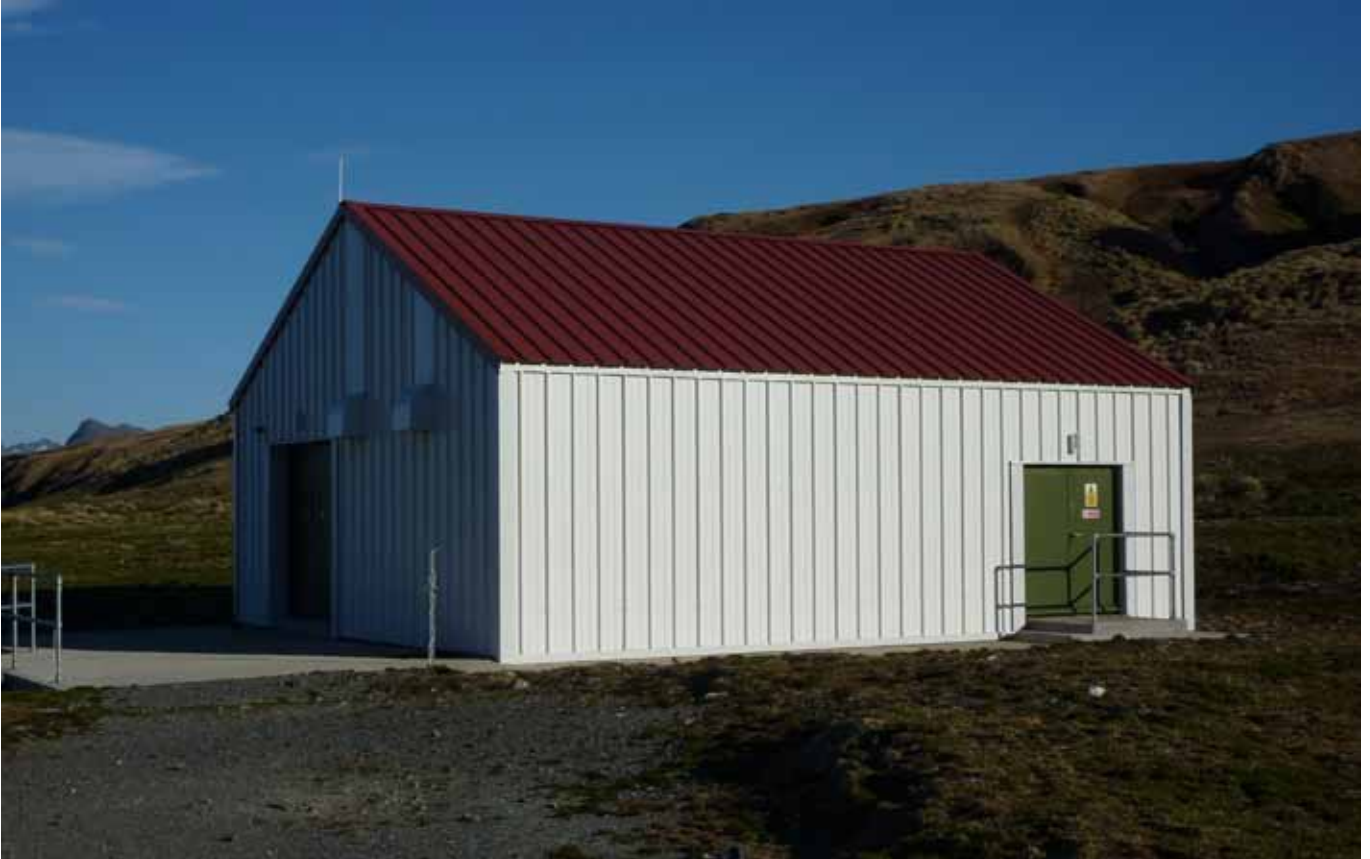
24.1 North and west elevations
