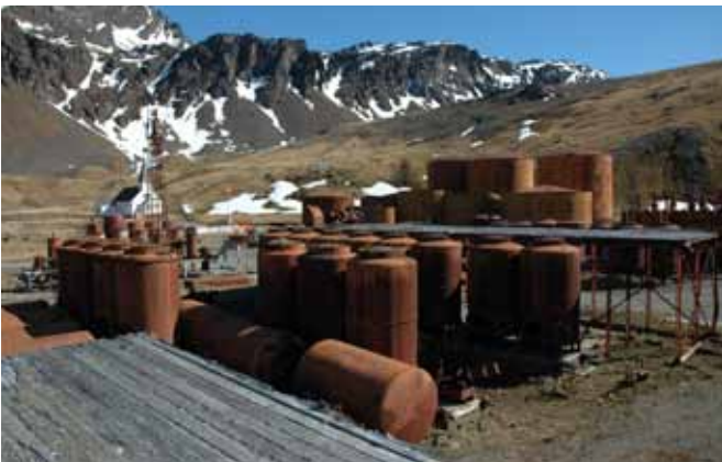
2.11 Remains of Bone Cookery seen from the platform over the Meat Cookery
