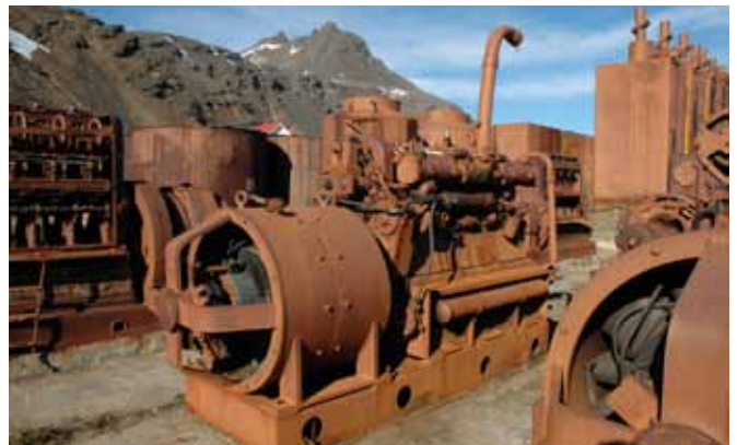
4.5 Detail of generator set
