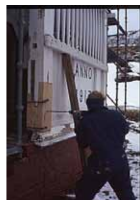
Tim repairs the porch
