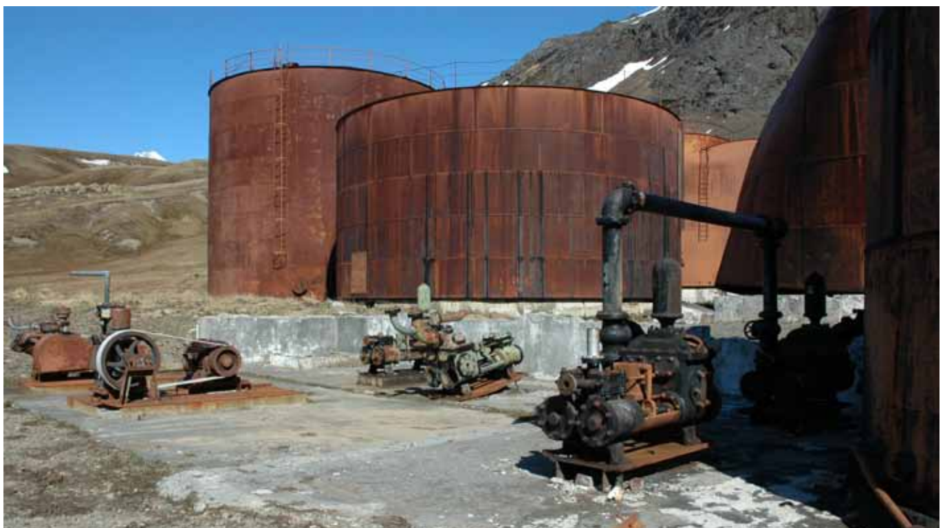
15.2 Site of the Pump House looking southwest with storage tanks behind
