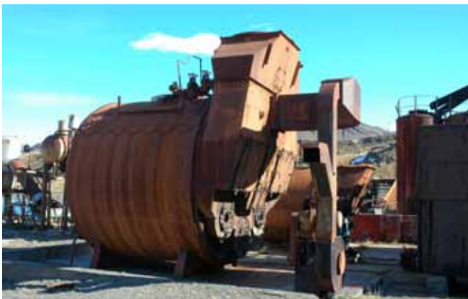
3.9 North side of second row of boilers
