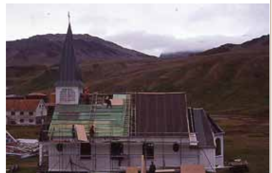
Felt laid at one end, plywood at the other.
