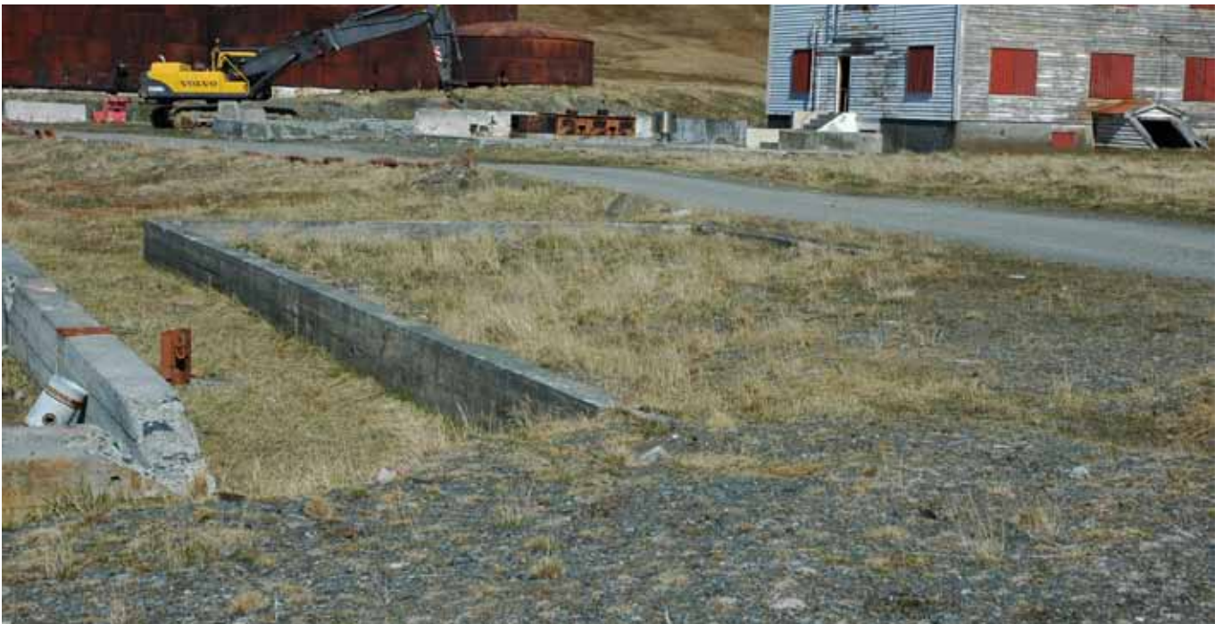
7.1 Foundation of the Building No. 7 Laboratory and Store
