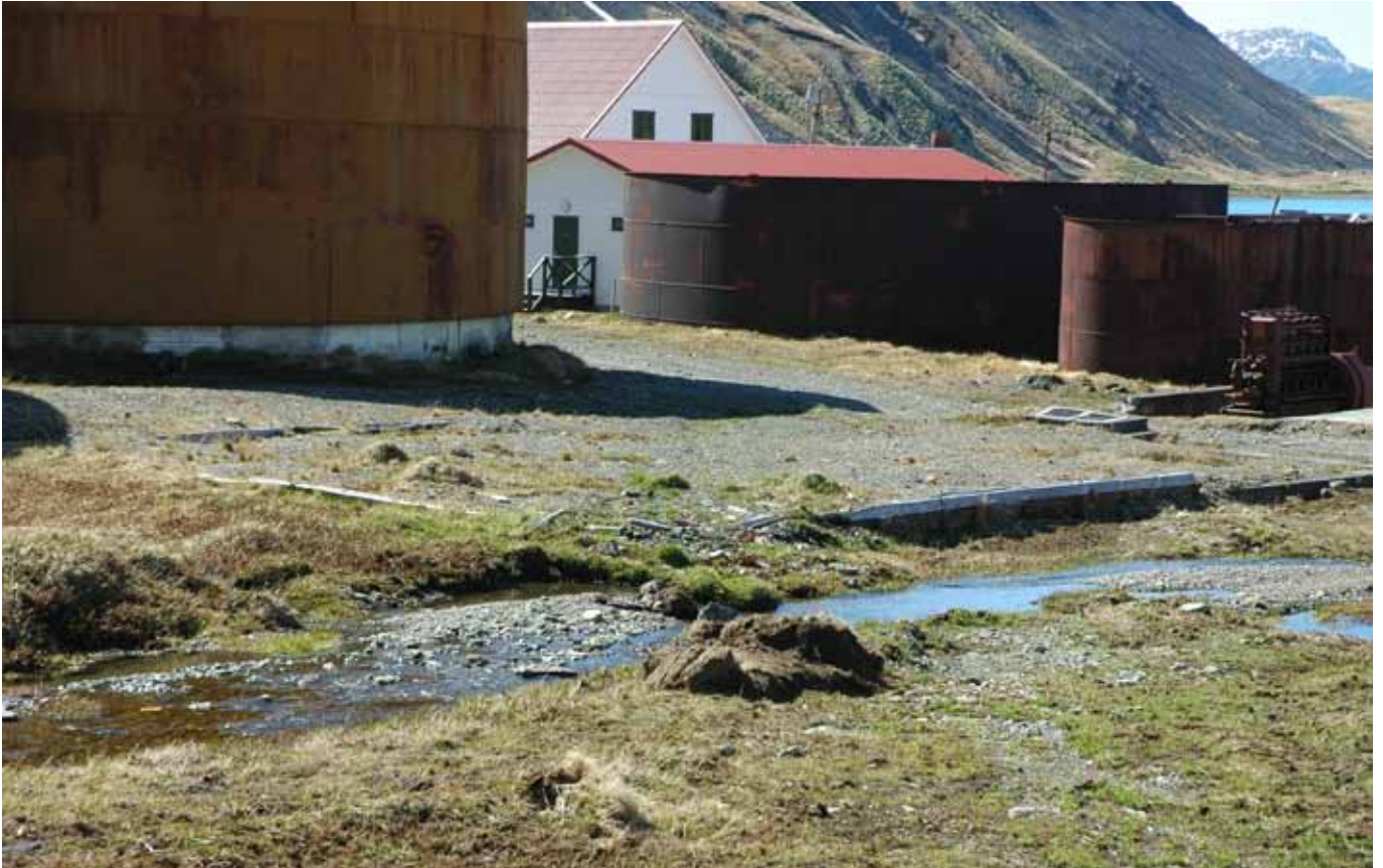
35.1 The remaining base of the Hospital looking northeast
