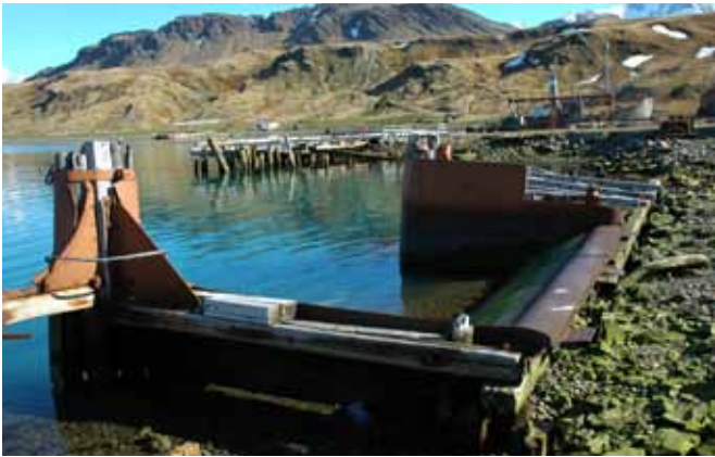
1.4 The slipway for hauling whales onto the Flensing Platform
