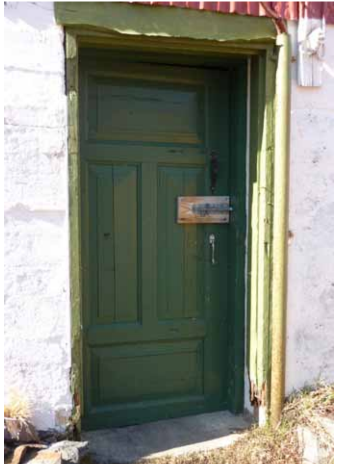
42.2 The door spoiled by the modern bolt and fixing block
