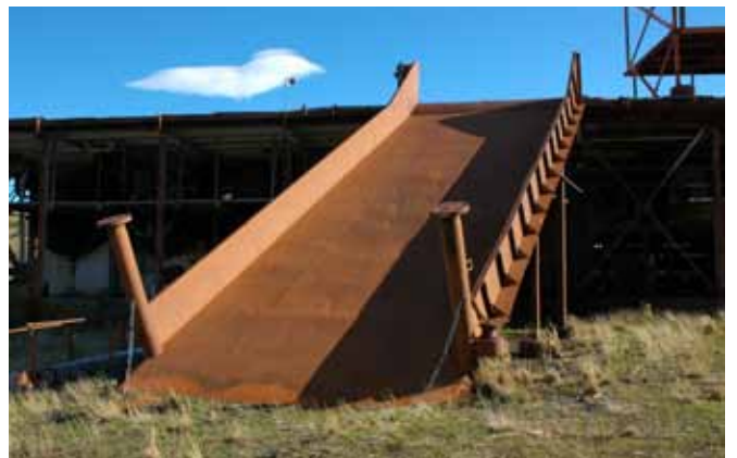
1.6 The steel ramp up to the platform over the Meat Cookery in Building No. 2
