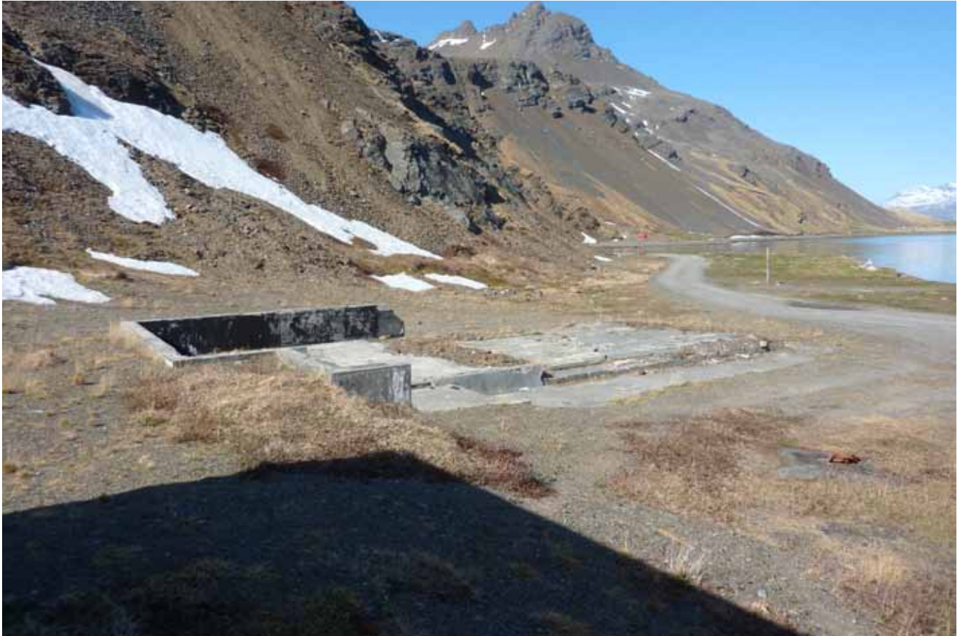
44.1 The remaining base of the Cold Store
