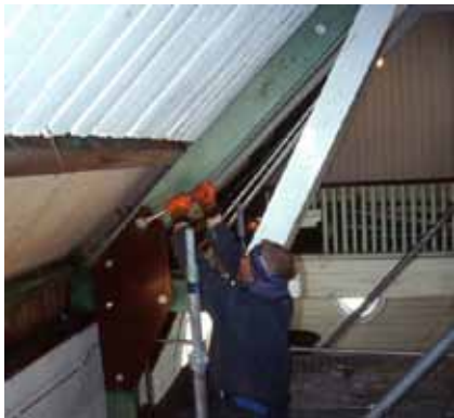
Tim bolts a plate to a roof truss.
