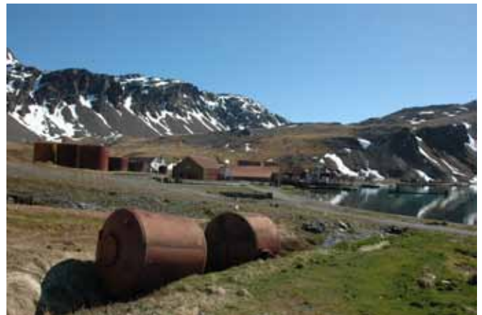
23.4 Fuel tanks tumbled into the stream bed below the site of the generator plant
