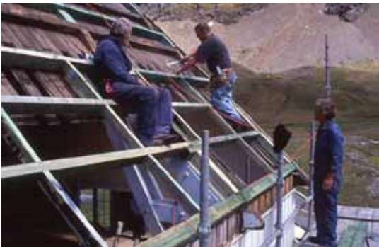
Sometimes the ceiling was removed. One works, two watch!
