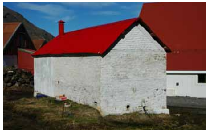
45.2 The west corner of the building
