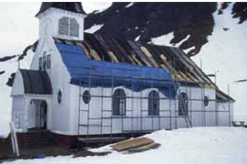
Temporary repairs after the 1994 storm.
