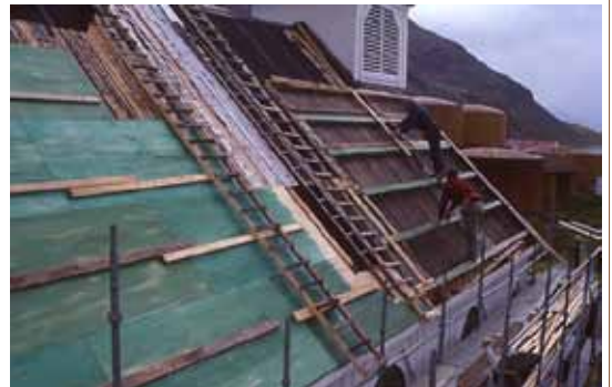
The board ceiling can be seen.
