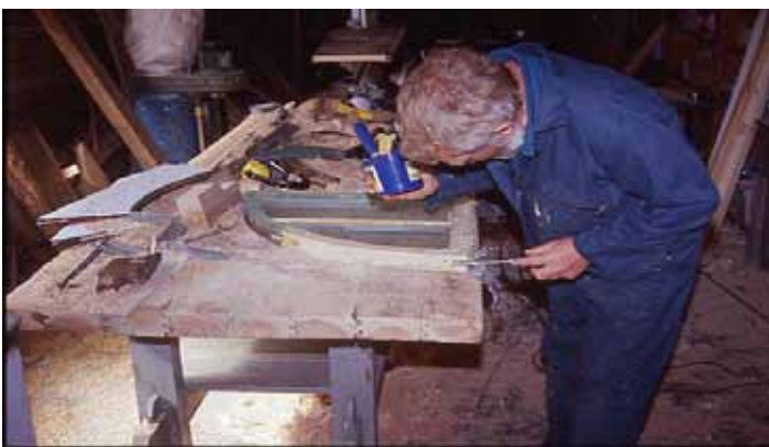
Tim rebuilds a rotten window frame.
