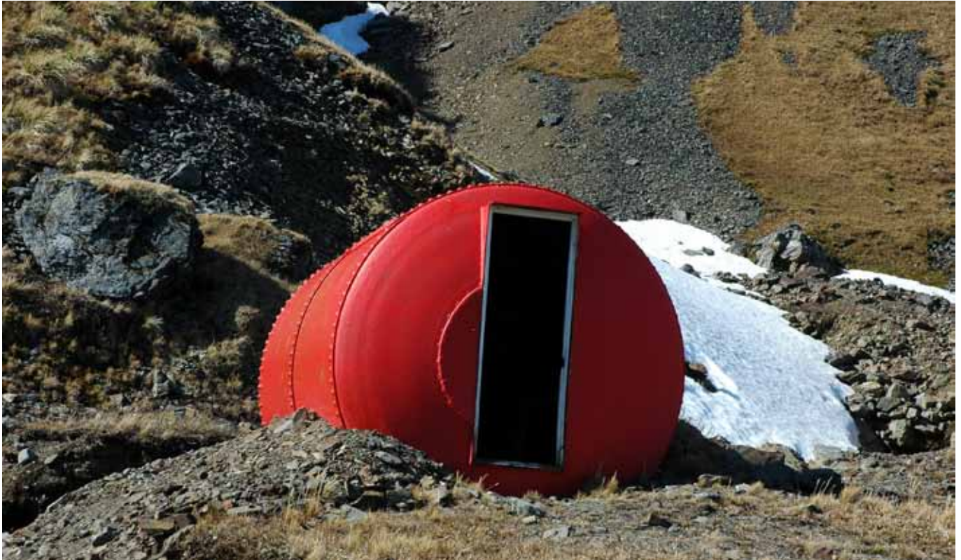
49.1 The store made from an old boiler
