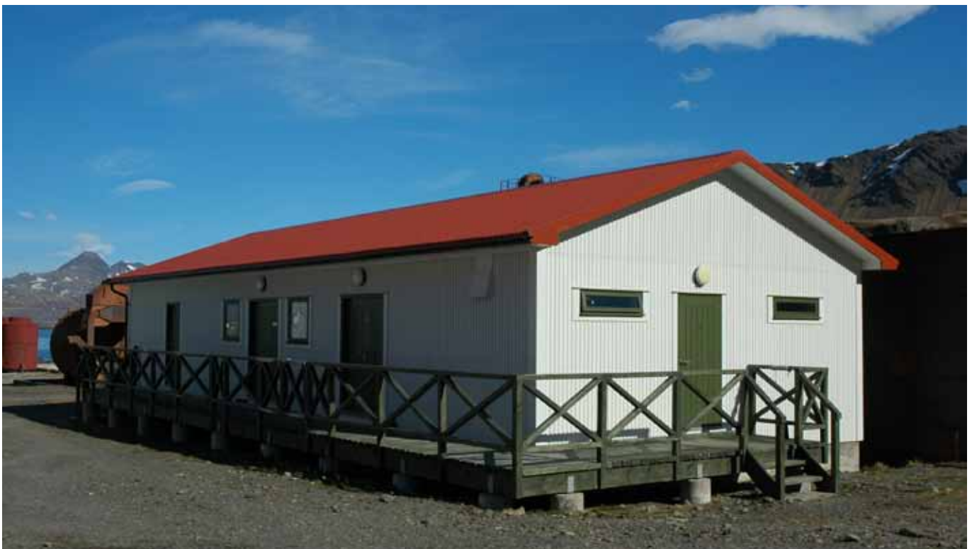
39.3 The north and west elevations
