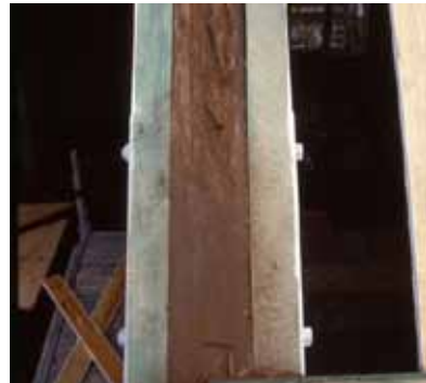
Original truss sandwiched between new timbers.
