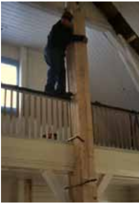
Tim strengthens the steeple pillars.
