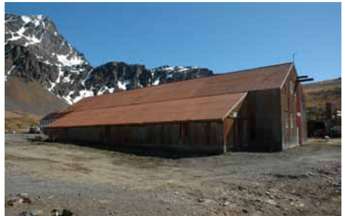
10.2 South and east elevations
