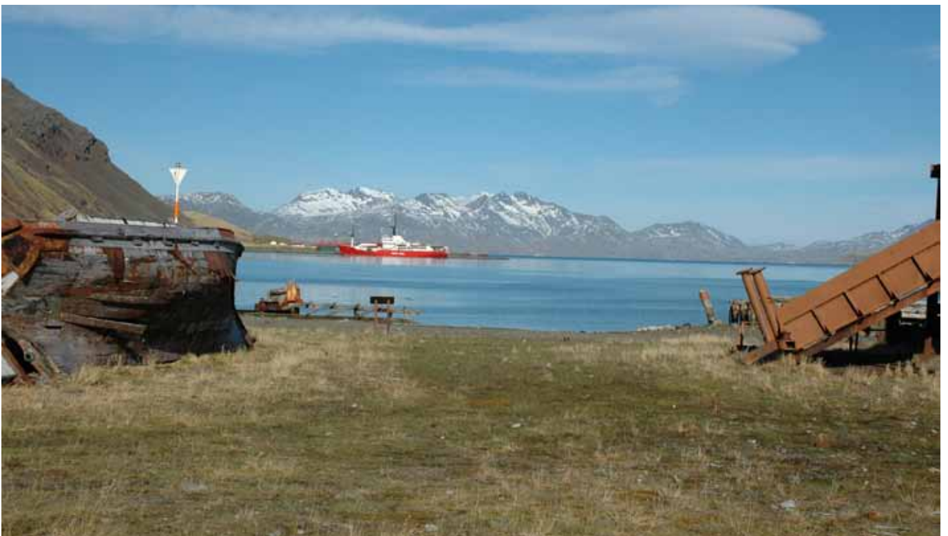
1.7 General view of the Flensing Platform looking east
