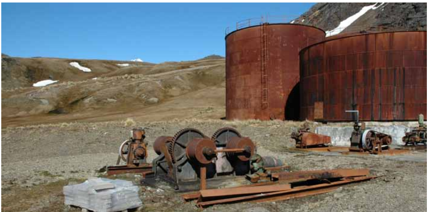
14.2 The site of the Winch House looking southwest with the Pump House behind
