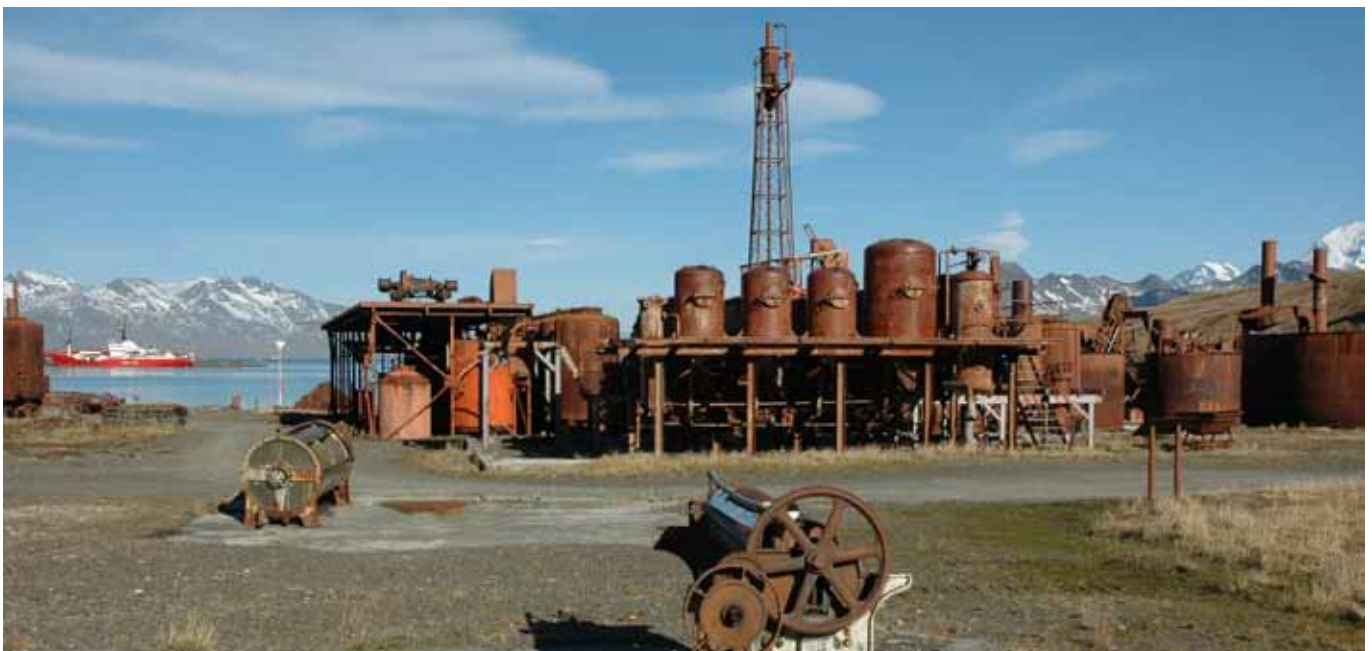
31.1 The remnants of the Russebrakka Barracks looking eastwards with the Glue Water Plant (No. 4) in the background
