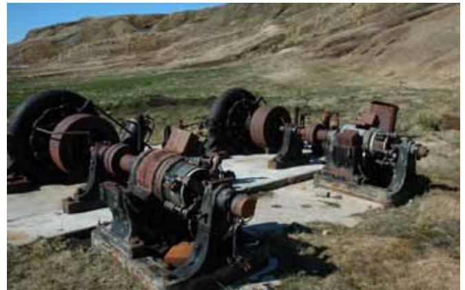
23.2 Hydro electric sets
