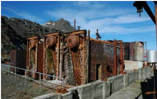
3.3 Southwest corner of the boilers
