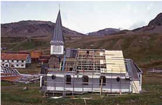
Laying plywood.
