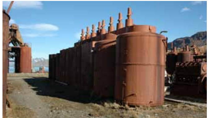
4.3 Cylindrical tanks to south of the building
