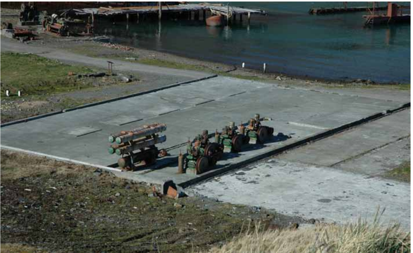
21.3 Detail of remaining Chiller Plant
