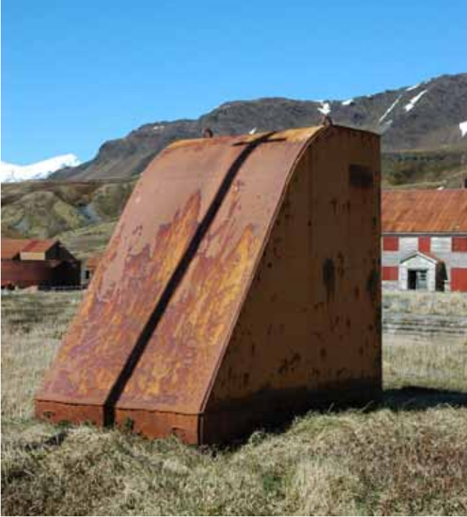
33.1 A metal covering to an underground chamber adjacent to the Cinema
