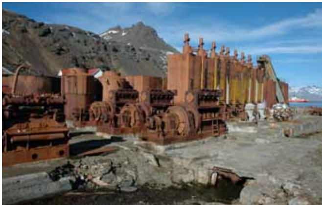
4.1 General view of Separator and Power Plant looking northeast
