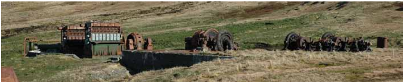
23.5 Remaining concrete floor of the hydro power plant looking south
