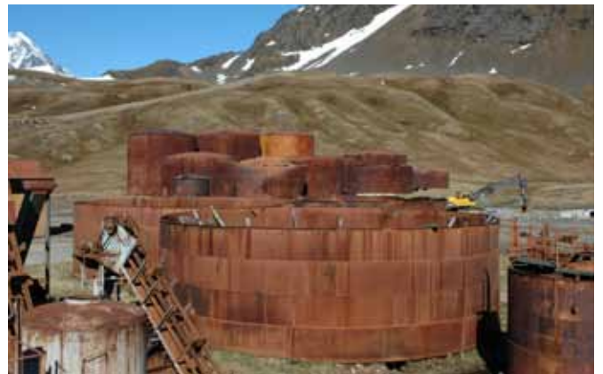
2.18 The storage tanks enclosed by the northwest arm of Building No. 2 and the Bone Cookery
