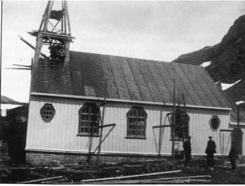
Building the steeple 1913.
