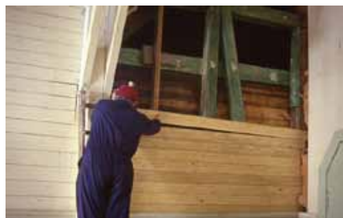
Dennis rebuilds the badly-rotten corner.
