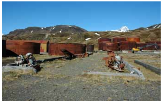
2.19 The remaining outline of the northwest wing of Building No. 2 looking southwards
