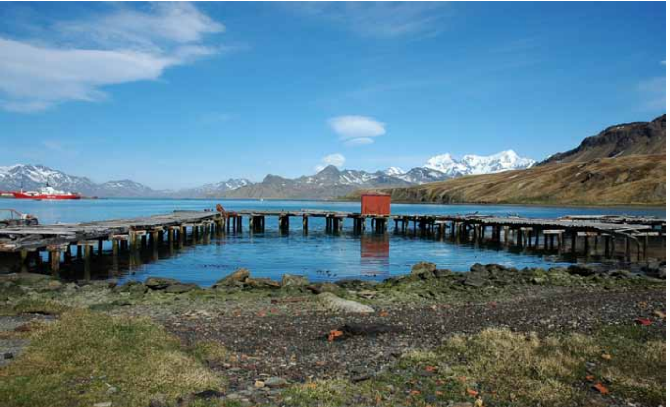
58.3 General view of the Harpoon Jetty
