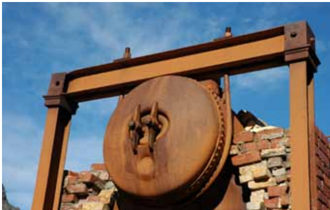
3.4 Detail of top of boilers showing very loose brickwork
