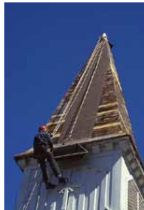
Tim repairs the steeple. New timbers and the plywood apex are in place and felt is being laid.
