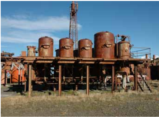
5.1 West side of Glue Water Plant
