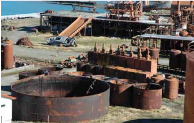
1.3 General view looking southeast
