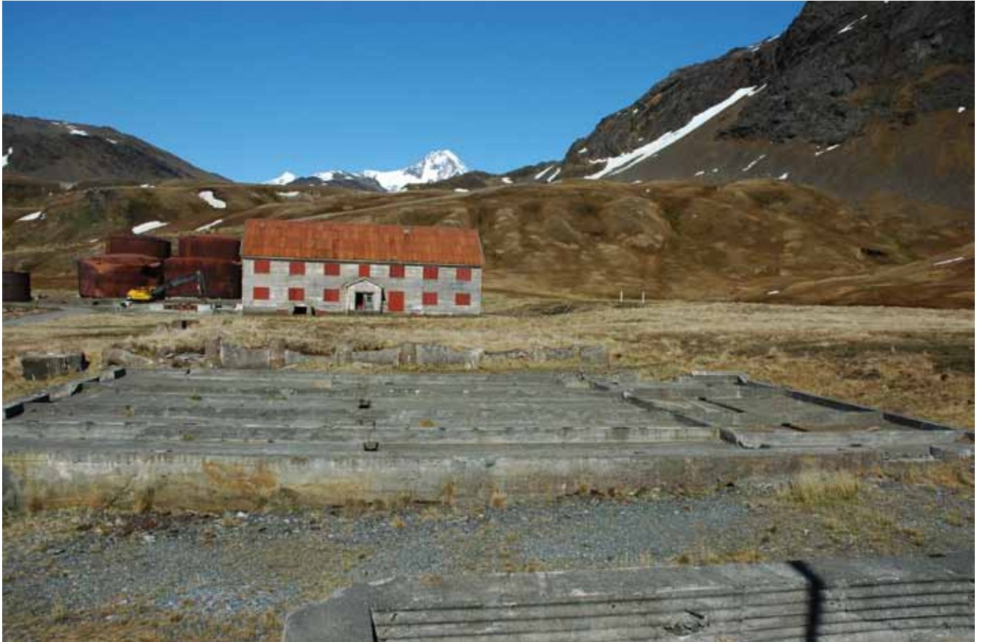
32.1 The concrete base of the Bath House in the foreground looking south to the Nybrakka
