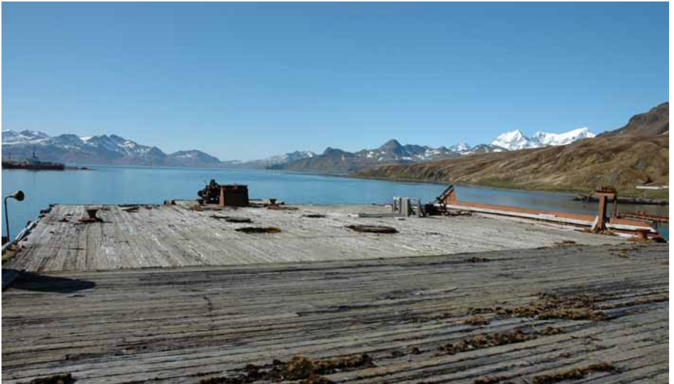
2.15 General view of the platform over Meat Cookery looking east
