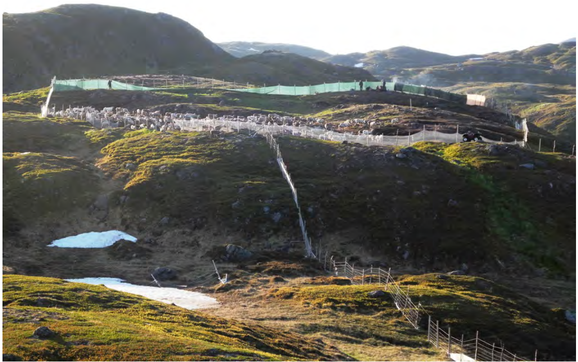
Figure 6. Initial enclosure and lead fence system. (Henrik Eira)
