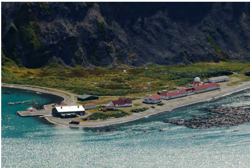
Figure 3. Existing KEP station and wharf (Alastair Wilson, BAS)
