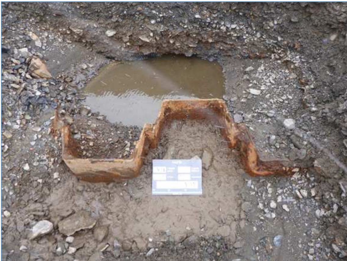
View on sheet piles to anchor wall
