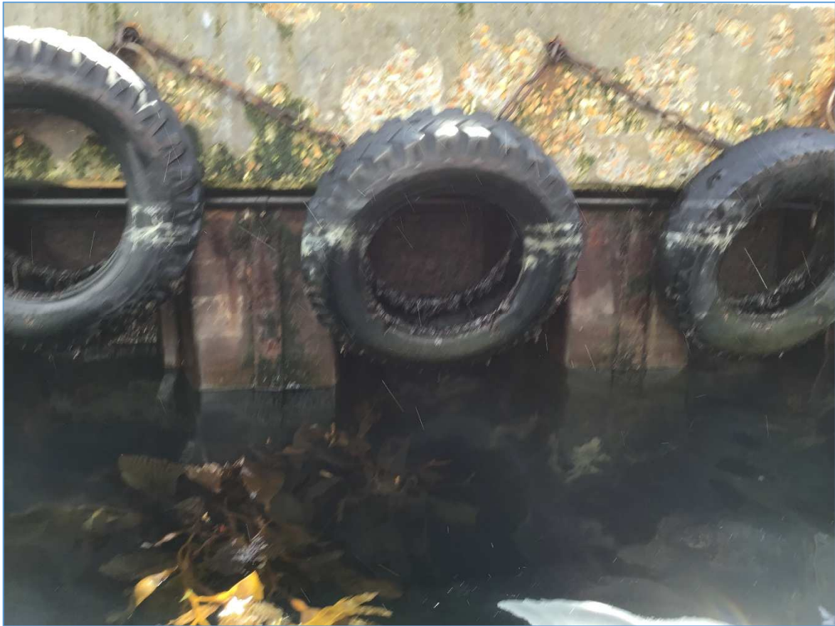
Close up view on west section of south wall
