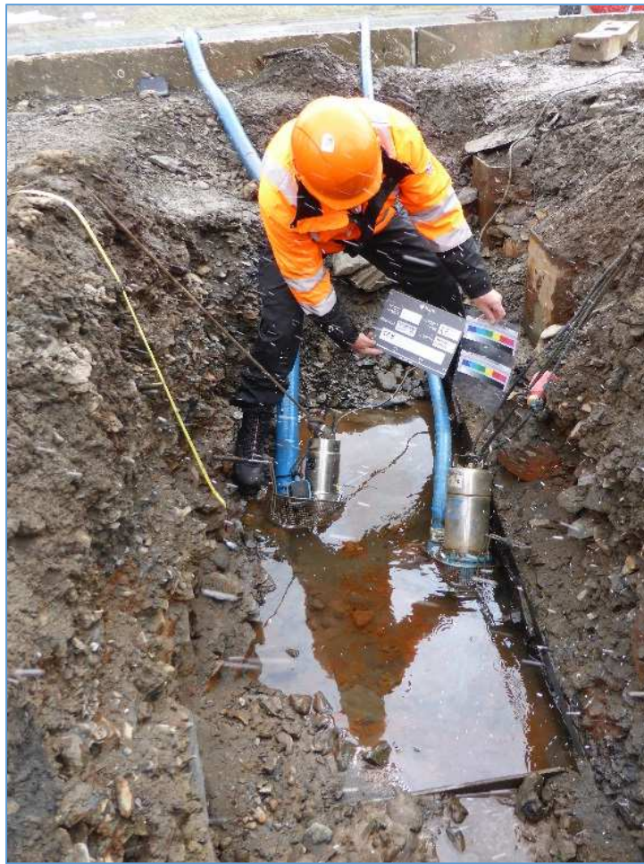
View along trial pit
