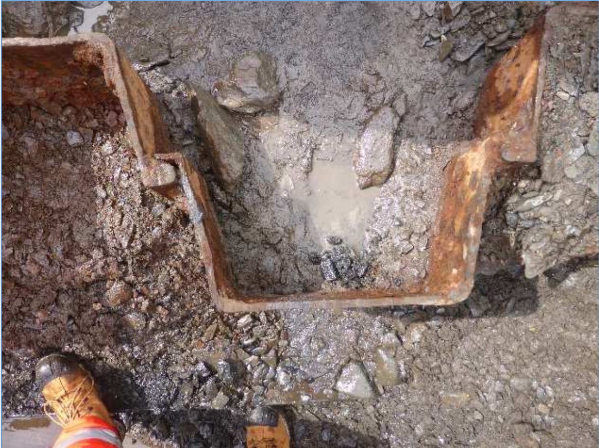
View on sheet piles to anchor wall
