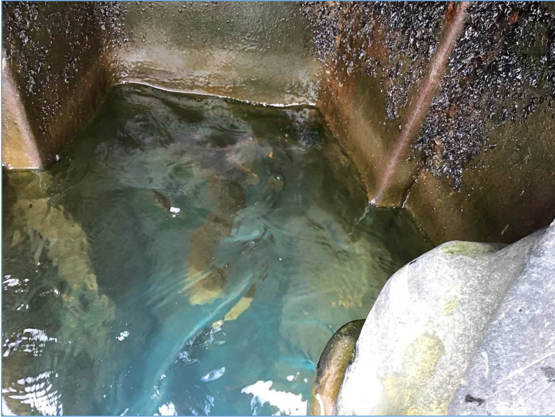
End view on sheet pile and tie rod
