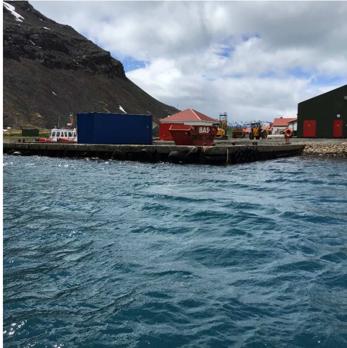
View on south and west walls
