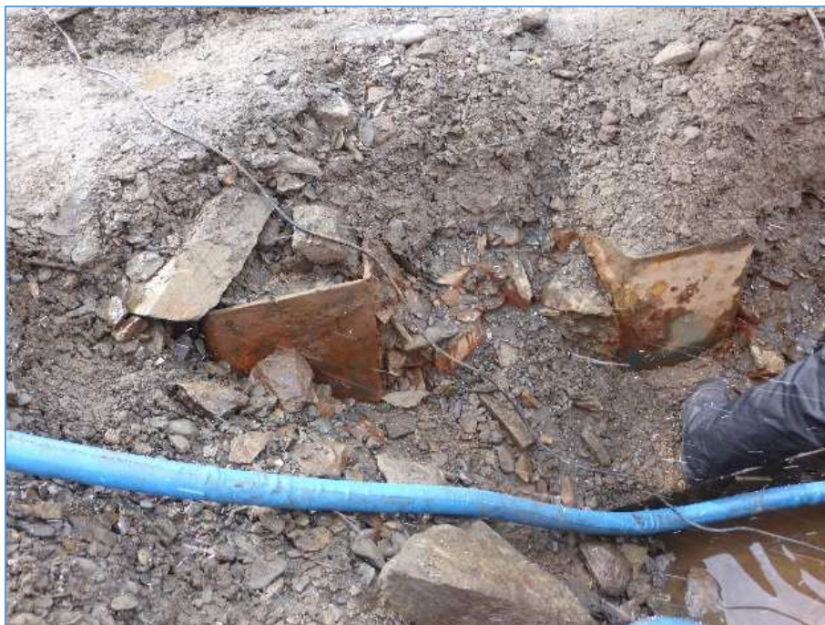
View on sheet piles to anchor wall
