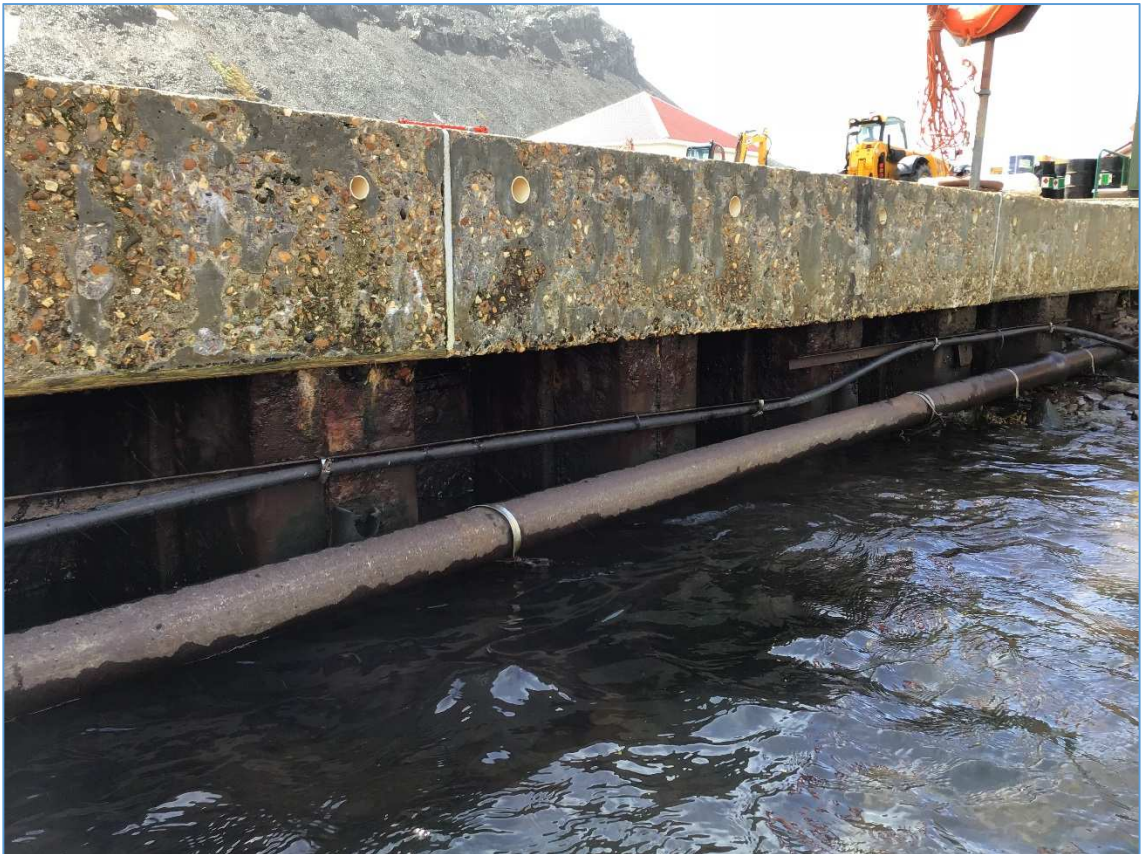
View along east section of south wall
