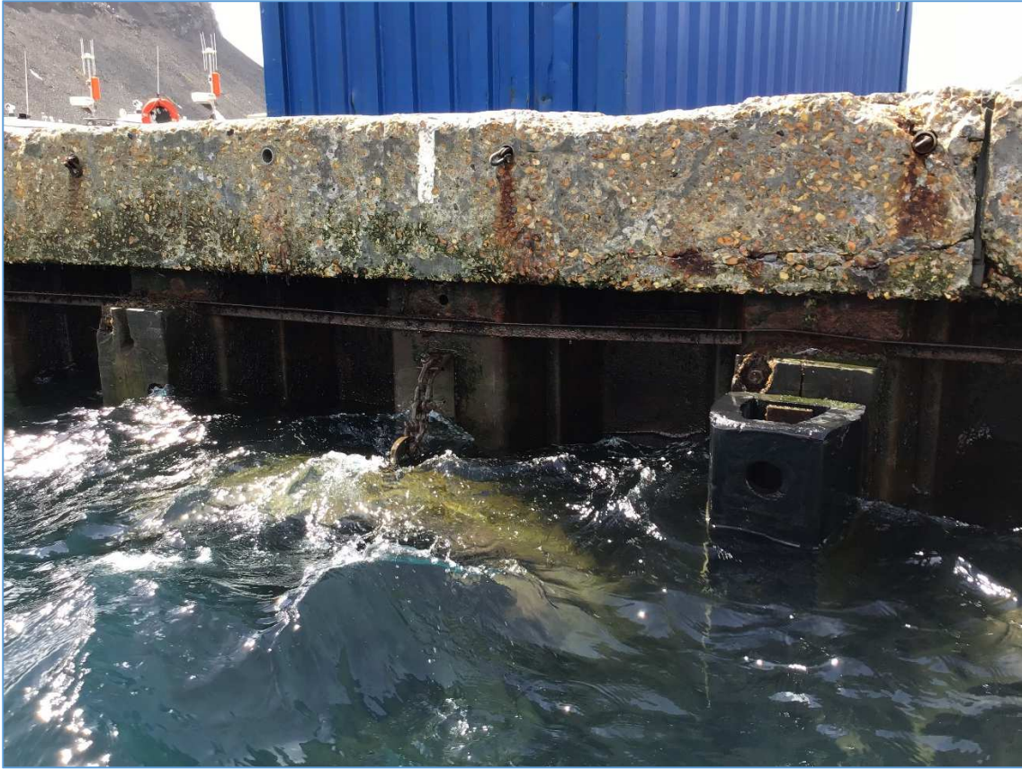
View on central section of west wall
