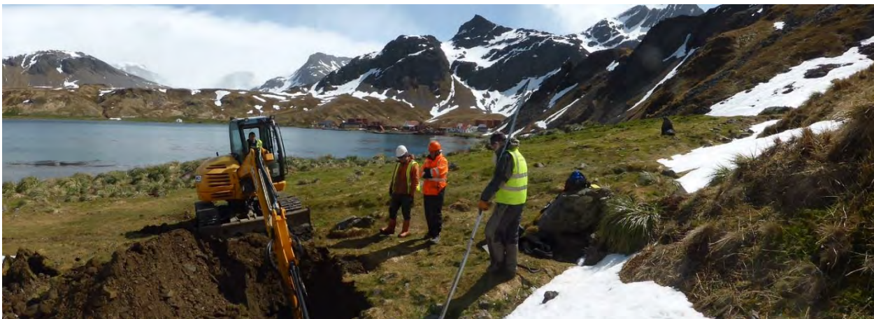
Figure 6 – Quarry 1, Trial pit 1 looking west.
