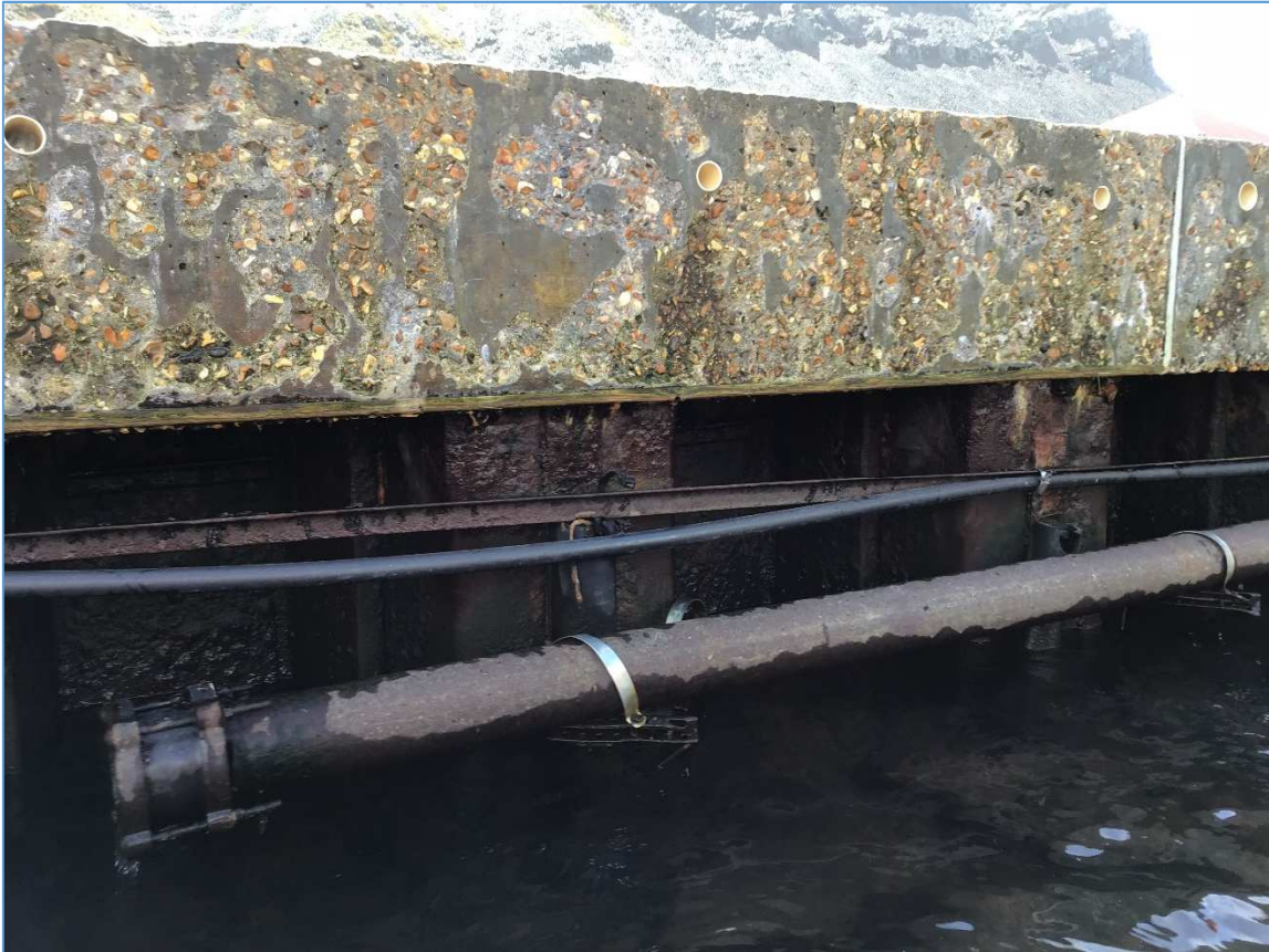
Close up view on east section of south wall
