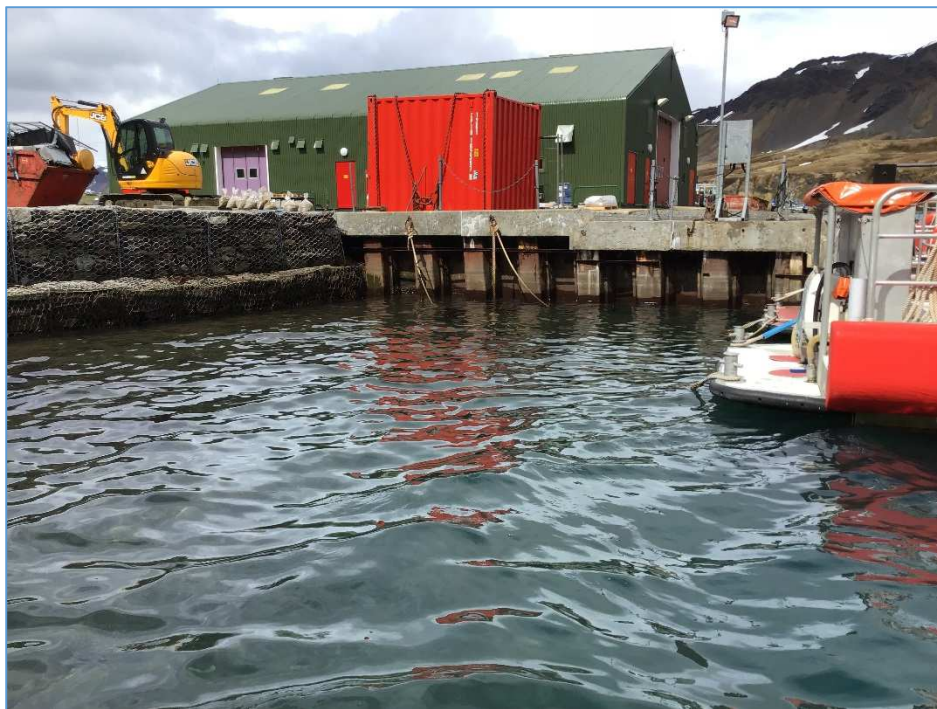
View along east section of north sheet pile wall
