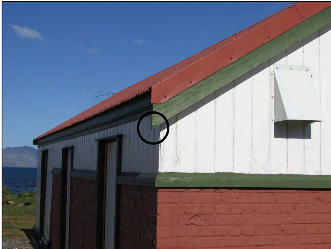
Figure 4-12; Indicated measure point on the coal shed.
