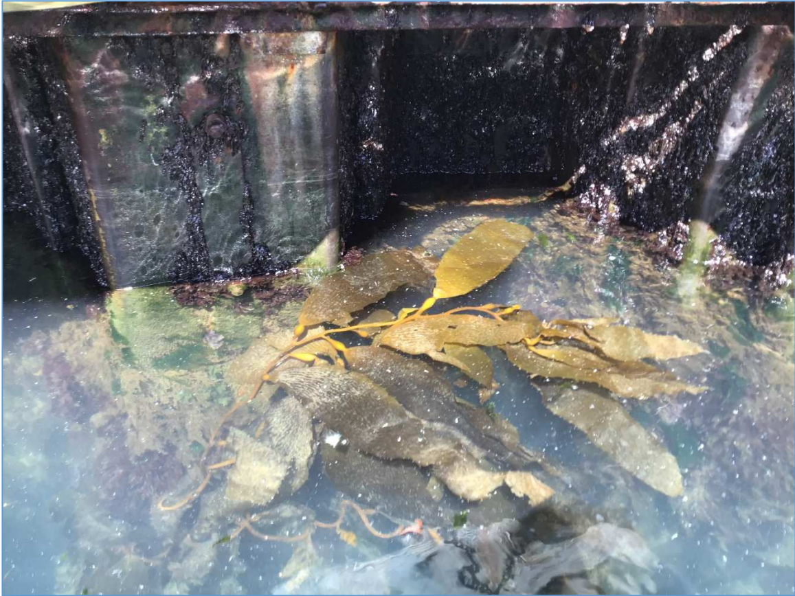
Typical view on sheet piles
