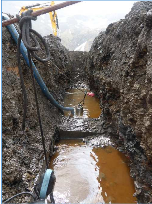
View along trial pit
