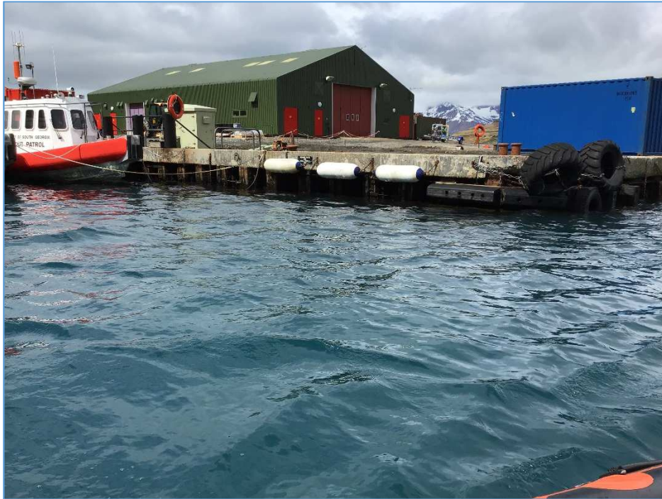
View along central and west sections of north sheet pile wall
