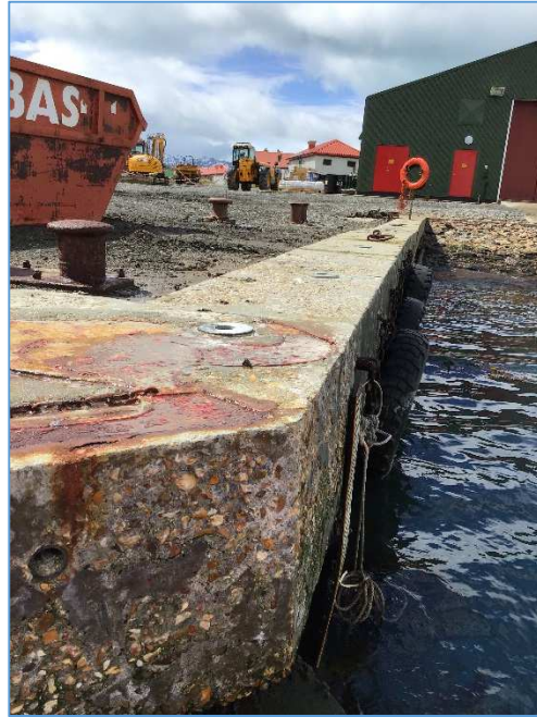
View along top of capping beam
