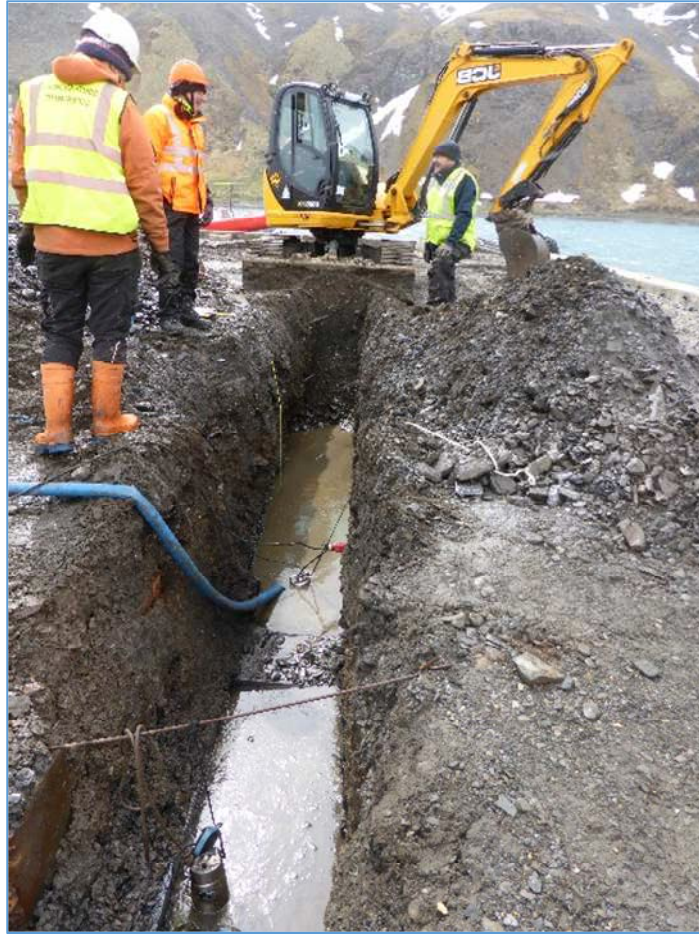
View along trial pit
