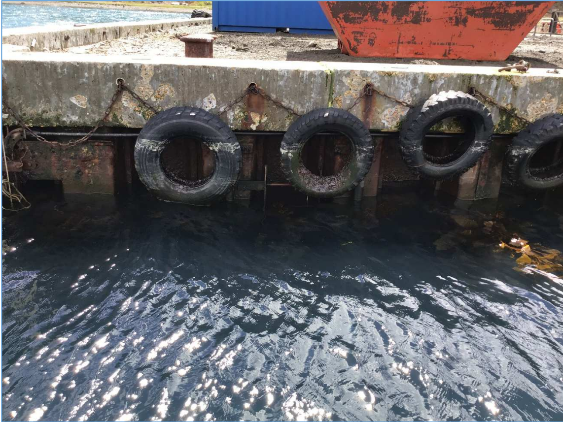
View on west end of south wall
