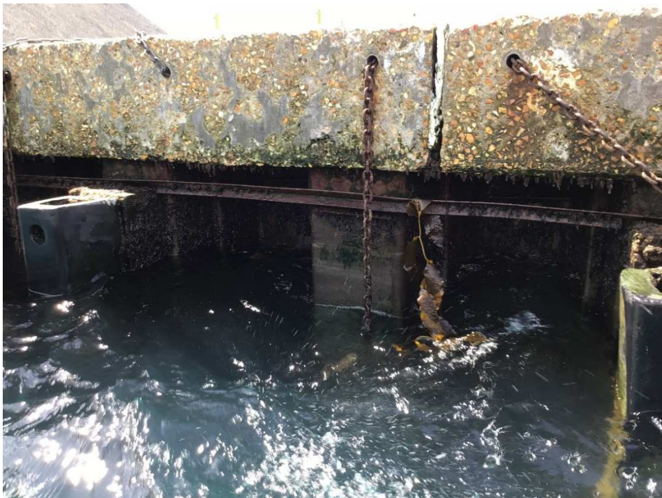
View on south section of west wall
