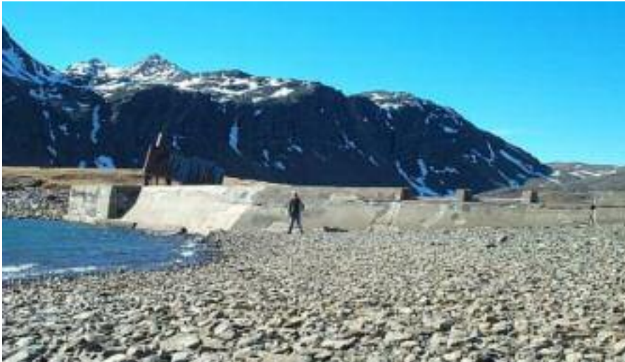
Photo of upstream face of Gull Lake dam showing water level
