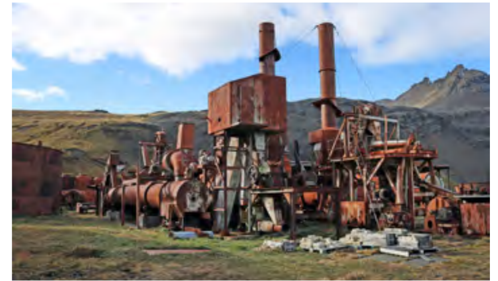
The chimneys of the Guano Factory are secured with ties
