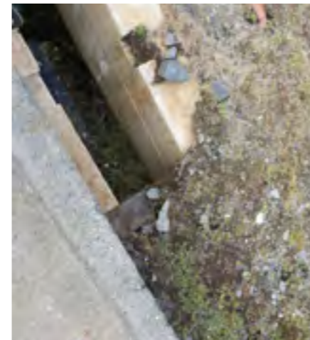
Exposed culvert near the Separator House
