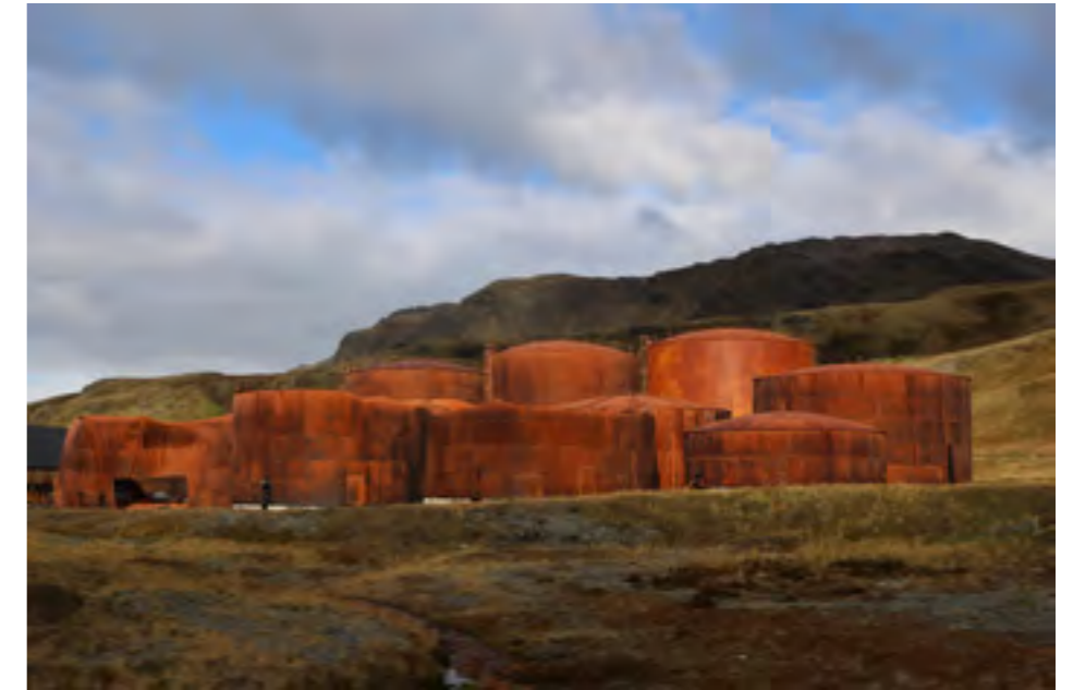
South-west storage tanks
