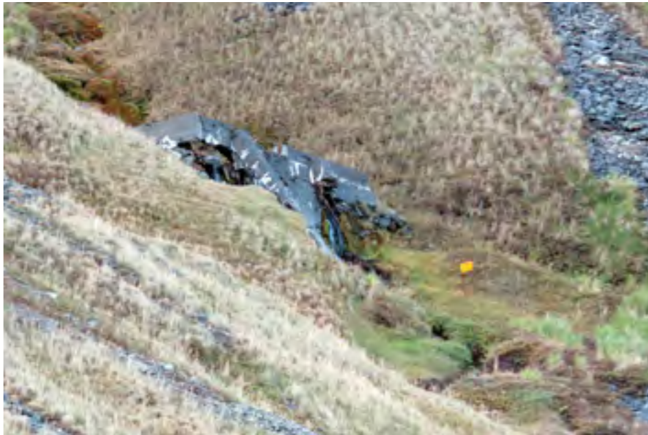
Remains of dam above KEP
