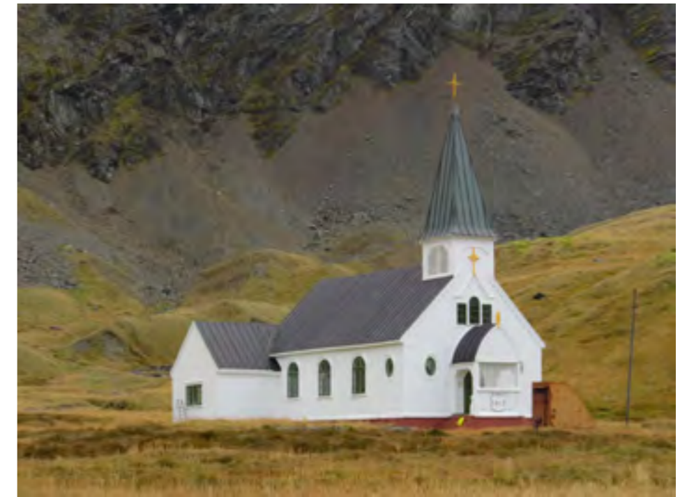
The Church was ordered as prefabricated parts from Norway and contains typical Norwegian details.
