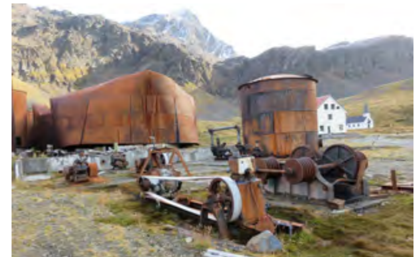
Winch House plant with Pump House plant behind. The traction winch in the foreground was originally on an early steam whale catcher and was converted for use on the slipway
