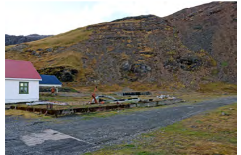
Base of the Foremen's Barracks with the machinery of the Bakery and the upstand wall of the Cold Store visible beyond
