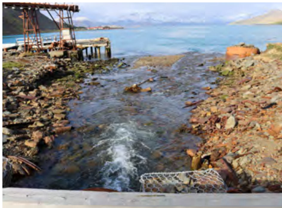
The eroding shoreline is revealing the industrial detritus used to reclaim land for the station
