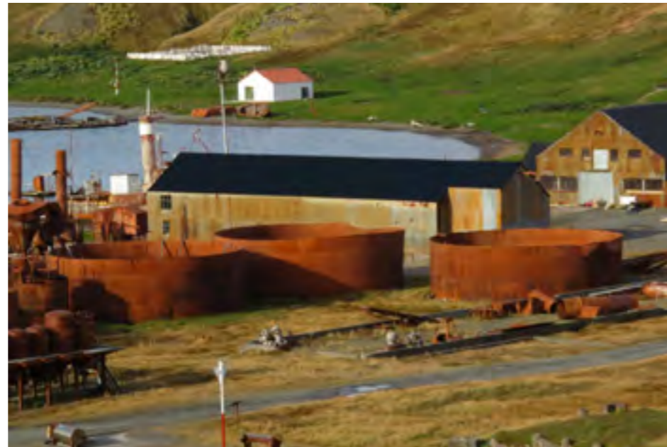
Three of the storage tanks adjacent to the factory
