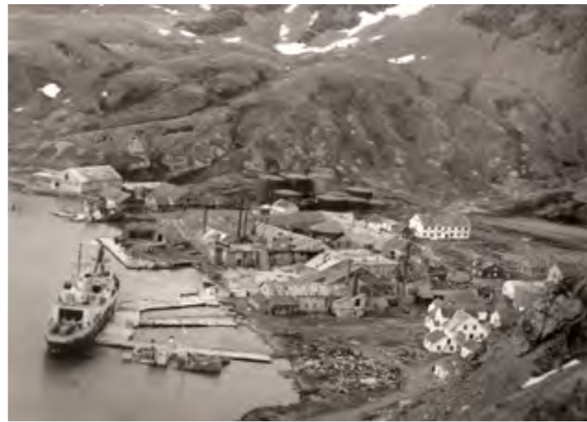
Grytviken viewed from the north in 1989. The foremen's barracks and the barracks and bath house north-west of Russebrakka had already disappeared whilst other buildings were in a poor condition. Albatros and Dias had sunk at their moorings. Reproduced courtesy of the South Georgia Museum
