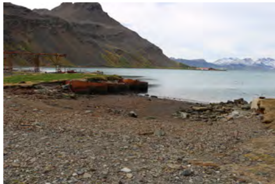
Remains of the catcher slipway
