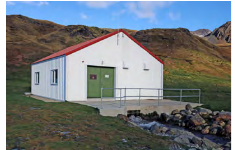
Hydro-electric Power Station
