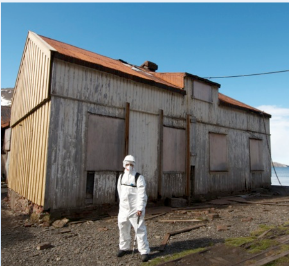
The Stromness Villa during repairs
